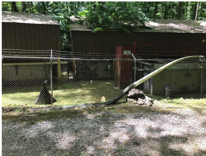
Influent PVC line is fastened to the top of the fence and should be properly buried.
