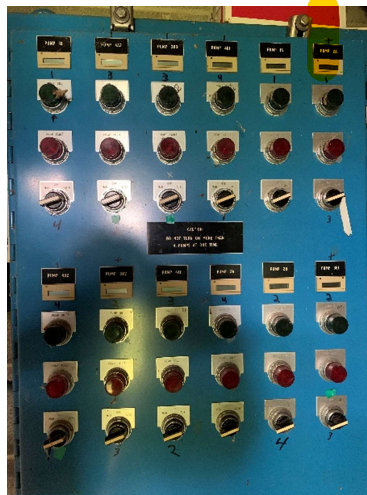
Irrigation Pump Stations Control Panel
