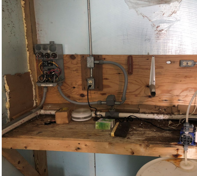
Exposed Wiring and Foamboard Being Used for Insulation
