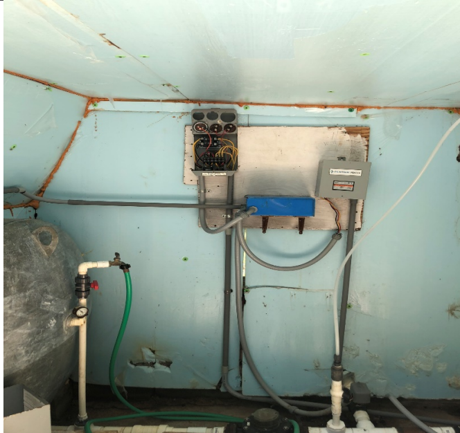
Exposed Electrical Wiring and PVC Piping That Needs to Be Converted to Steel
