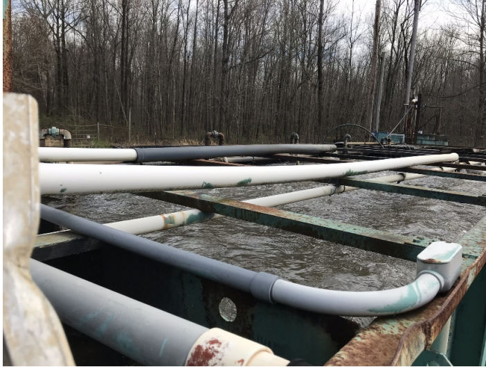
PVC lines need to be replaced
