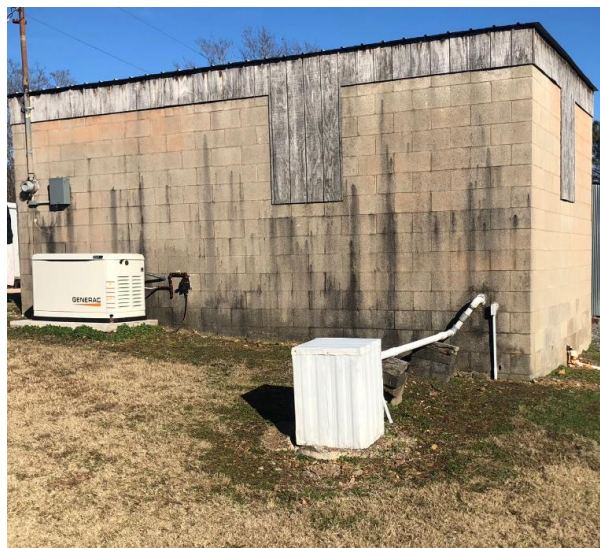
Wellhead with Exposed Wiring
