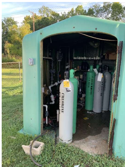
Gaseous Chlorine Storage
