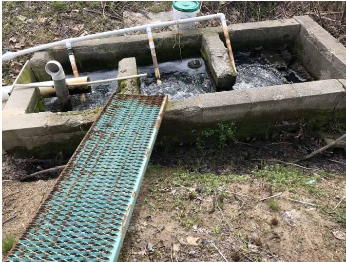
Chlorination Contact Chamber not up to code
