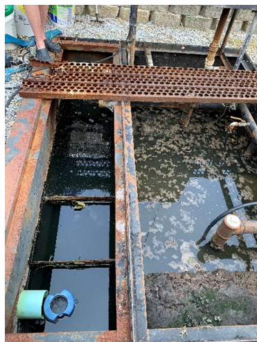
Clarifier and Contact Tank
