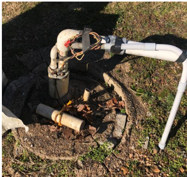
Wellhead with Exposed Wiring
