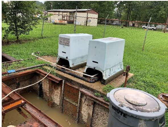
Blowers, EQ Basin, and Electrical Cables
