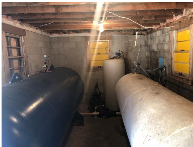
Hydro-Tank, Chlorination System, No Ceiling
