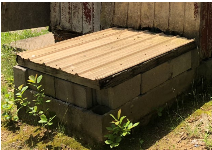
Block Structure Housing Well
