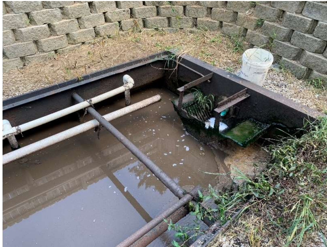
Manually Cleaned Bar Screen
