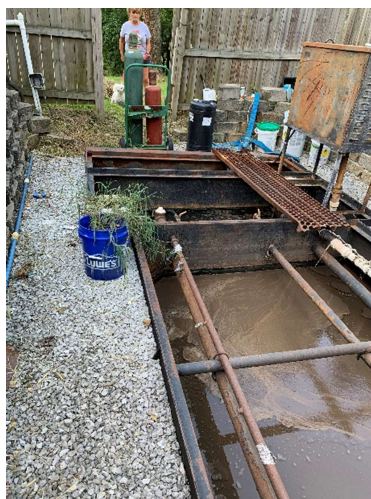
Aeration Tank, Clarifier, Contact Tank
