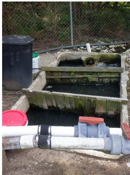
Wooden baffling in contact chamber.
