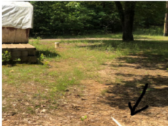
Electrical conduit servicing well pumps exposed in driveway.
