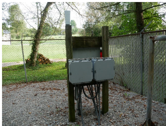
New control panels installed and electrical improvements
