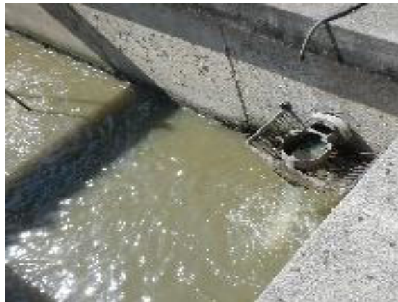
Rusted, failing bar screen
