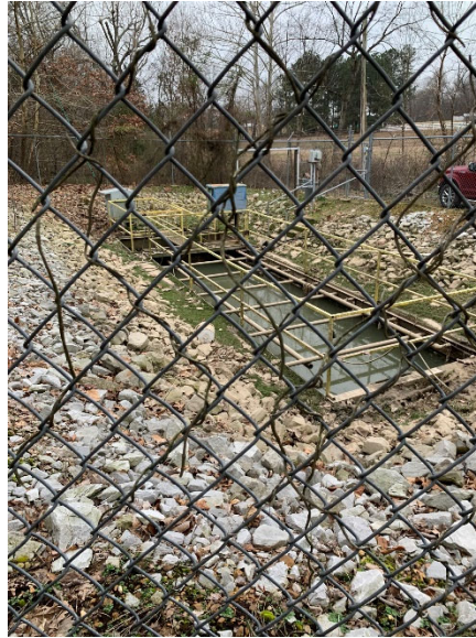
Staining notable on riprap indicating regular flooding
