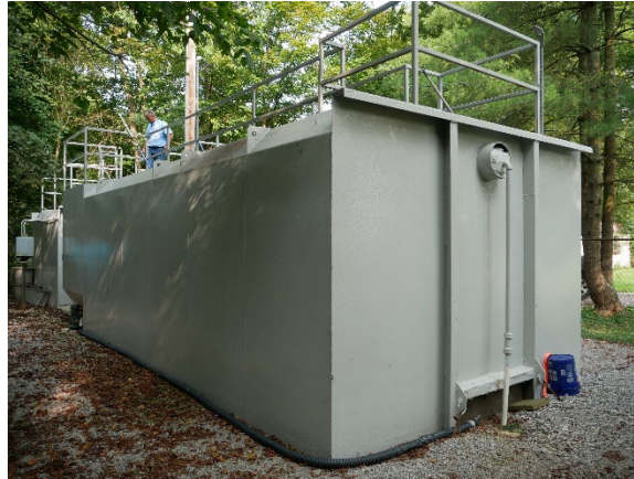
Repainted tanks, handrails, etc. new influent line
