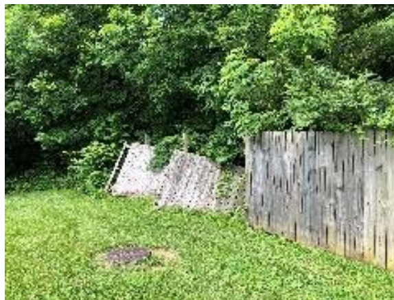
Vegetation overgrowth damaged fencing around the facility.
