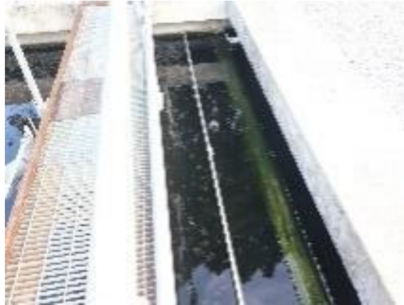
Submerged section of clarifier trough allowing passthrough of solids.
