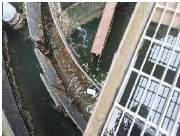
Clarifier skimmer not reaching the edge of the chamber.
