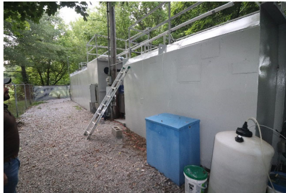
Tanks patched, sanded, and painted; debris removed
