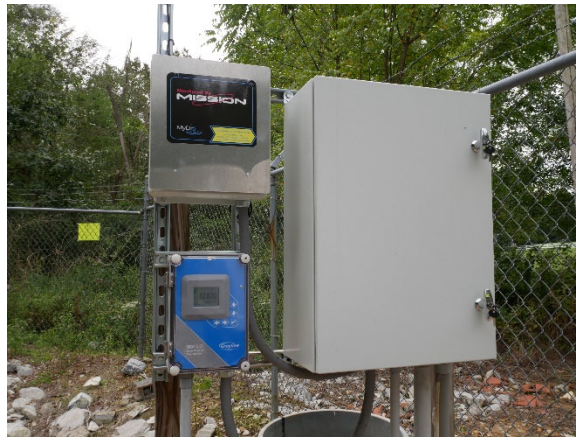
Mission remote monitoring at plant with new flow meter and control panel
