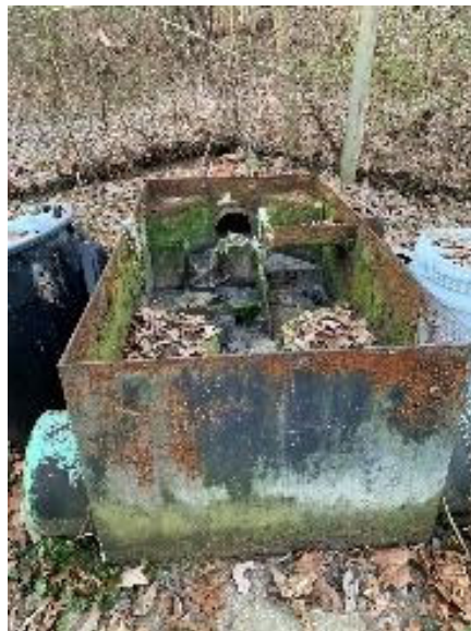
Deteriorated bar screen and splitter system almost completely rusted out.
