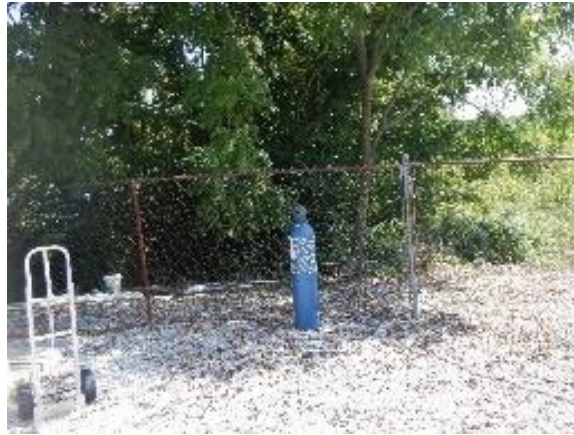
Improper chemical storage.
