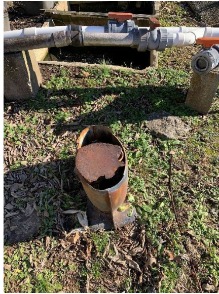
Yard piping condition and corrosion examples.
