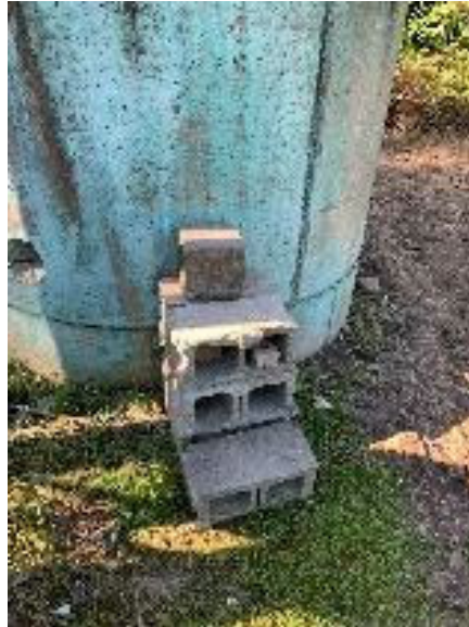
Unsafe stack of cinder block used to access the lift station.
