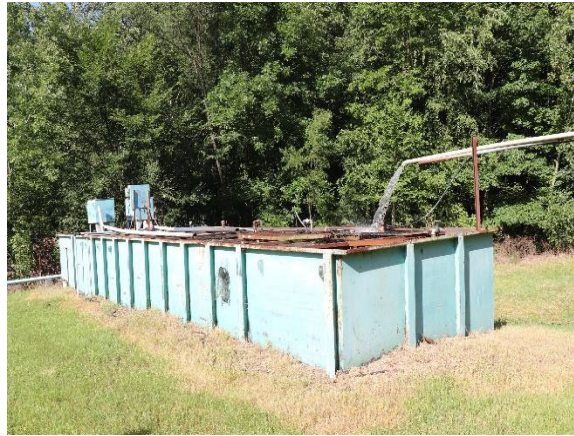
Bizarre influent line forms influent lift station, dropping waste from above into the plant.
