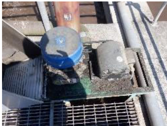
Improperly cleaned and maintained blower housings.
