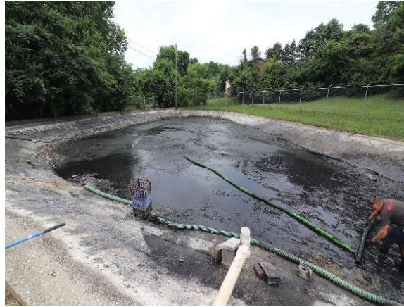
Lagoon during sludge removal.
