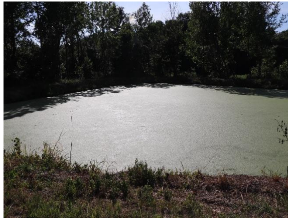
Sludge-filled with poorly maintained berms.
