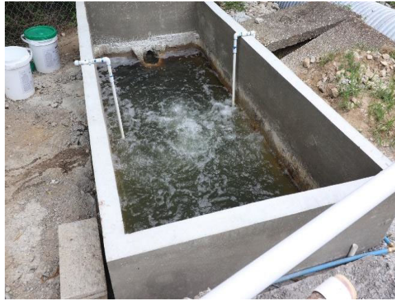
Extended walls contact chamber and post aeration repaired.
