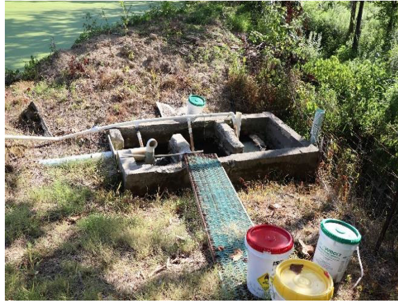
Damaged contact chamber with poorly improvised post aeration system.
