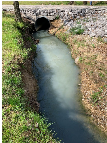
Terrible effluent quality at acquisition causing pollution
