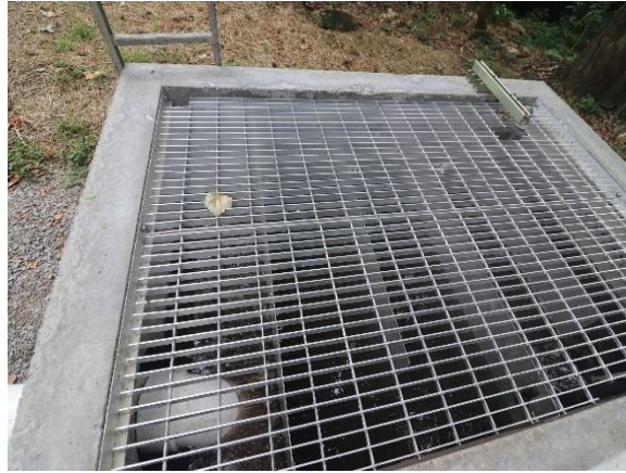
Rebuilt contact chamber.
