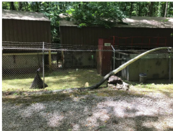
Improper influent line installation.
