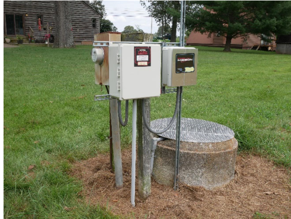
Mission remote monitoring installed at lift station
