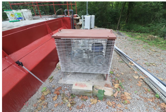
Blowers and blower housing replaced and mission remote monitoring installed
