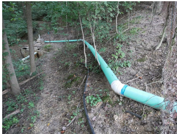
New Effluent line bypassing derelict contact chamber, outfall structure still needed
