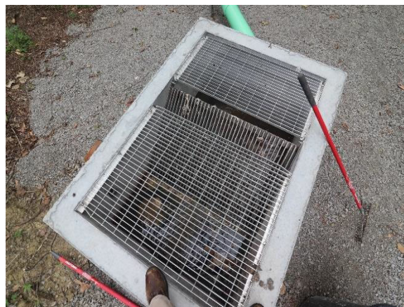
Rebuilt bar screen system. New yard piping installed
