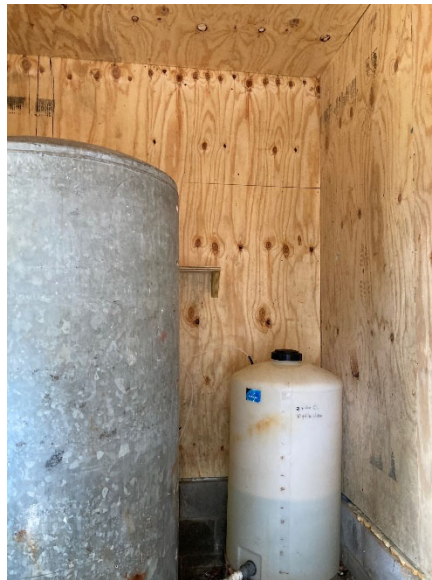
Well house interior walls replaced to improve insulation and contain wiring.
