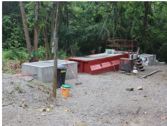
Aeration tankage patched, sanded, and repainted. Steel repaired and walkways replaced. Sludge returns replaced.
