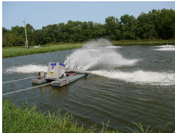
Airmaster aerator installed improving treatment
