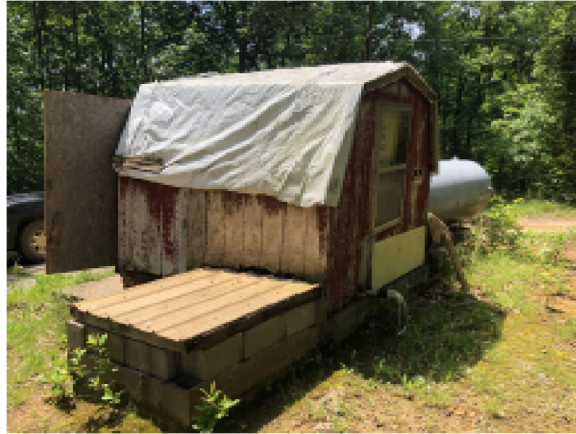
Non-compliant, improvised roof repair: a tarp nailed to roof.
