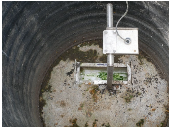
New flow meter installed
