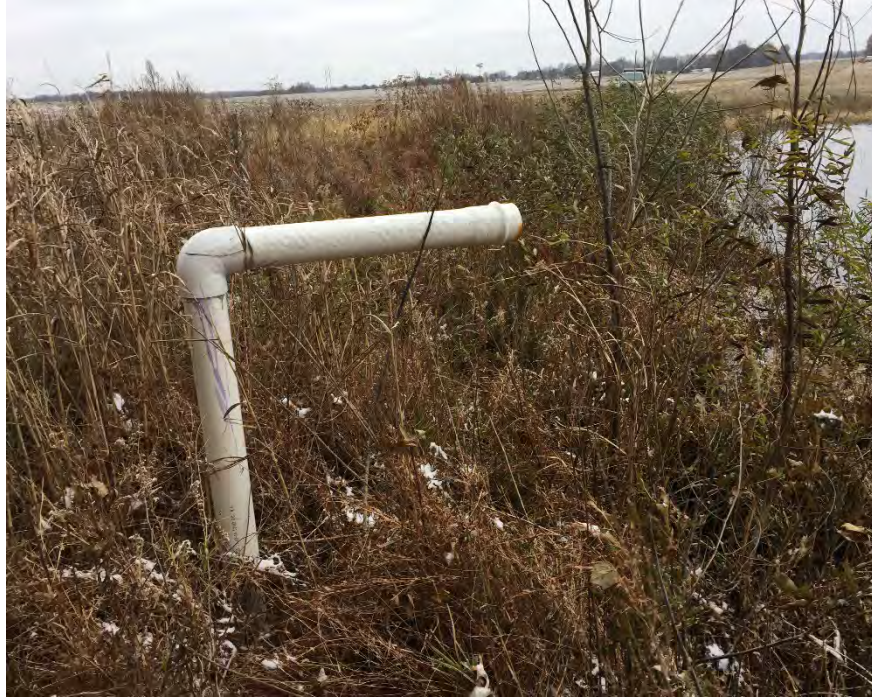
9. A water well discharge pipe feeding a pond on Parcel 38-20 as identified by the owners representative.
