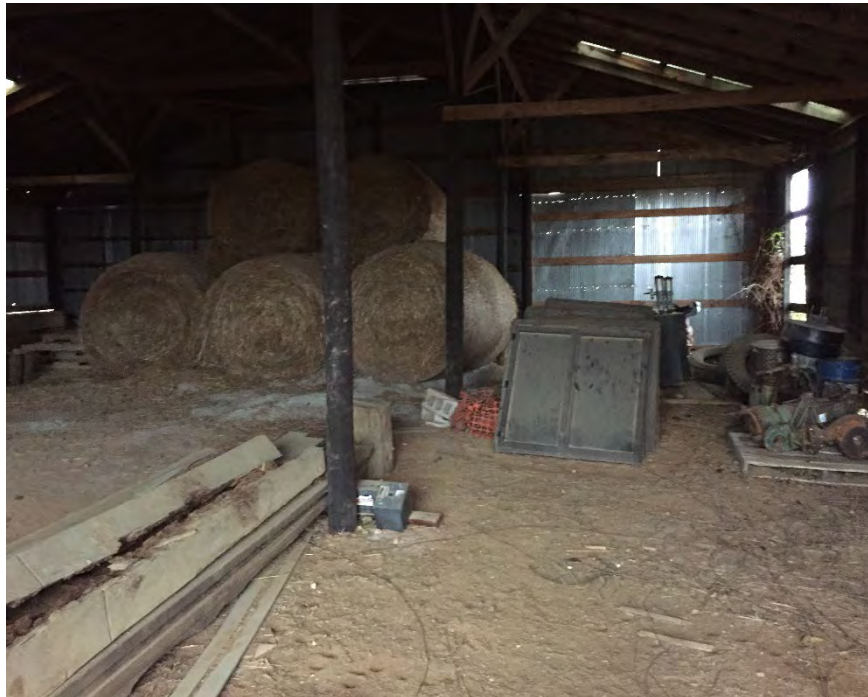
32. Inside the wood framed barn on Parcel 38-15. SMG observed hay bales, lumber, windows, farm implements and parts, a welder, pails of cut nails and two empty fuel tanks
