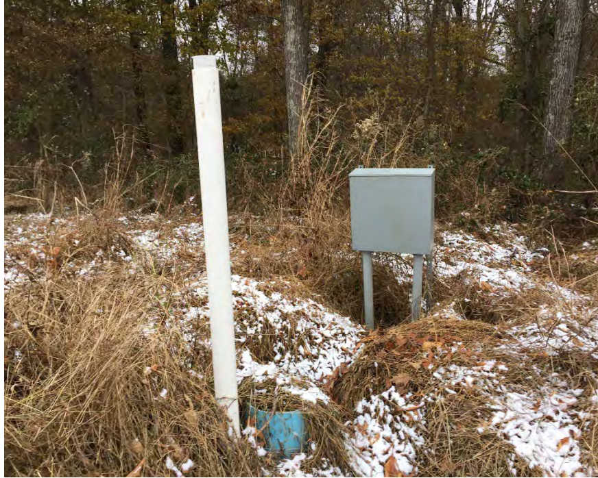
35. An electrical box and PVC pipe identified by the owners representative as being part of the electric conduit for the irrigation system on Parcels 38-15 and 38-16.
