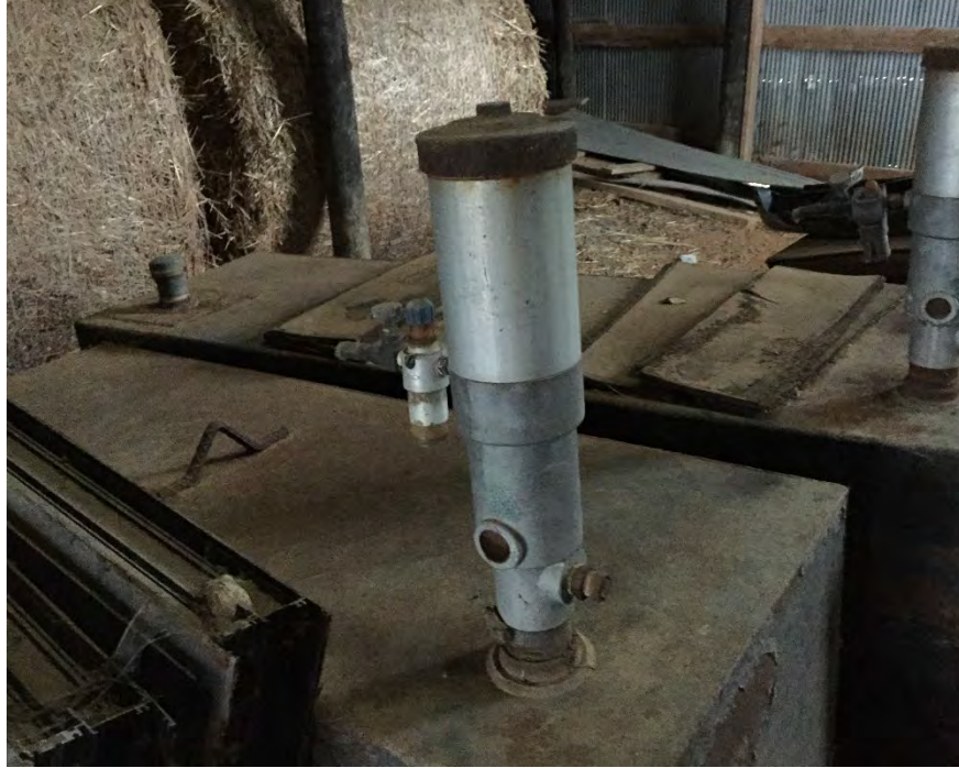
33. Two fuel tanks observed in the barn on Parcel 38-15. No odors or staining indicative of spills or releases were observed.
