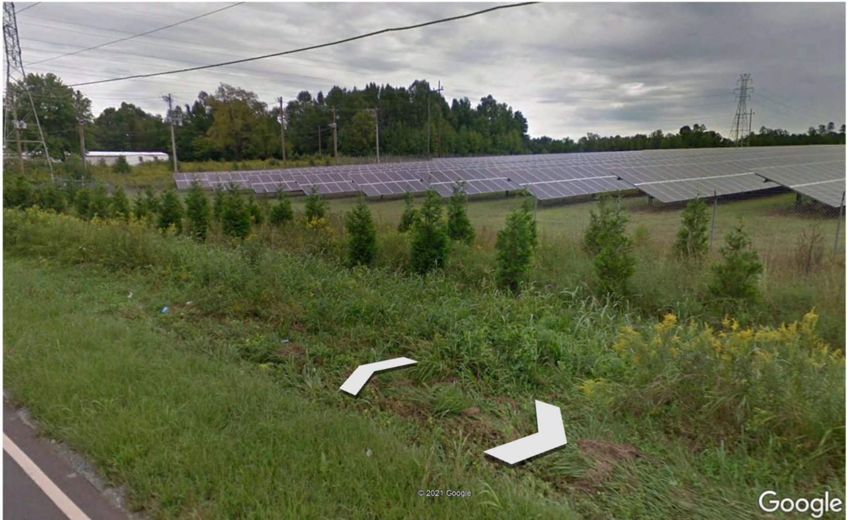
Image 4: Solar Farm in Orange County, outside of Mebane, NC. Buffer shown is an alternating row of evergreen trees approximately 6-7ft tall. Image from Google Streetview.
