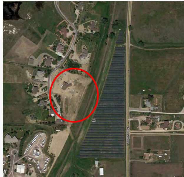
Brighton PV Solar, Adams County, CO June 2017
