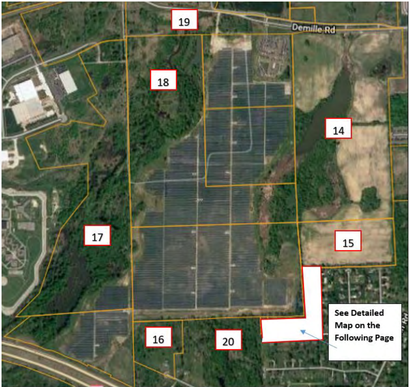
DTE's Lapeer Solar Projects - Demille Adjoining Properties
