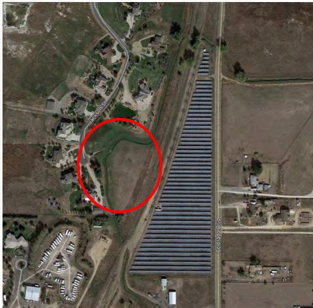
Brighton PV Solar, Adams County, CO June 2016
