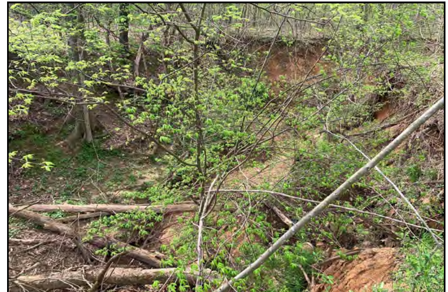
S0203, View Looking Downstream
