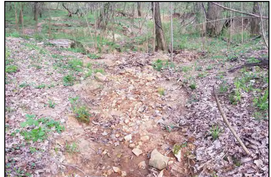
S0011, View Looking Downstream
