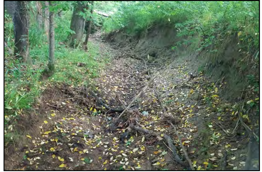
S1016, View Looking Downstream
