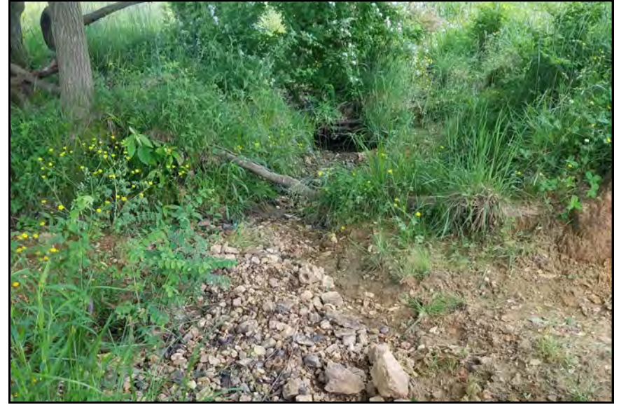
S1003, View Looking Downstream
