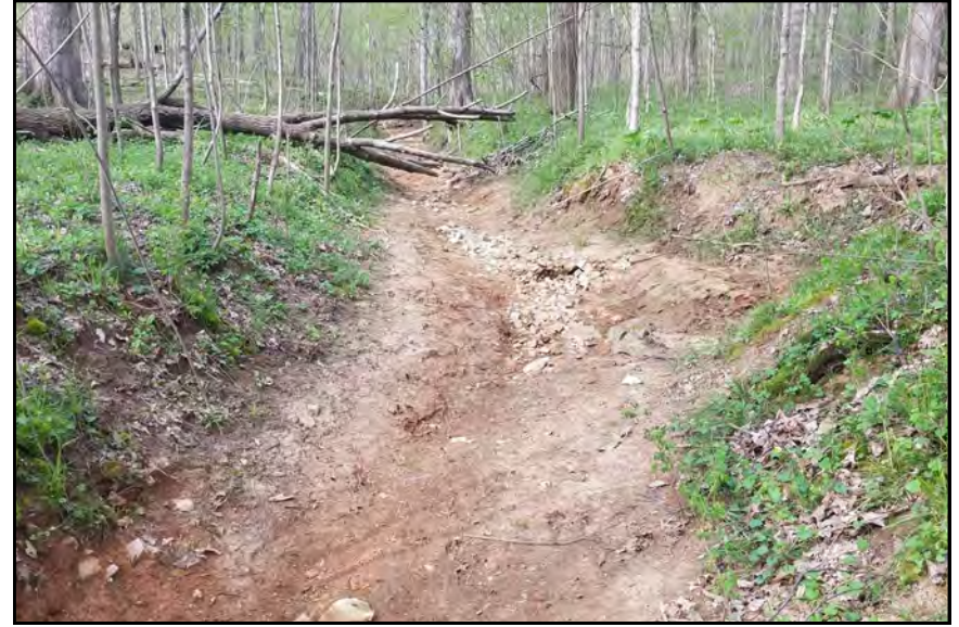
S0010, View Looking Downstream
