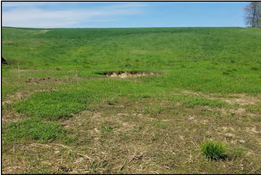
DP0009, View Looking North
