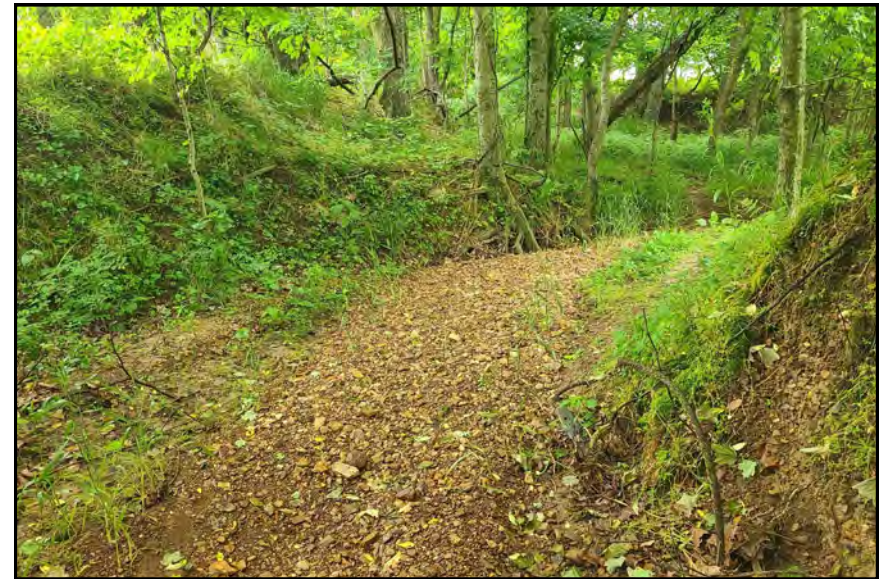
S1117, View Looking Downstream
