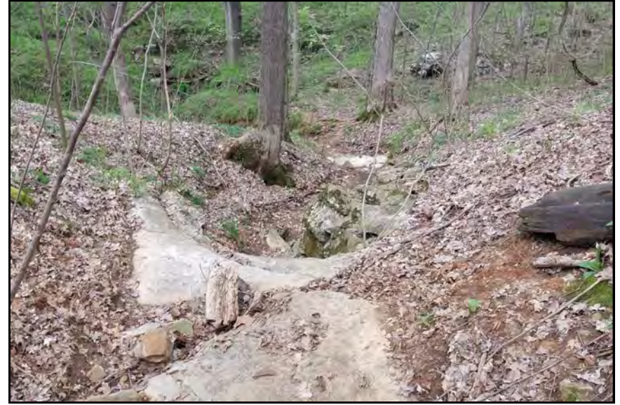
S0008, View Looking Downstream
