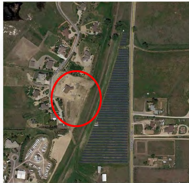
Brighton PV Solar, Adams County, CO June 2017
