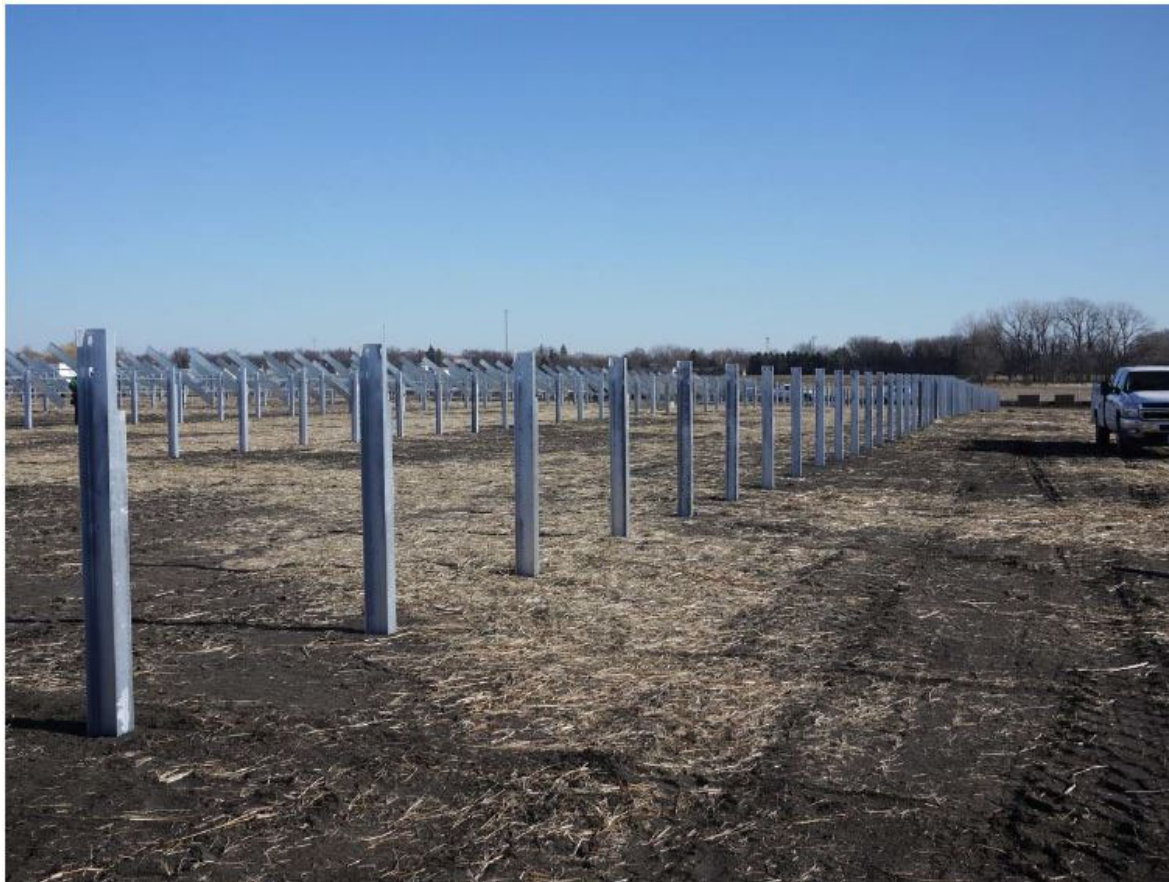
Figure 3 Standard Steel Pier Foundations
