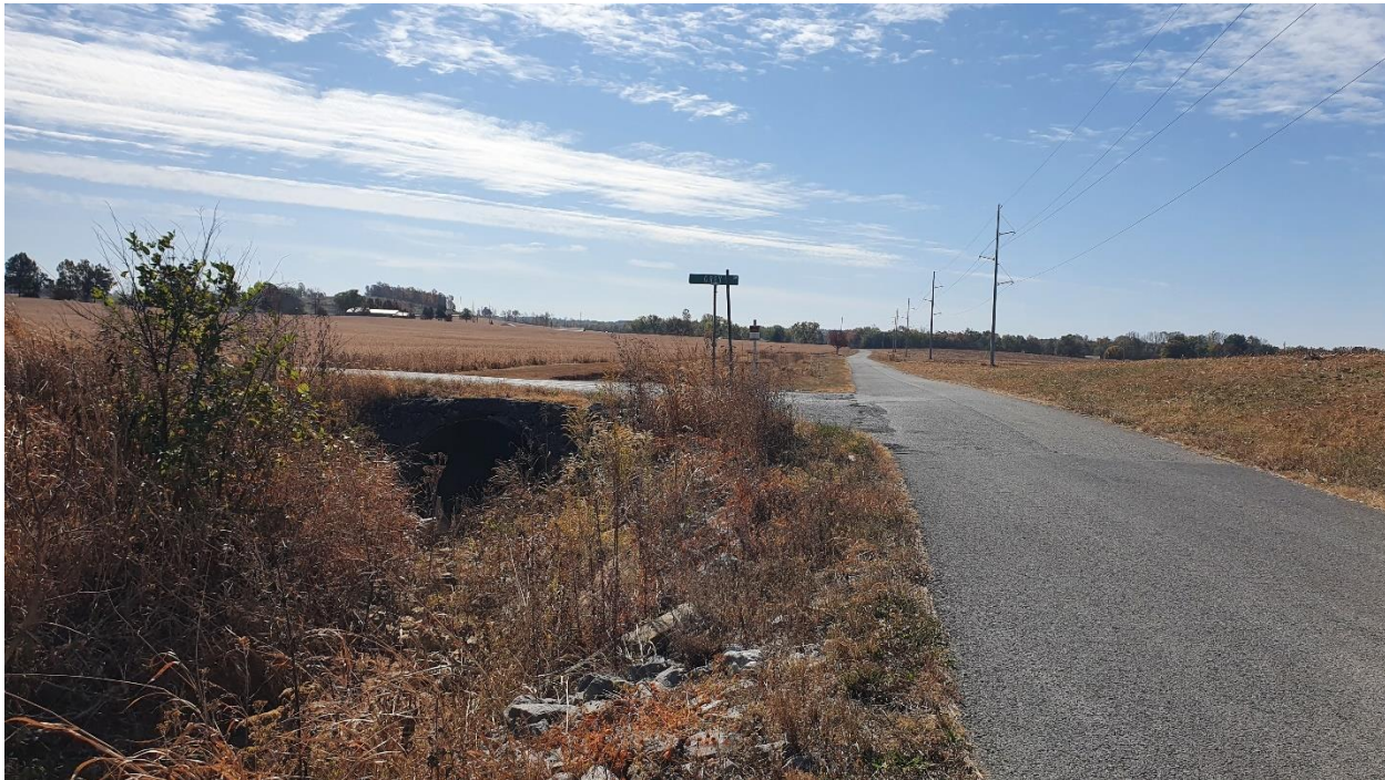
Picture (22) Culvert on Grey Rd
