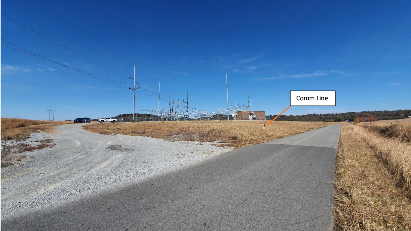
Picture (12) Location #3 Existing Substation on Goodsprings Rd
