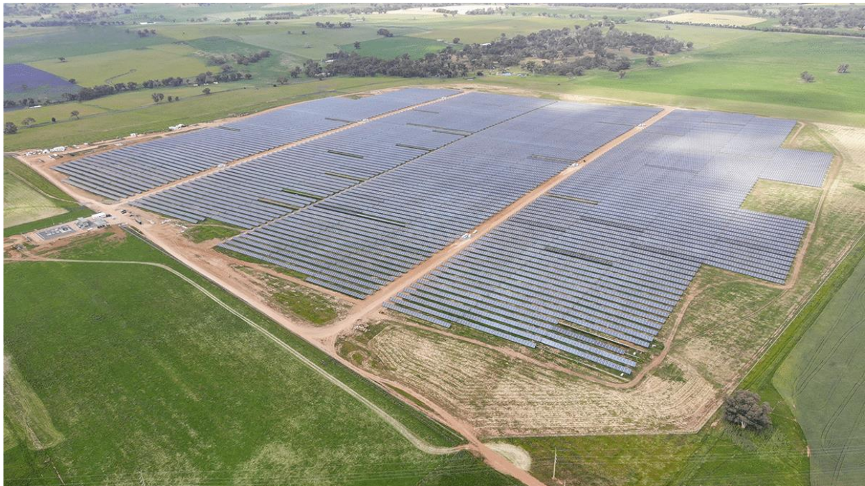
Picture (3) Solar Modules Installed on Farmland 4
