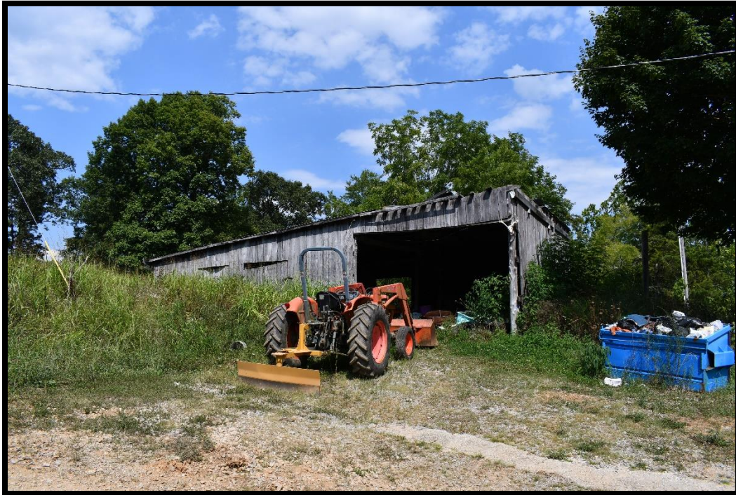
Plate 206. CA-509B, Equipment shed, west elevation, looking east.
