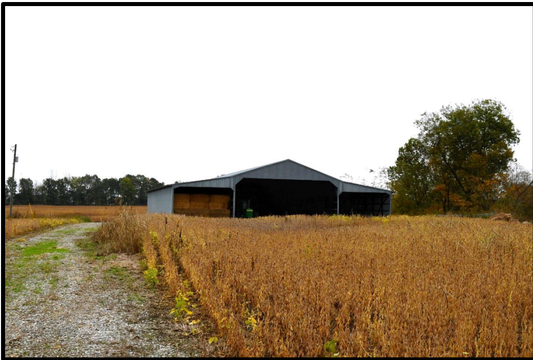
Plate 171. CA-24G, modern Midwest Three-Portal Barn, southwest elevation, looking northeast.
