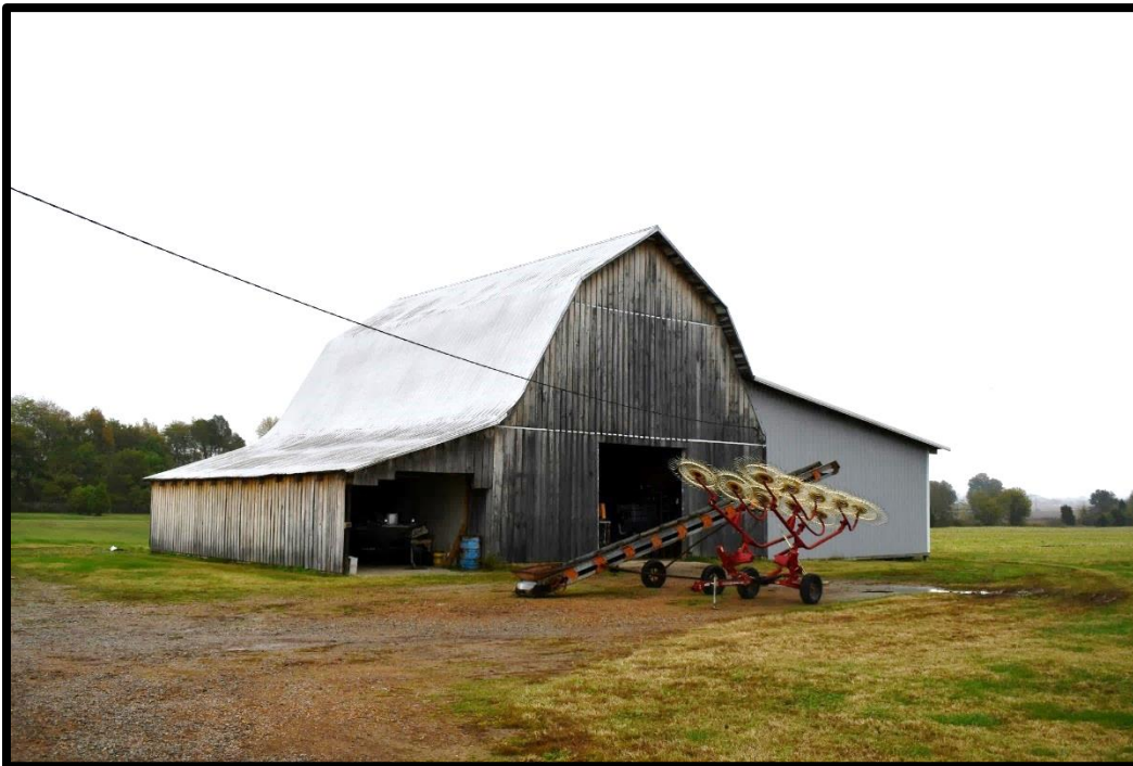
Plate 178. CA-27F, Finnish Cattle Barn, northwest and southwest (front) elevations, looking east.
