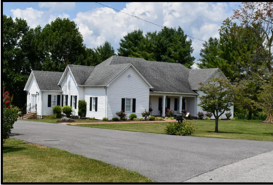
Plate 199. CA-507, House, façade and south elevation, looking northwest.
