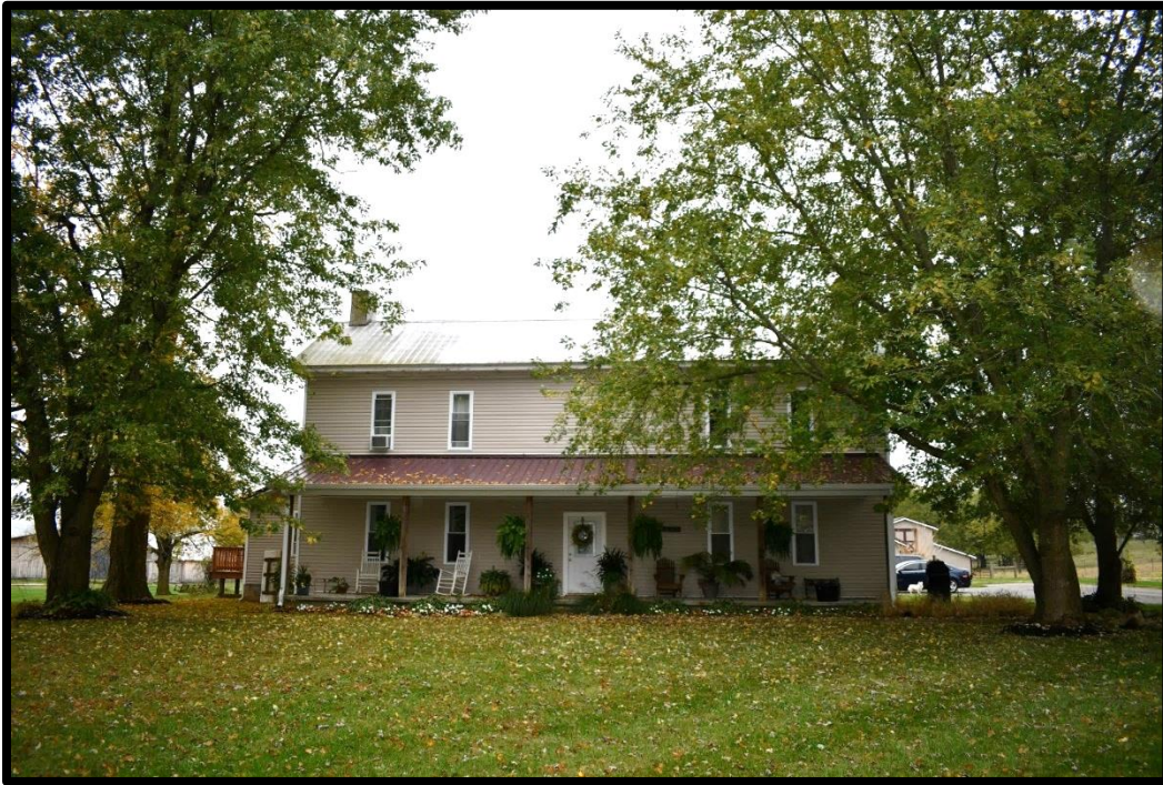
Plate 173. CA-27, I-House, looking southwest.
