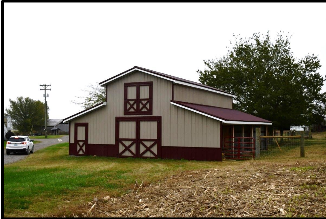
Plate 175. CA-27C, Transverse frame barn, northeast (front) and northwest elevations, looking south.
