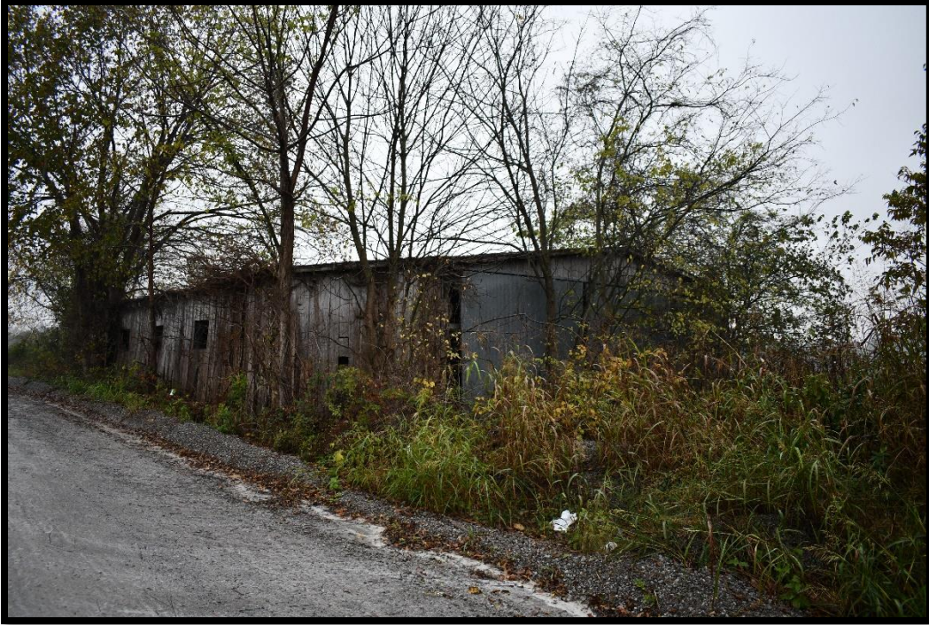
Plate 194. CA-455, Stock barn, looking northwest.
