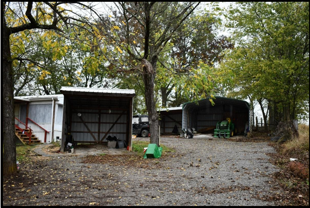
Plate 189. CA-28F, Carport, and CA-28G, carport, east elevations, looking west.
