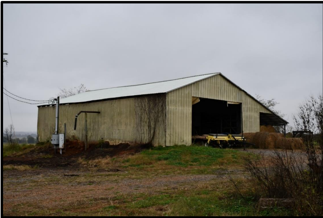
Plate 182. CA-27J, Pole barn, northeast and northwest elevations, looking south.
