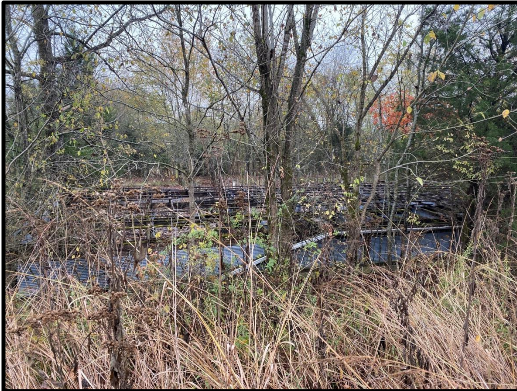
Plate 192. CA-28K, Equipment shed (ruin), looking south.
