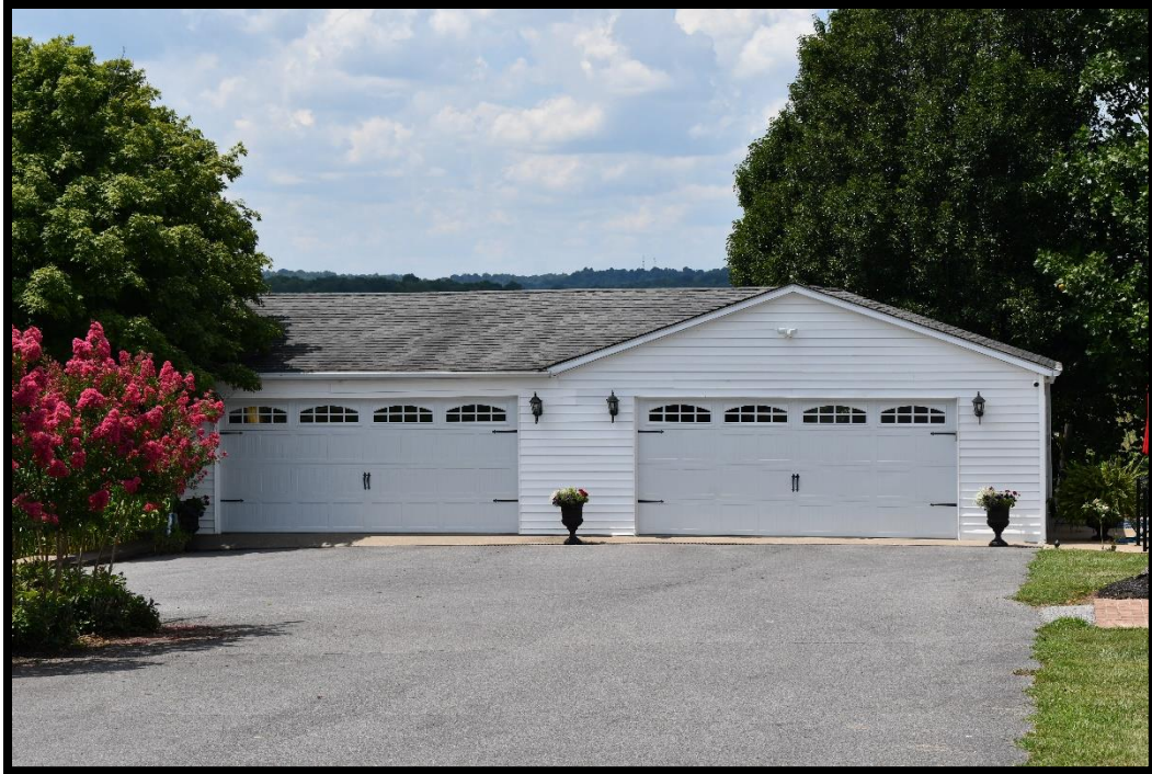
Plate 200. CA-507B, Garage, looking west.
