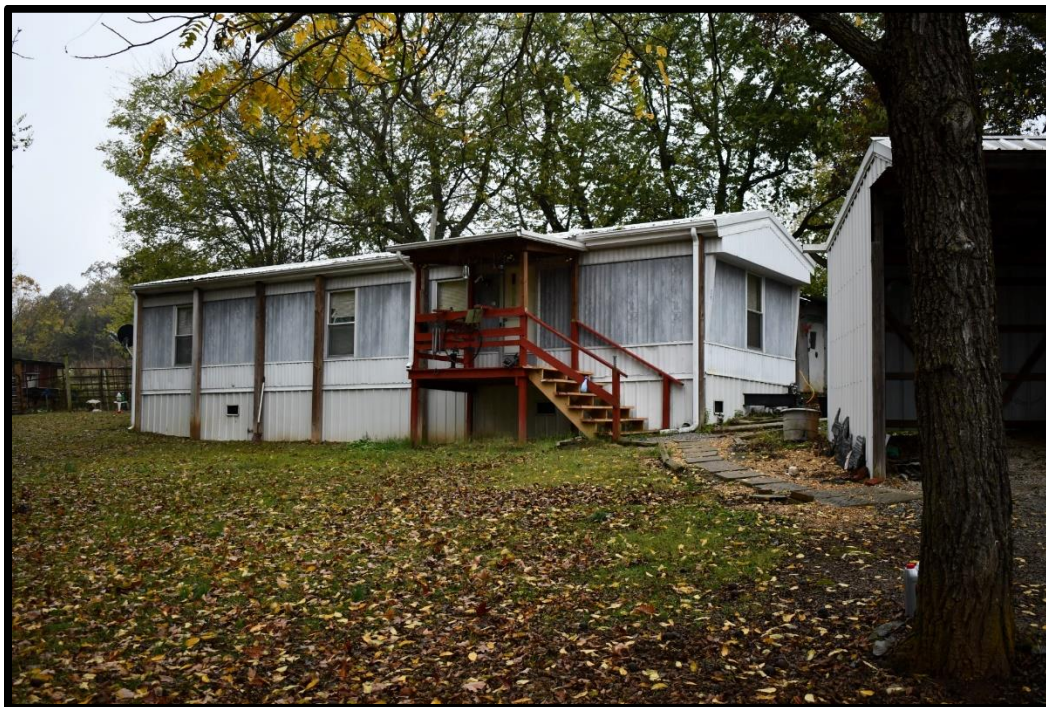
Plate 188. CA-28E, Mobile home, northeast and southeast (front) elevations, looking west.
