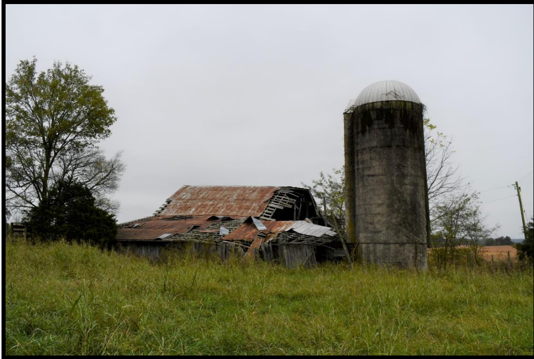
Plate 167. CA-24A, Barn, and CA-24B, silo, northwest and northeast elevations, looking south.
