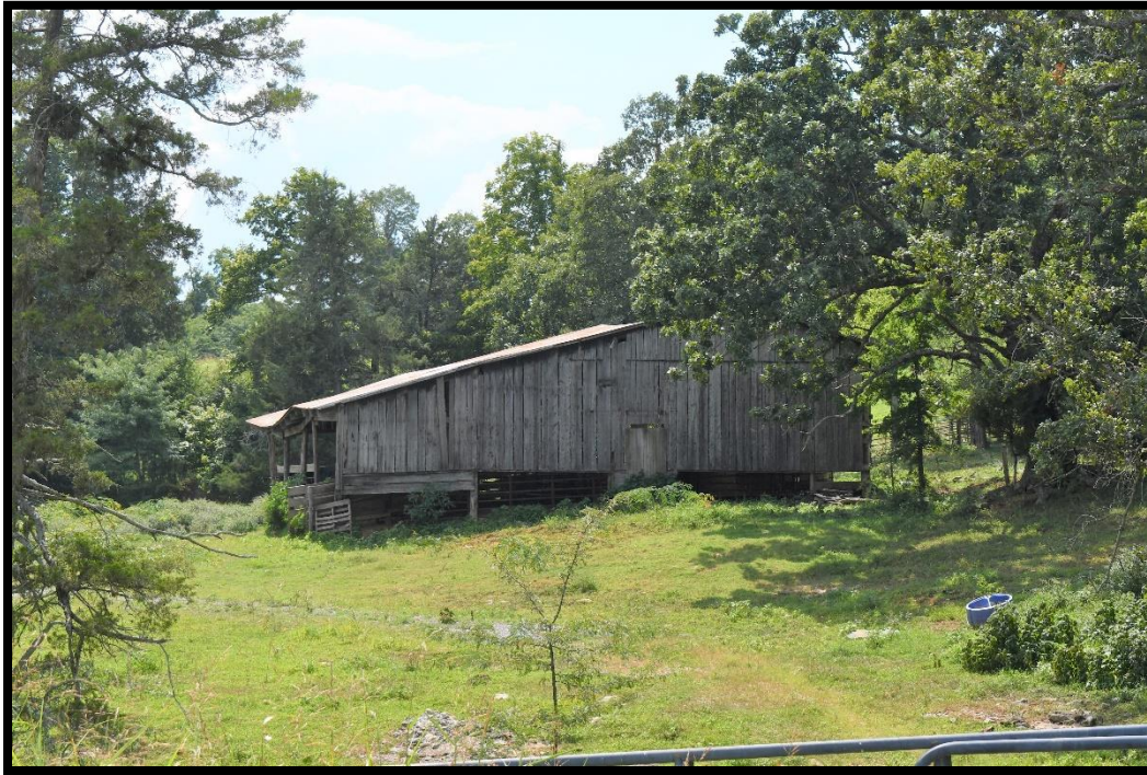
Plate 205. CA-509, Cattle barn, east elevation, looking west.
