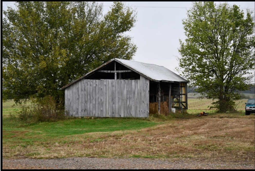
Plate 181. CA-27I, Machine shed, northwest and southwest elevations, looking east.
