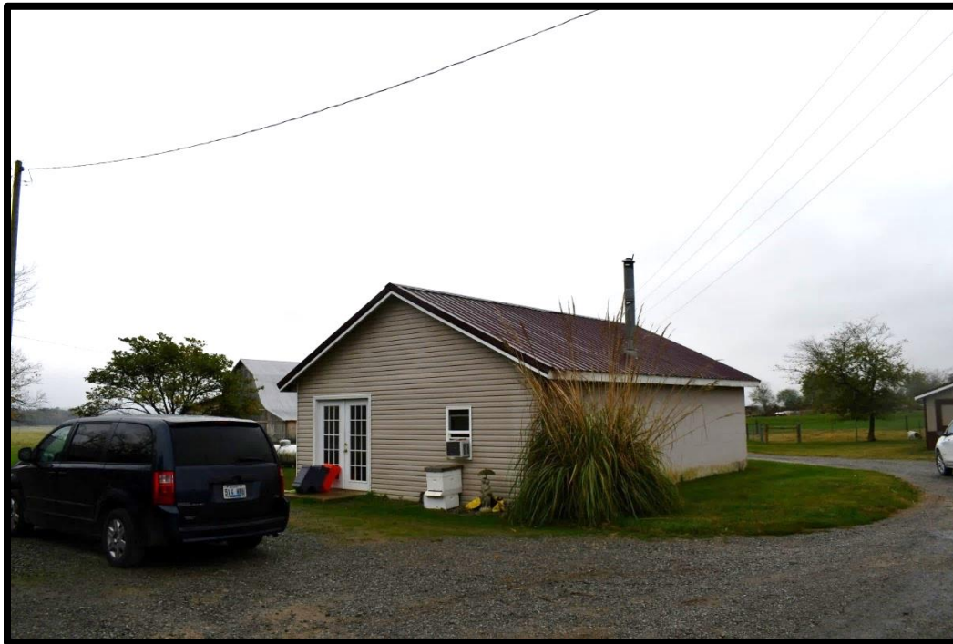
Plate 174. CA-27B, Garage, northeast (front) and northwest elevations, looking south.
