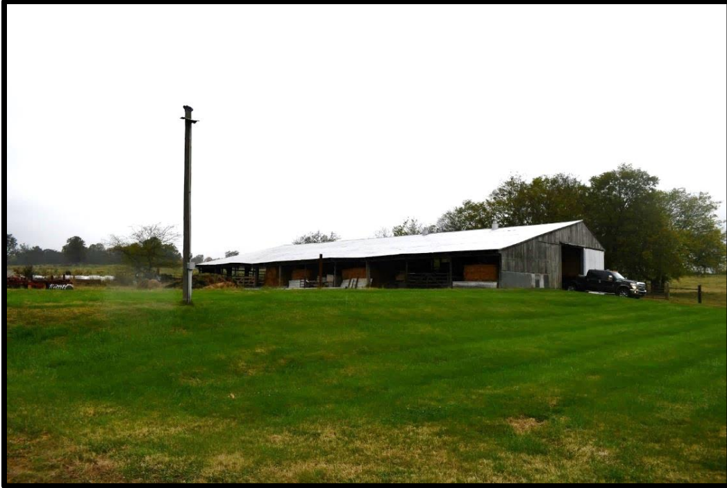
Plate 183. CA-27K, Pole barn, northeast and southeast elevations, looking west.
