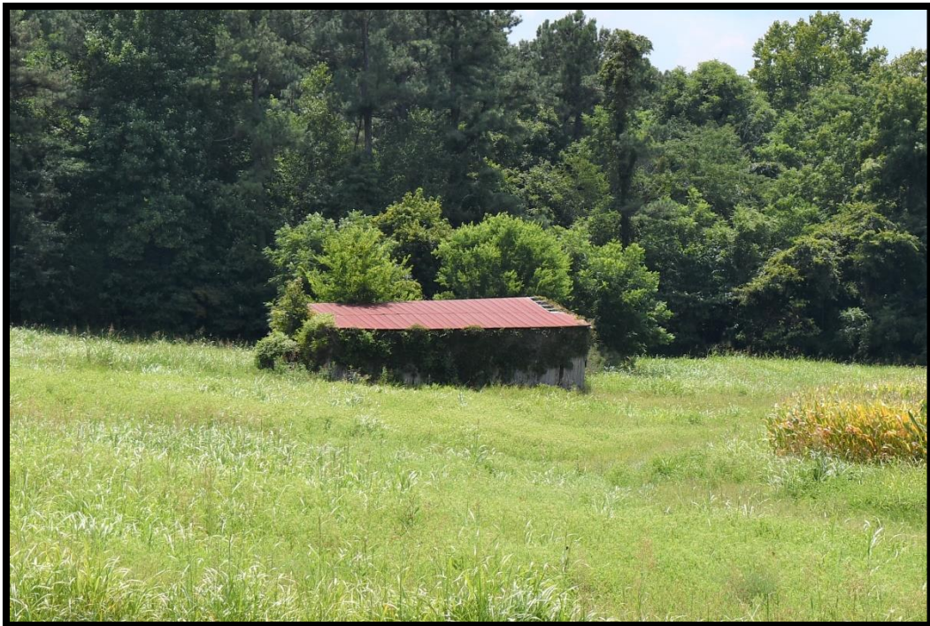
Plate 201. CA-507C, Barn, looking southwest.
