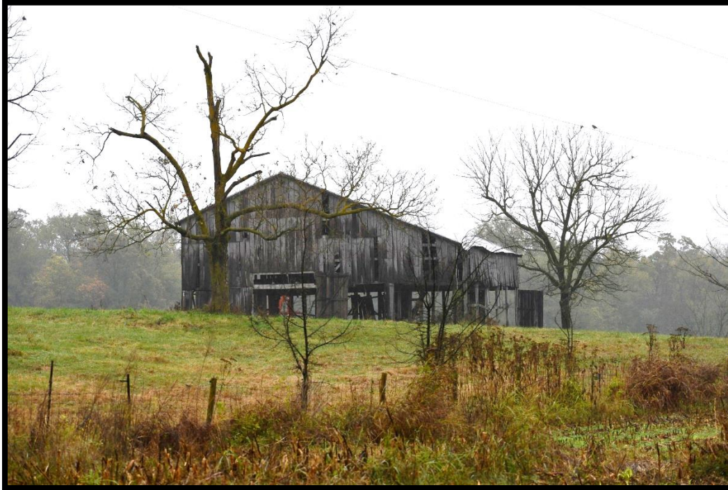
Plate 196. CA-45A, Barn, west (front) and south elevations, looking northeast.
