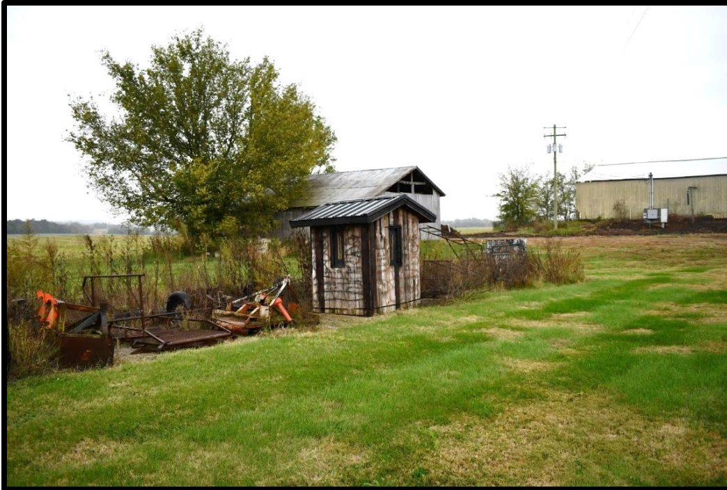
Plate 179. CA-27G, Shed, northwest and northeast elevations, looking south.
