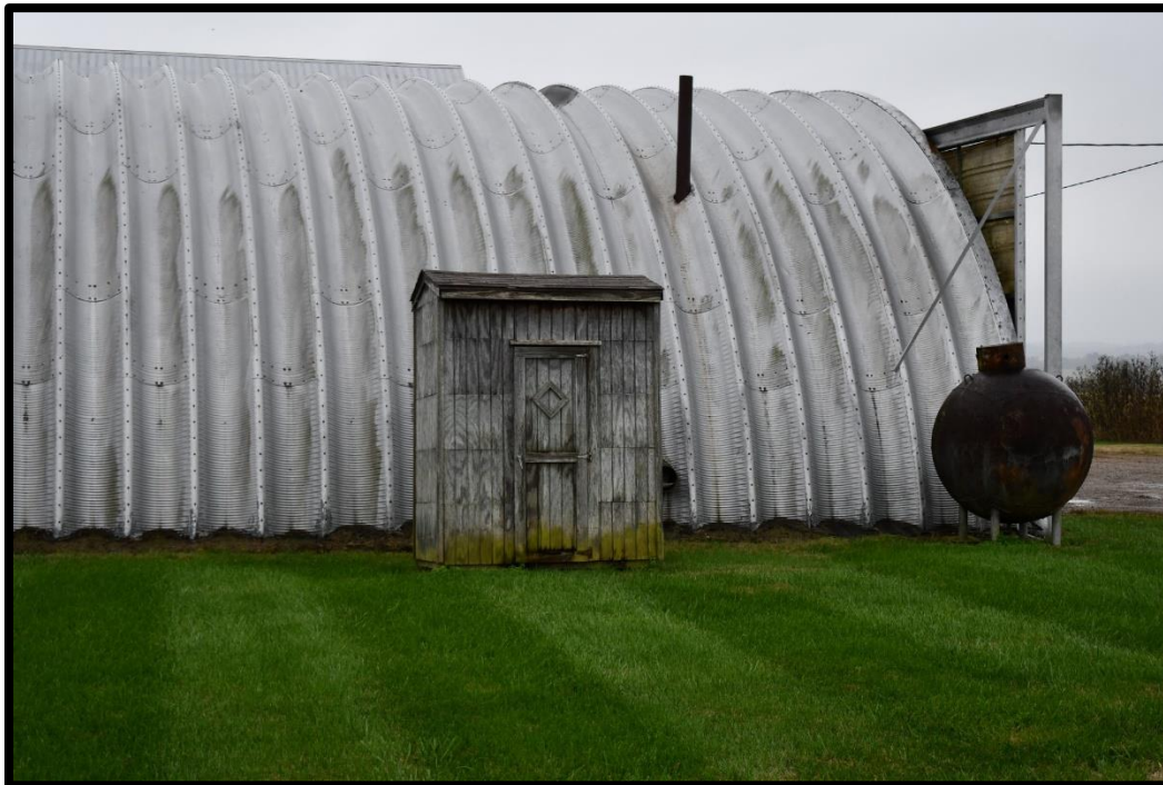
Plate 176. CA-27D, Outhouse, northwest elevation, looking southeast.
