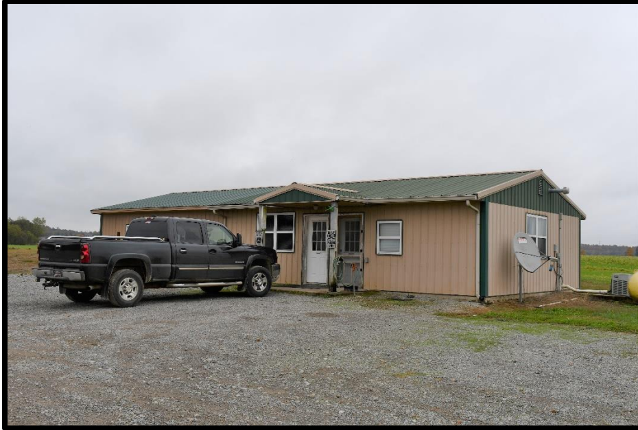
Plate 148. CA-449I, Older office, north and south elevations, looking northeast.
