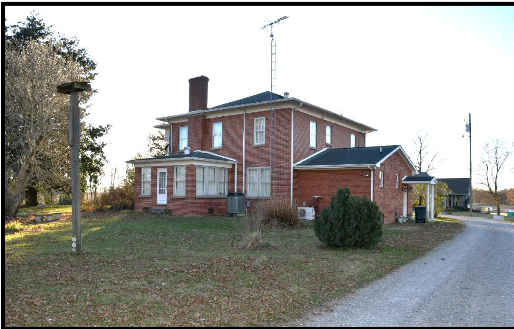
Plate 138. CA-449A, House, east and north elevations, looking southwest.
