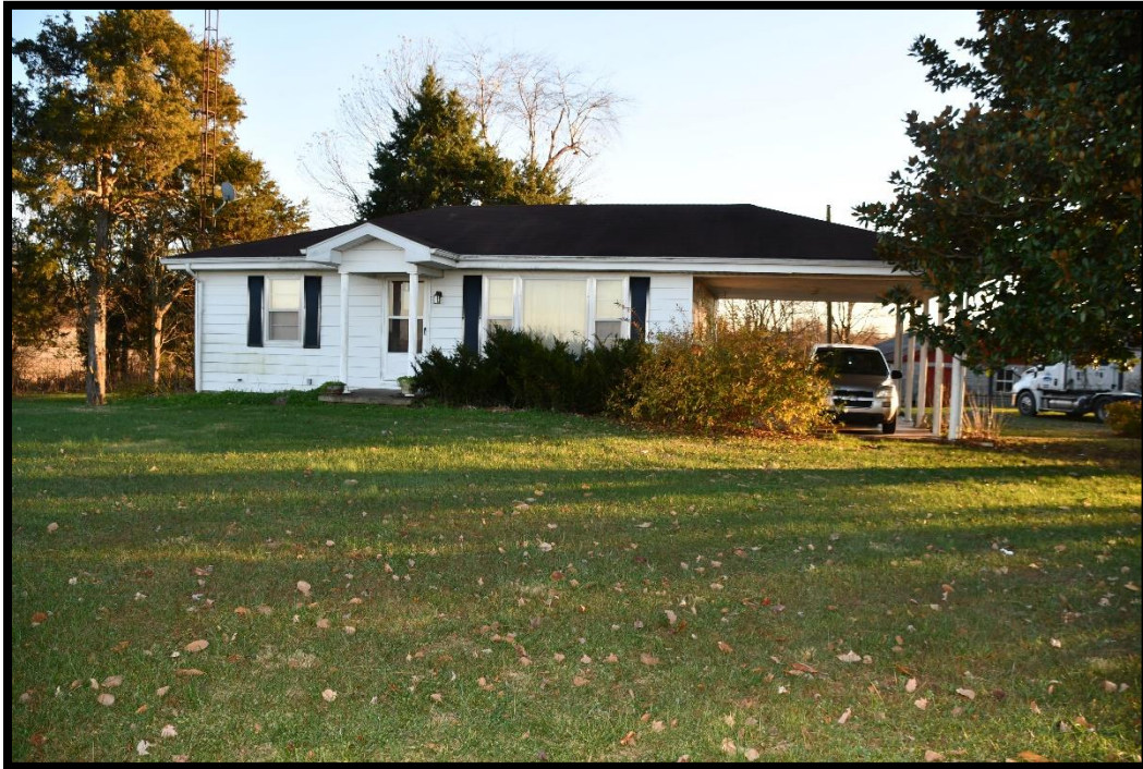
Plate 33. CA-481, House, looking south.
