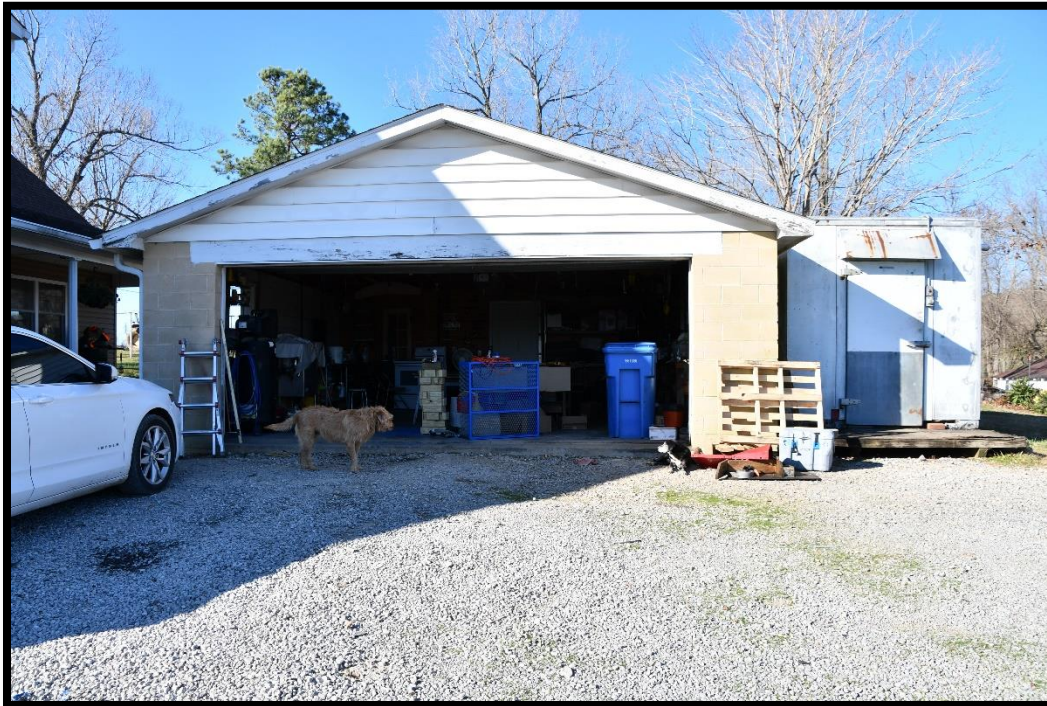
Plate 62. CA-489B, Garage, looking west.
