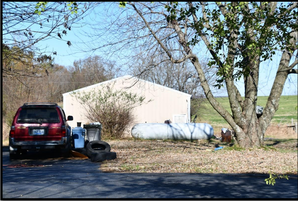
Plate 7. CA-469B, Workshop, looking NE.
