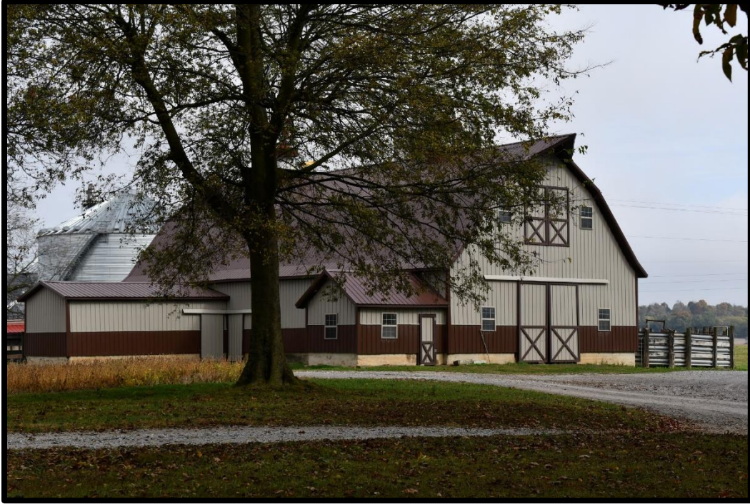
Plate 142. CA-449C, Dairy Barn, south (front) and west elevations, looking northeast.
