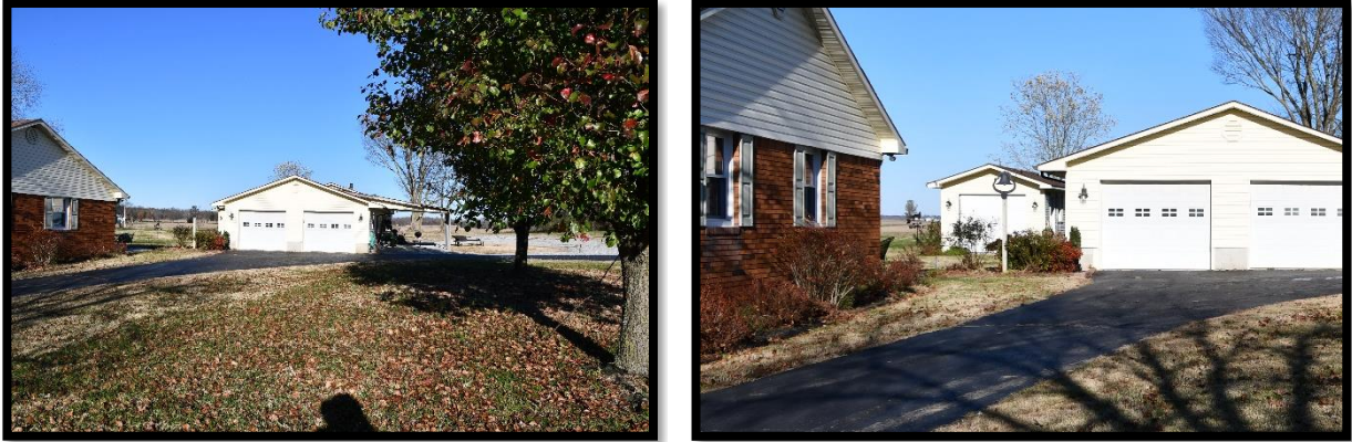
Plate 68. Left: CA-492B, Garage, looking north. Right: CA-492C, Workshop, looking north.
