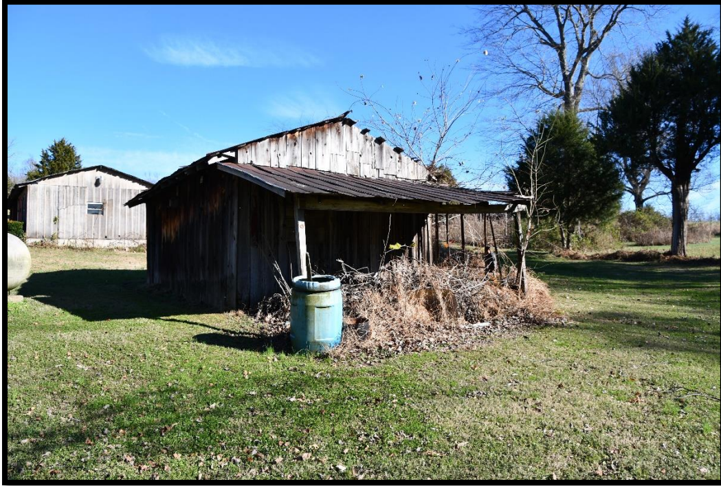
Plate 40. CA-482B, Shed, looking north.
