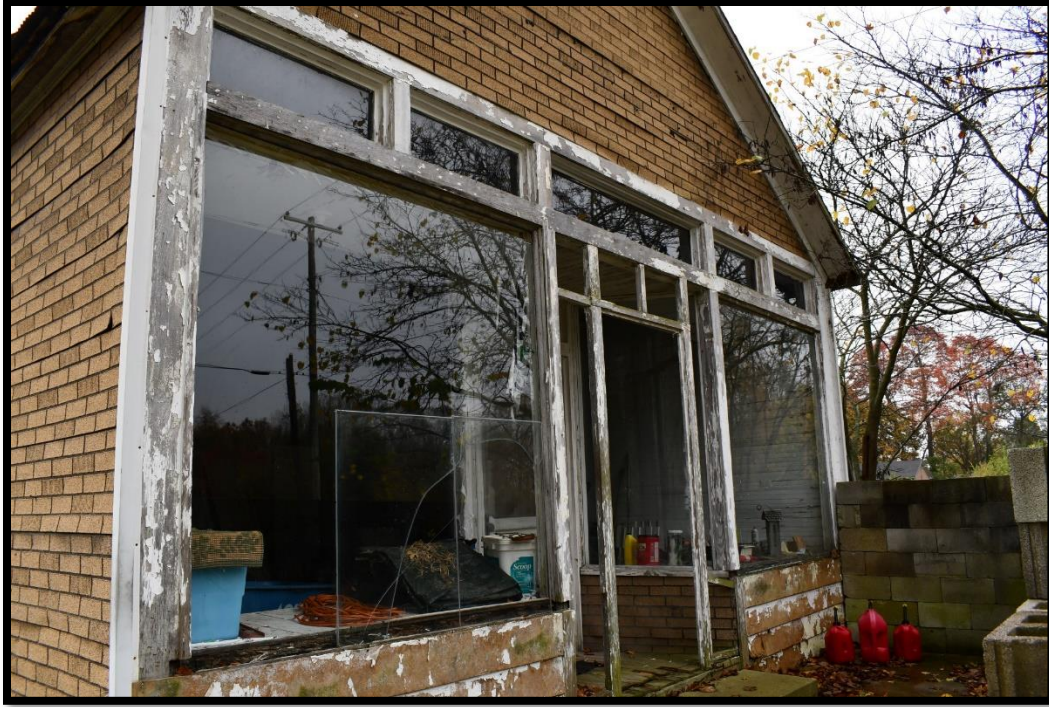
Plate 133. CA-20, Crider Store storefront detail, northwest elevation, looking southwest.
