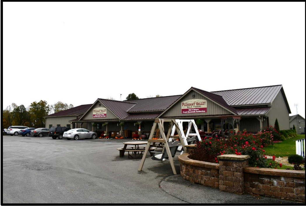
Plate 155. CA-453B, Store, northeast (front) and northwest elevations, looking south.
