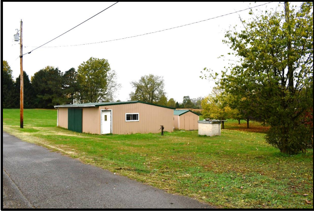
Plate 102. CA-19, Garage (B), shed (C), and well house (D) southwest and southeast elevations, looking north.
