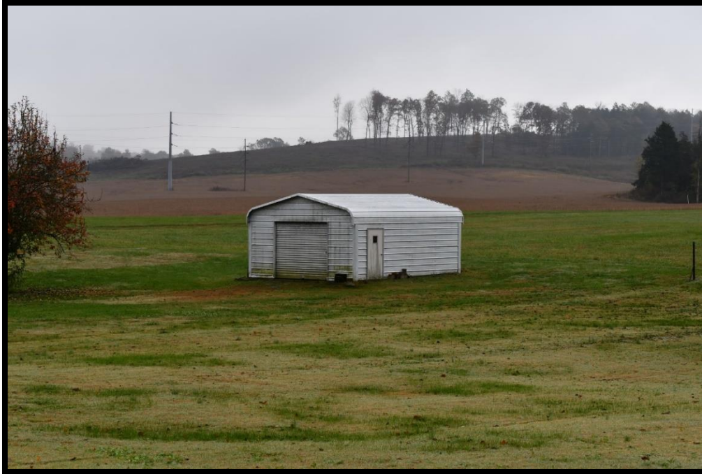
Plate 129. CA-447C, Garage, northwest and southwest elevations, looking east.
