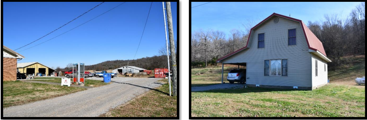
Plate 9. Left: CA-470C, Garage (left); and CA-470B, Barn (right), looking NW. Right: CA-470D, Modern House, looking NE.
