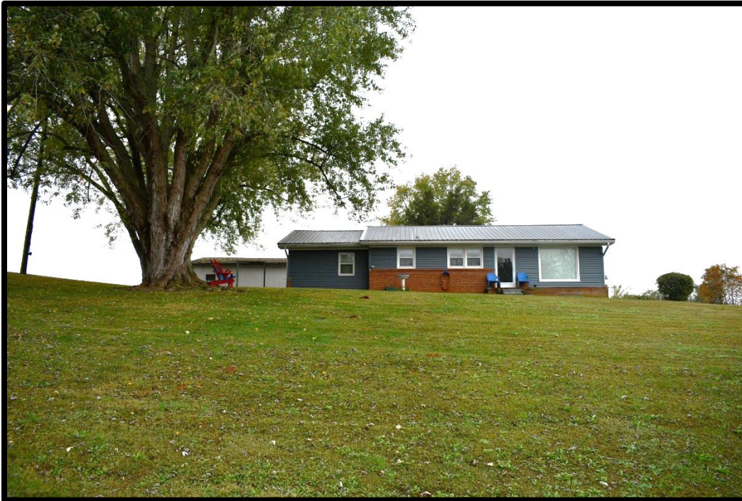
Plate 79. CA-435, House and Garage, northeast elevations, looking southwest.
