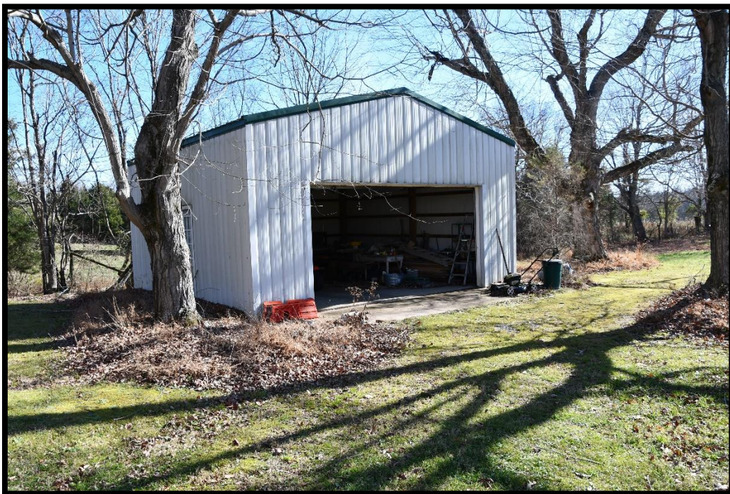
Plate 50. CA-484B, Garage, looking SE.
