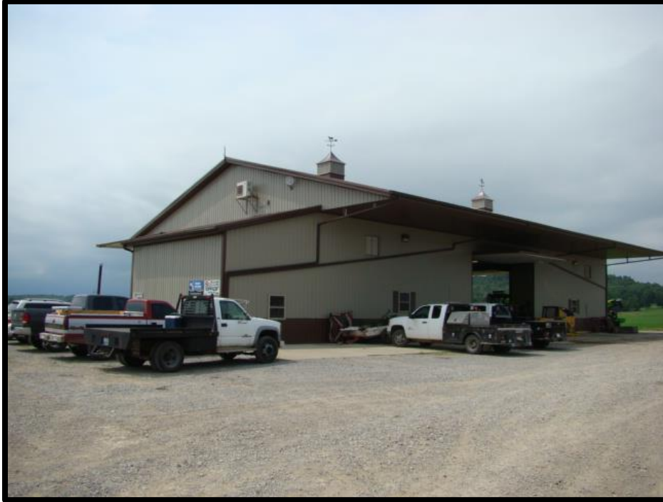
Plate 146. CA-449G, the Modern barn/office, south and east elevations, looking northwest.
