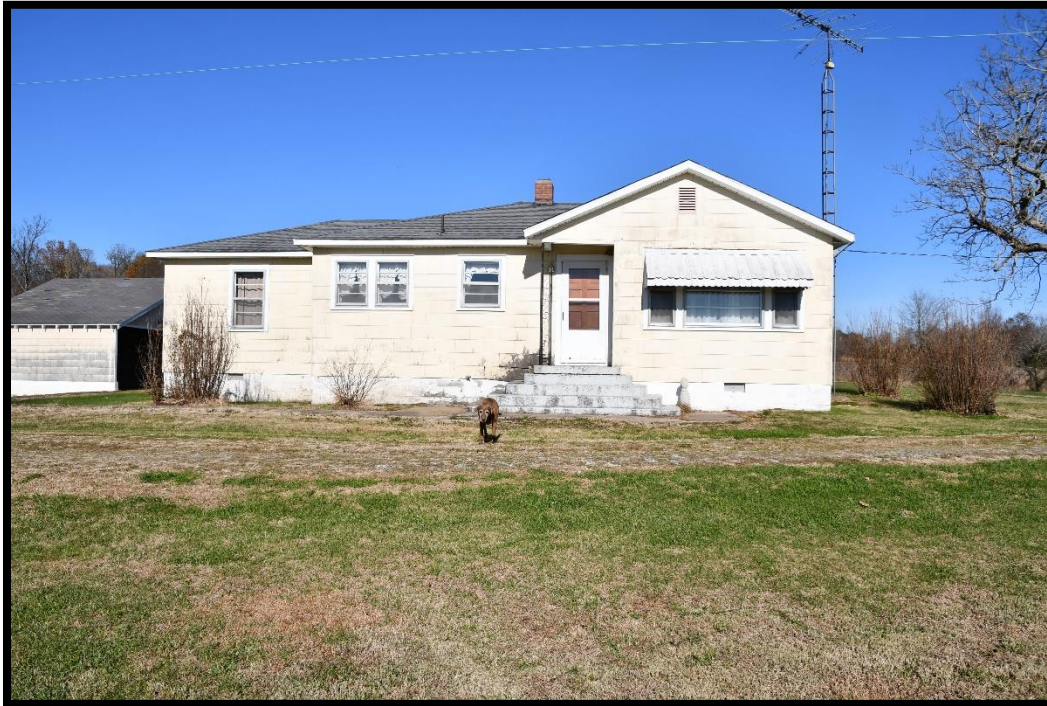
Plate 57. CA-487, House, looking NE.
