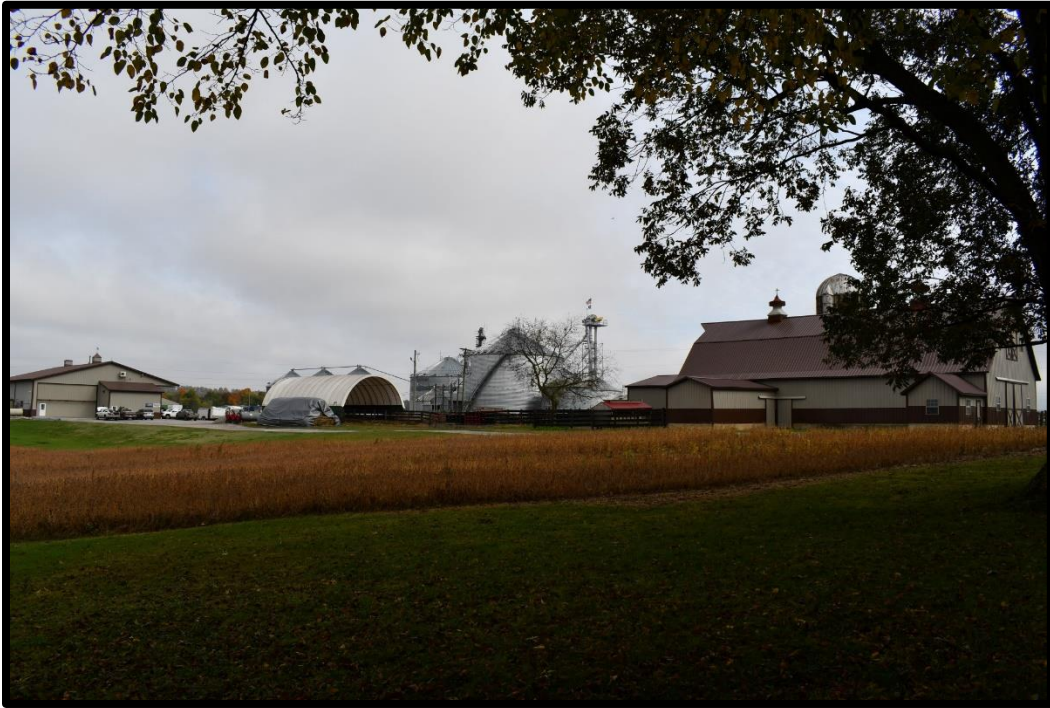
Plate 141. CA-449, Clift Farm Barns and Outbuildings, looking northeast.
