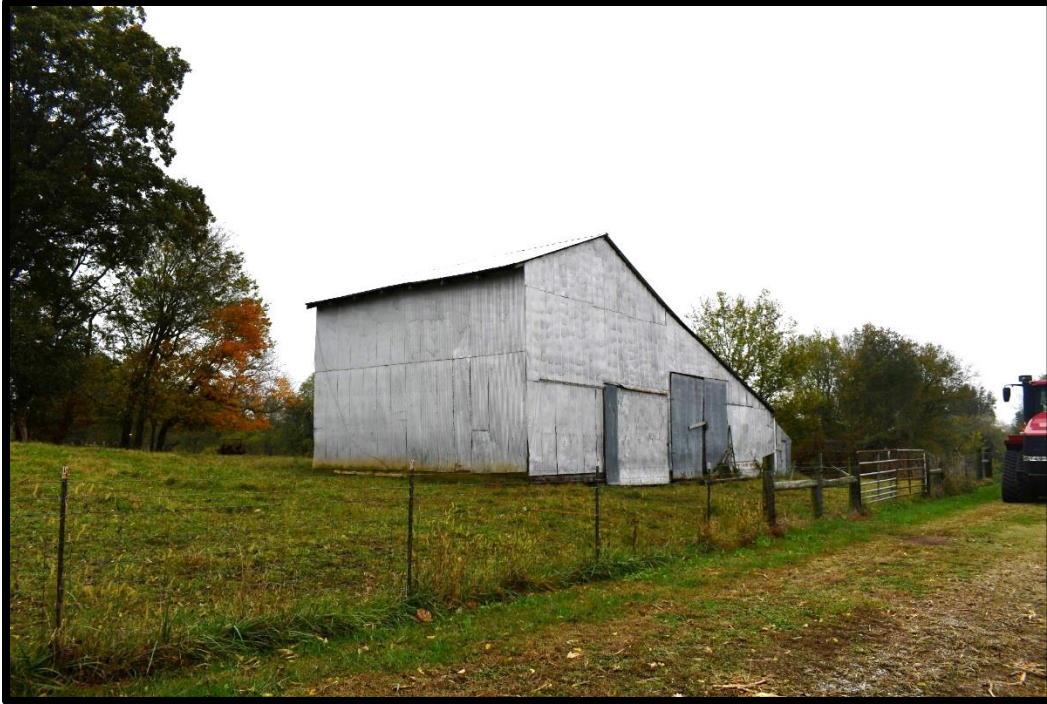
Plate 95. CA-439C, Transverse frame barn, northwest and southwest elevations, looking southeast.
