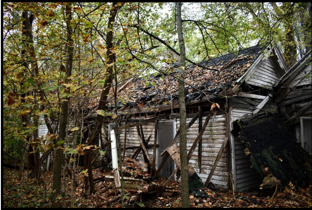
Plate 106. CA-465, House, southwest (front) and northeast elevations, looking west.
