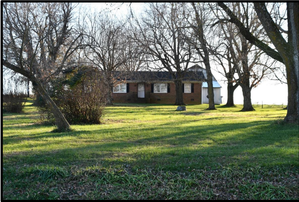
Plate 149. CA-450, House, northeast elevation, looking southwest.
