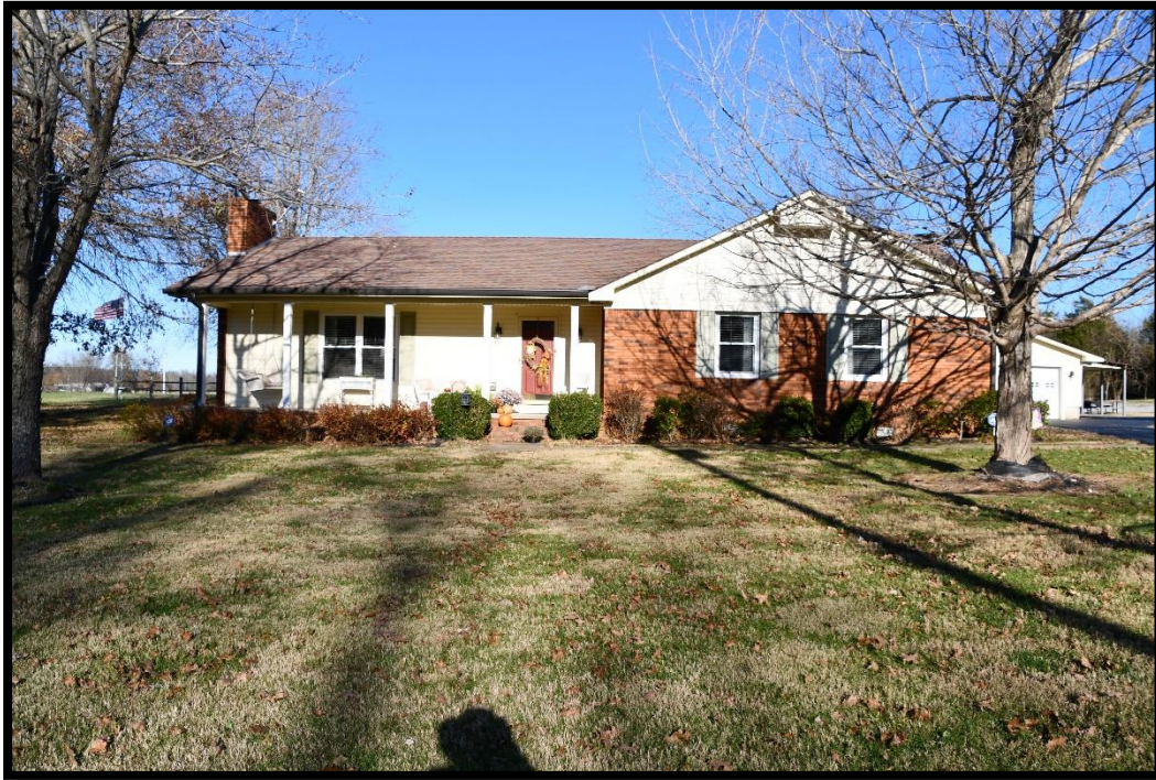
Plate 67. CA-492, House, looking NE.
