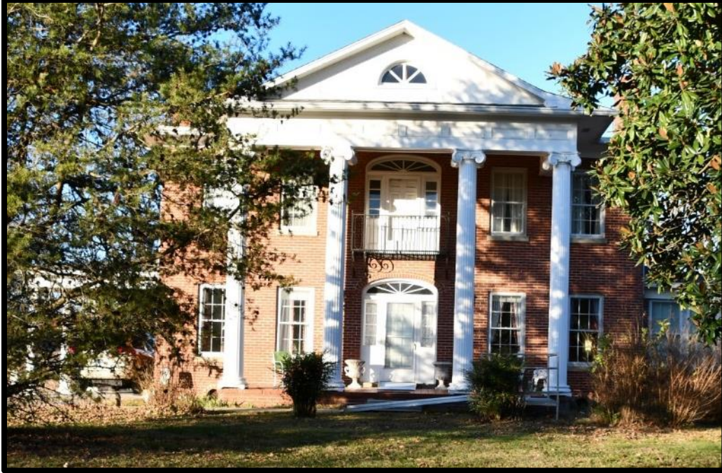
Plate 139. CA-449A, House, portico detail, south (front) elevation, looking north.
