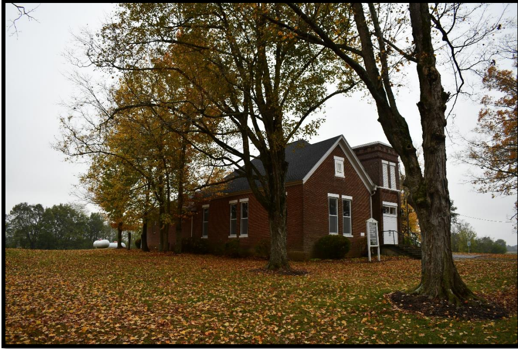
Plate 105. CA-17, Crider Baptist Church, looking southwest.
