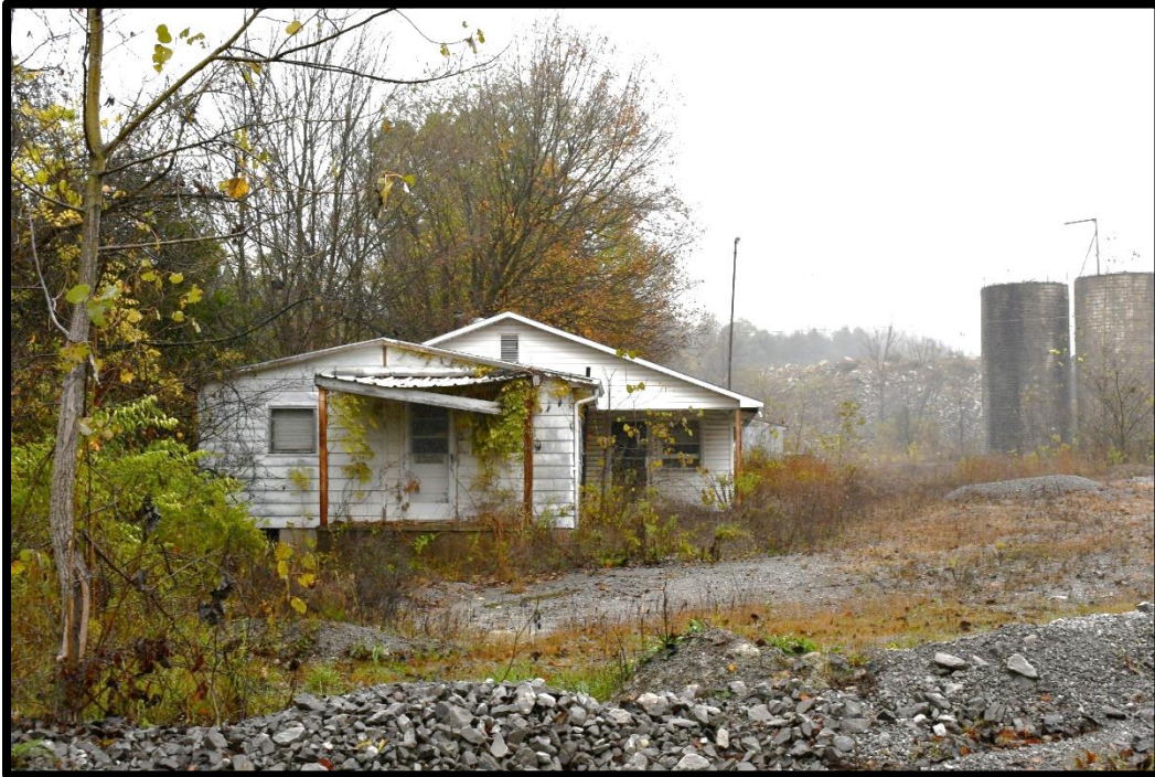
Plate 69. CA-347, Fredonia Quarry Office, southwest elevation, looking northeast.
