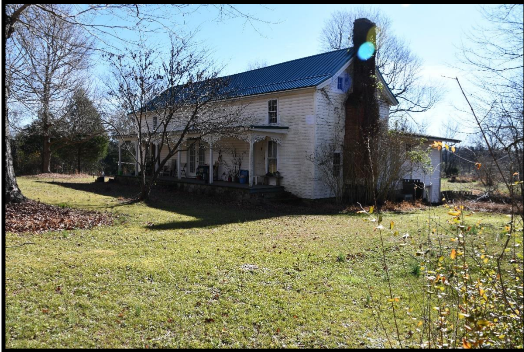
Plate 49. CA-484, House, looking SE
