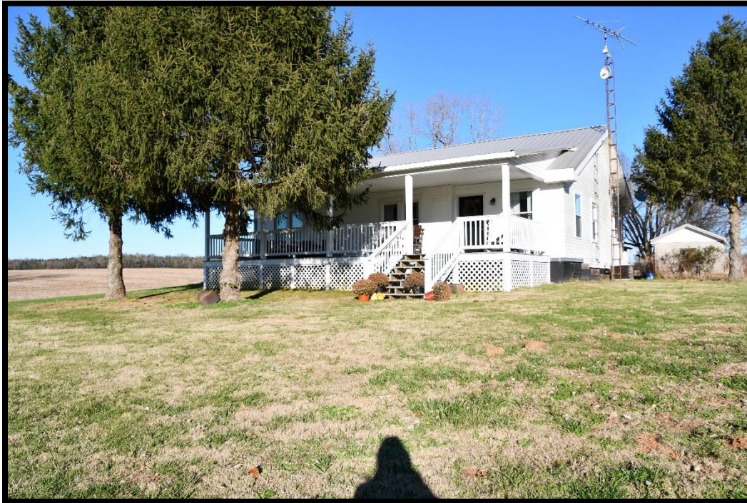
Plate 26. CA-478, House, looking NE.
