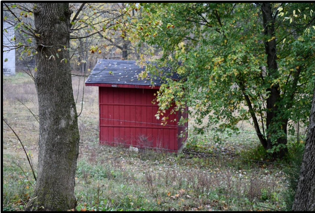
Plate 86. CA-18H, Shed, east elevation, looking west.
