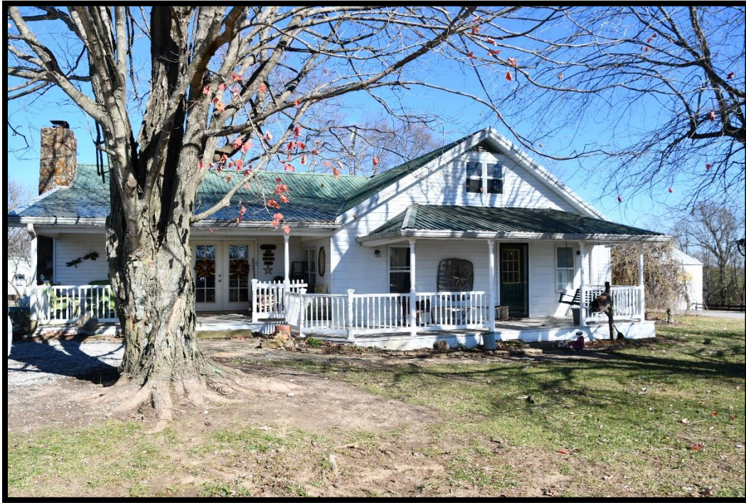
Plate 15. CA-474, House, looking NE.
