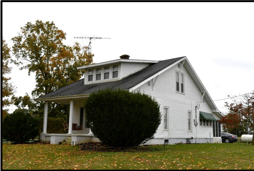
Plate 151. CA-452A, House, northeast (front) and northwest elevations, looking south.
