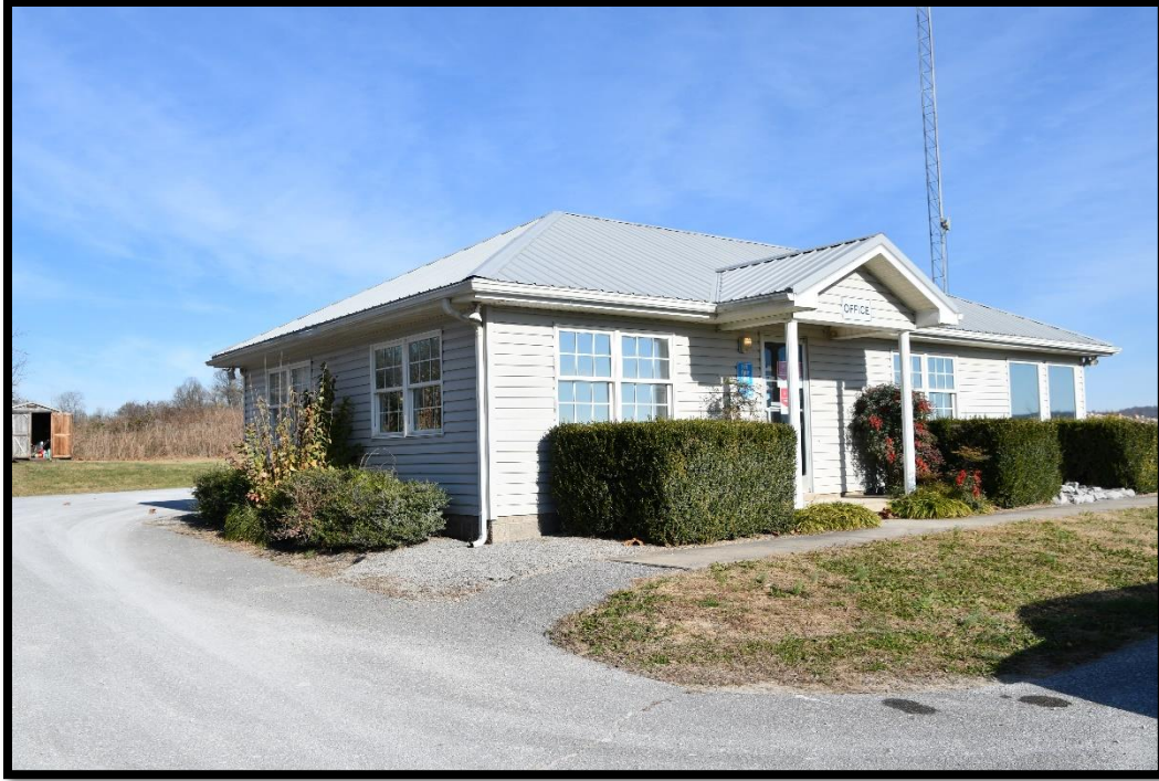
Plate 74. CA-347, Fredonia Quarry. CA-347F Modern office and CA-347G, storage shed (back left), façade and south elevation, looking northwest.
