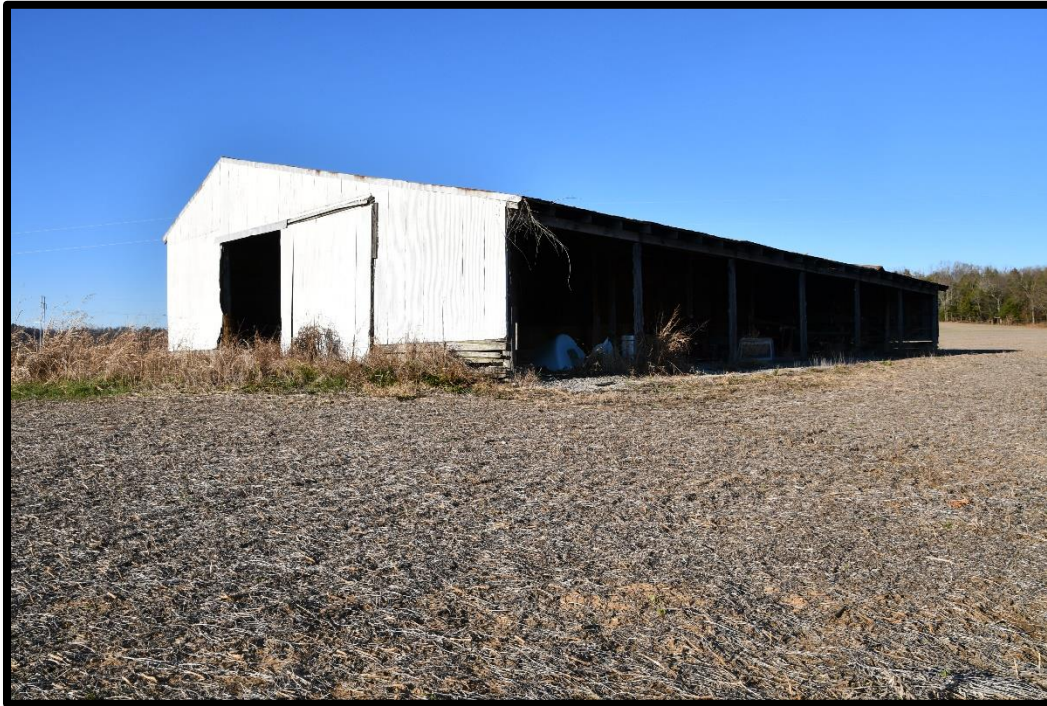
Plate 29. CA-479, Barn, looking north.
