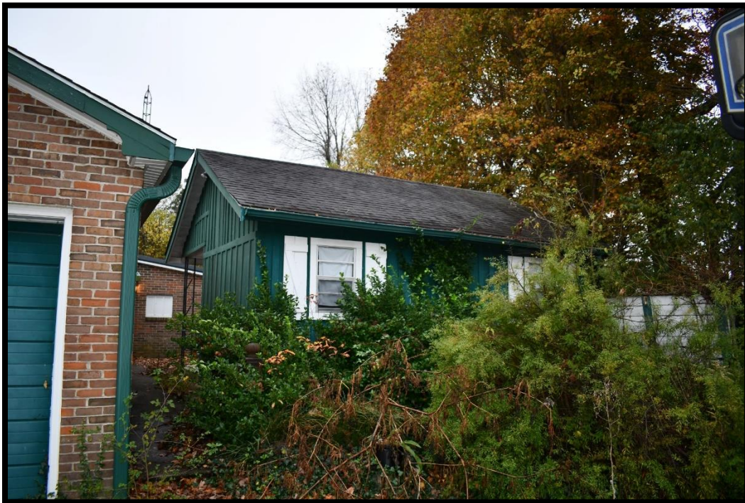
Plate 113. CA-443B, Shed, northwest elevation, looking southeast.
