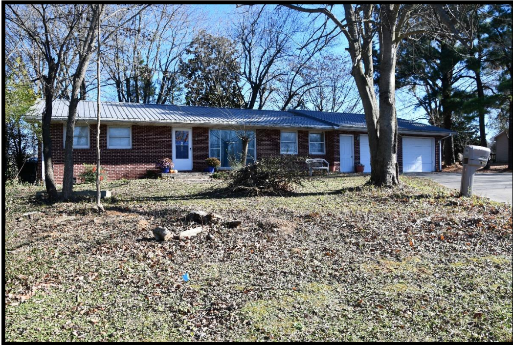
Plate 1. CA-466, House, looking NE.
