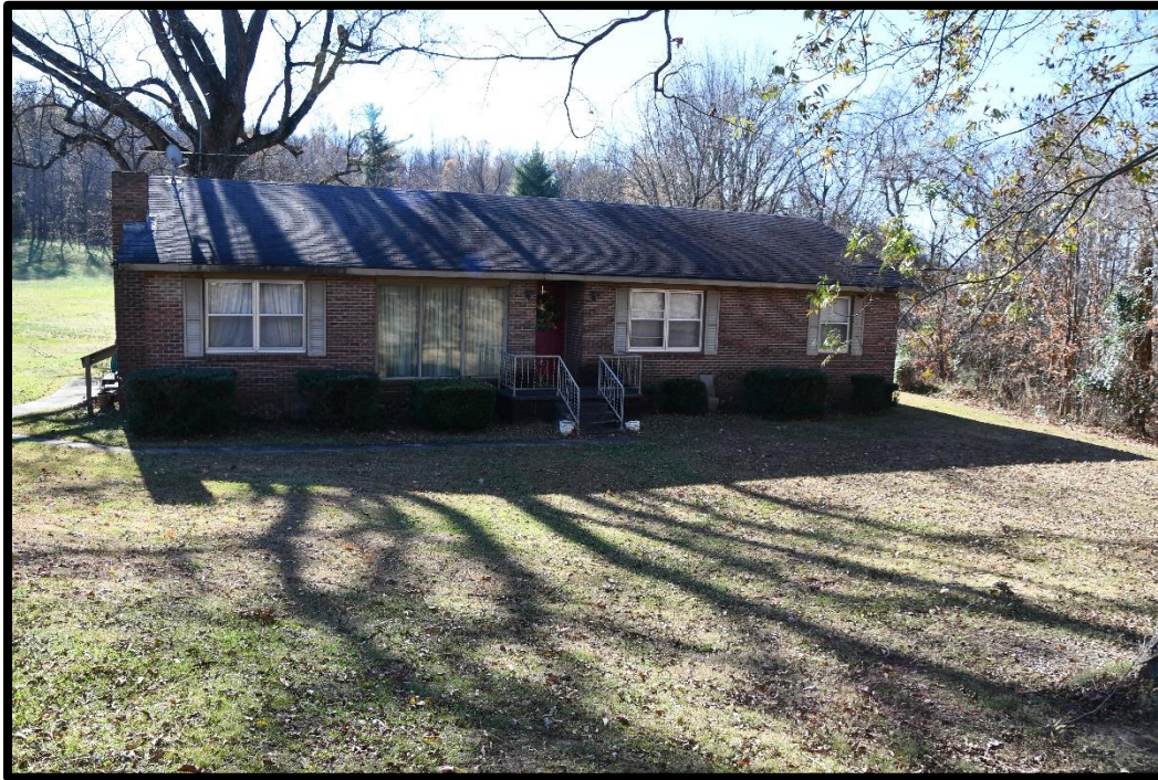
Plate 39. CA-482, House, looking south.
