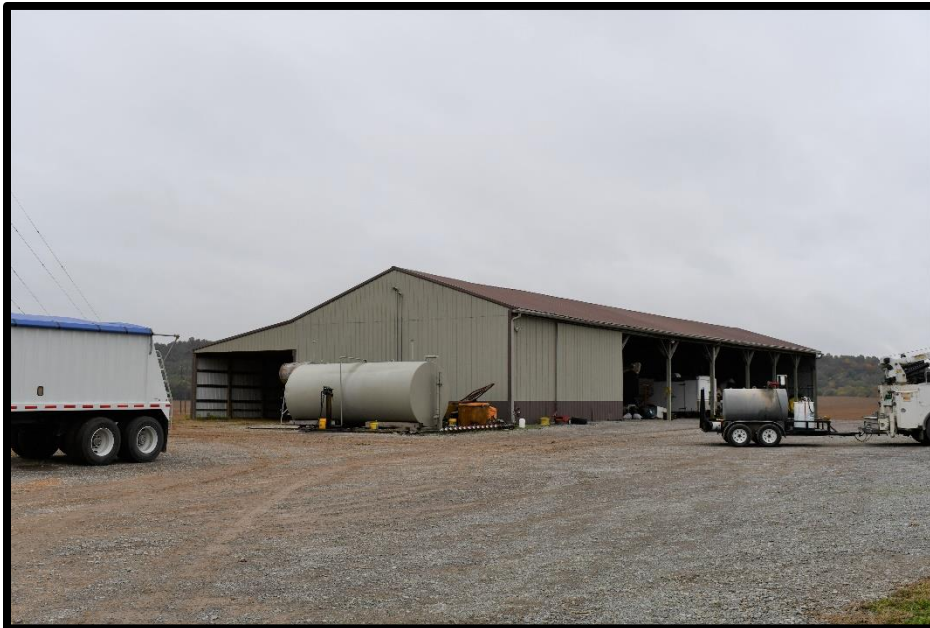
Plate 147. CA-449H, Equipment barn, south and east elevations, looking northwest.
