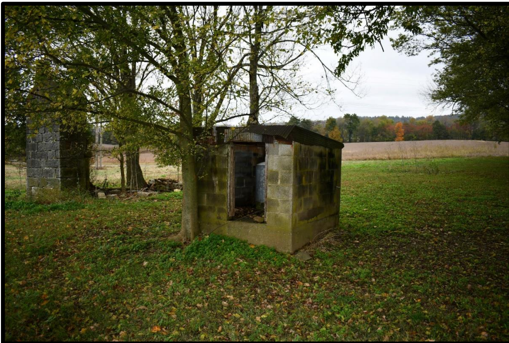
Plate 158. CA-454B, Pump house, looking northeast.
