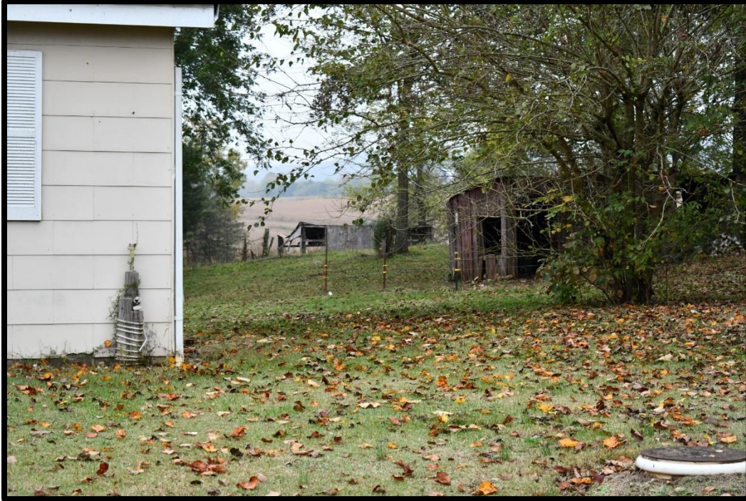
Plate 92. CA-438D and CA-438E, Sheds, southeast elevations, looking northwest.
