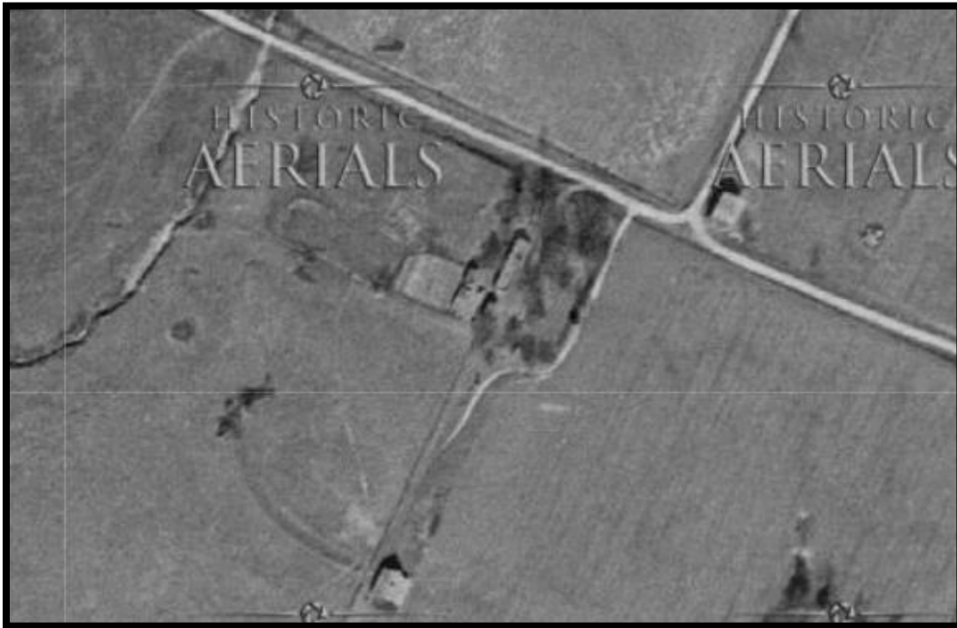
Figure 12. Aerial of Adamson Farm, 1952 (NETR 1952).
