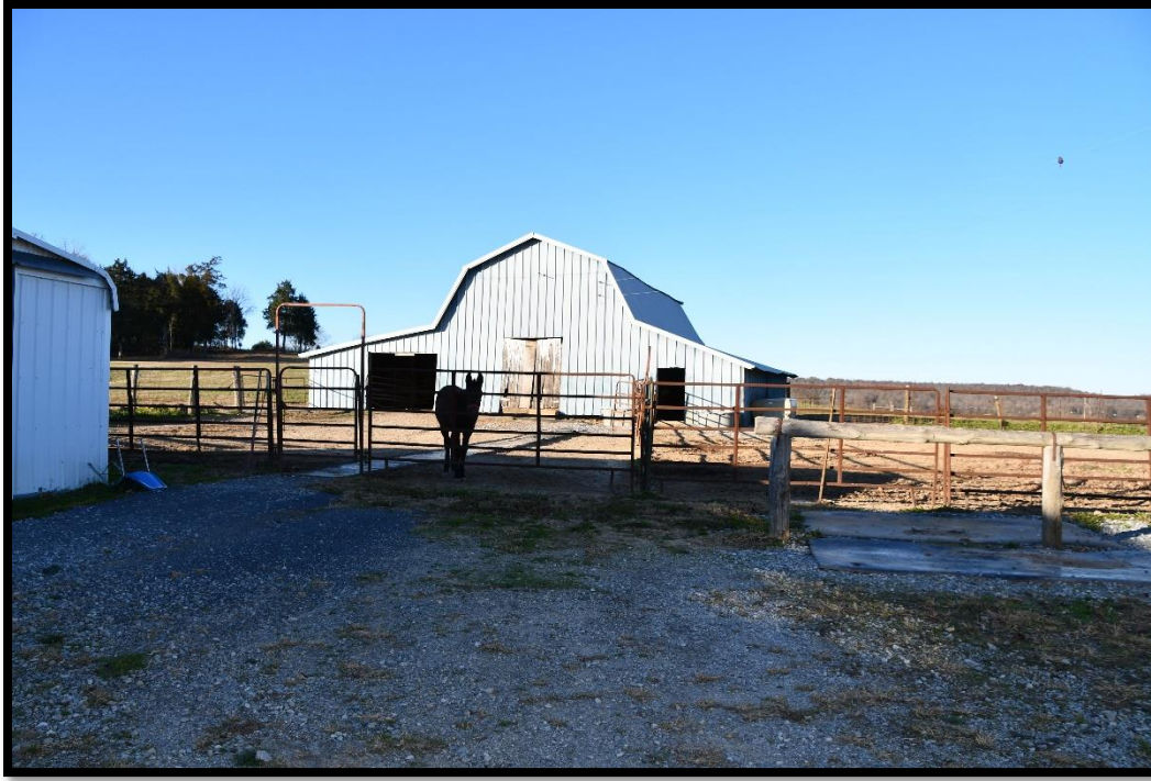
Plate 31. CA-480B, Barn, looking north.
