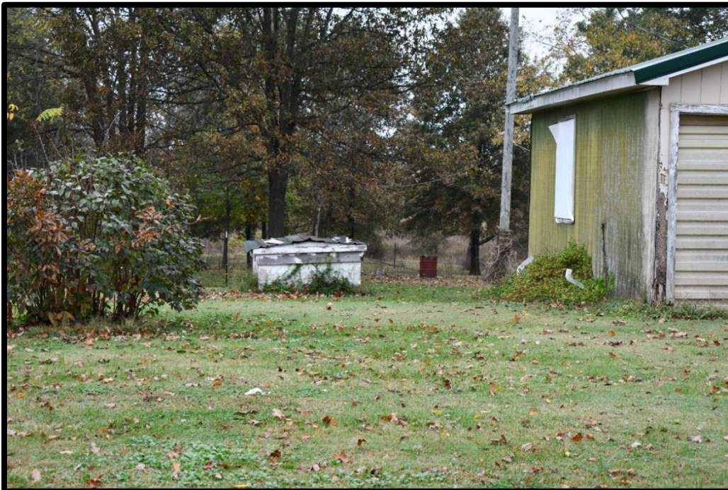
Plate 91. CA-438C, Well house, southeast elevation, looking northwest.
