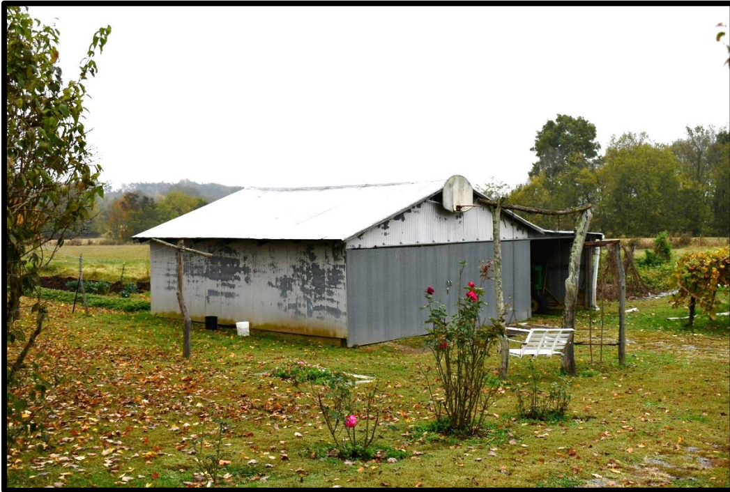
Plate 94. CA-439B, Garage, northwest and southwest elevations, looking east.
