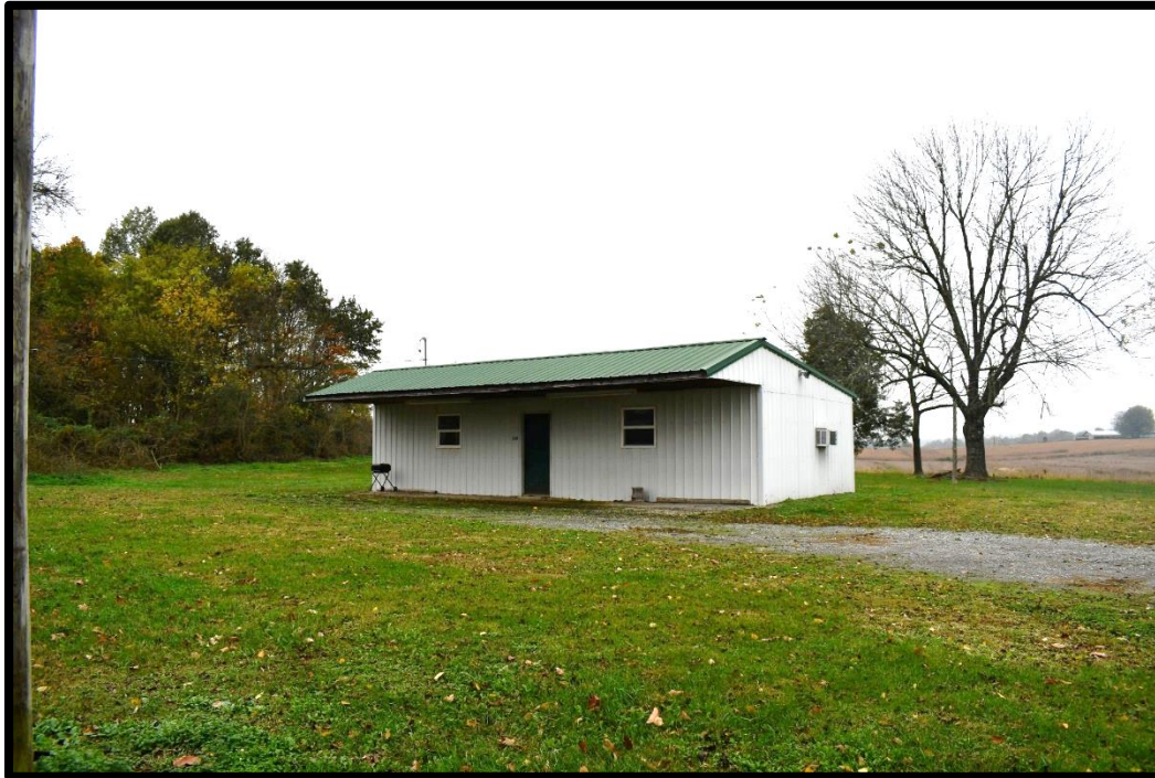
Plate 96. CA-440, Crider Sportsman Club, southeast (front) and northeast elevations, looking west.
