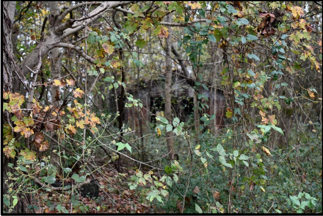
Plate 116. CA-444B, Garage, looking southwest.
