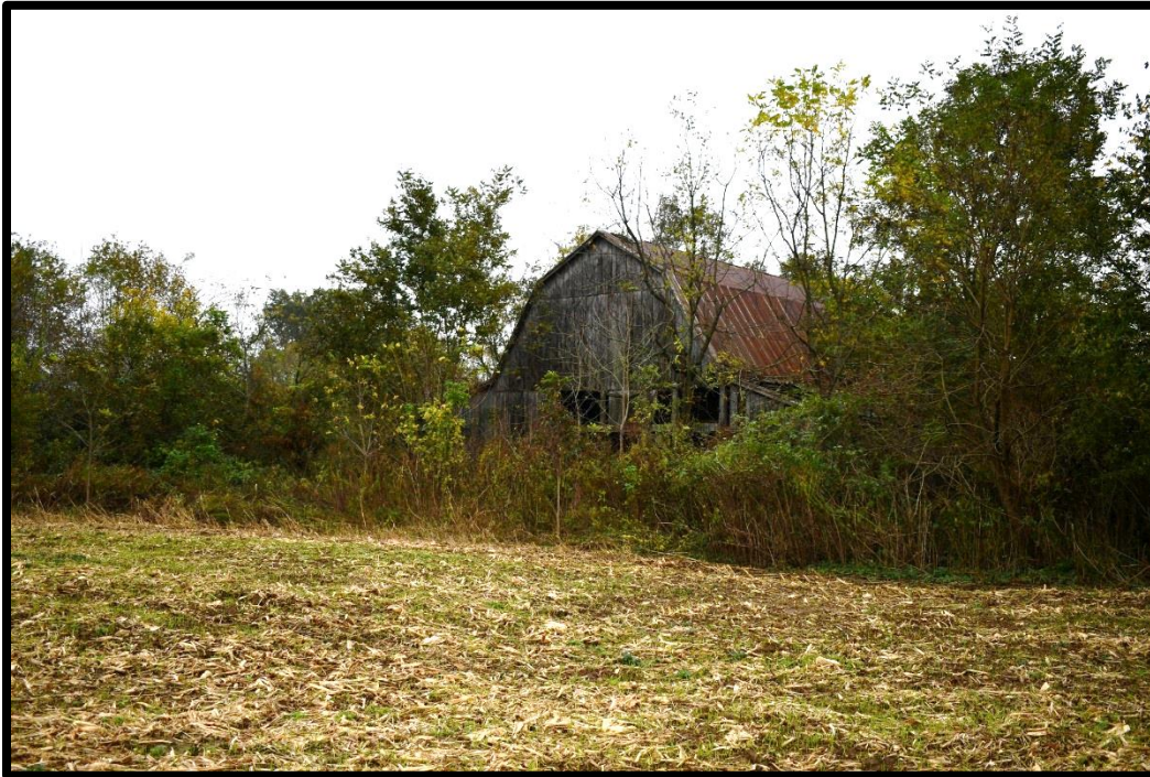
Plate 87. CA-436, Barn, north elevation, looking southeast.
