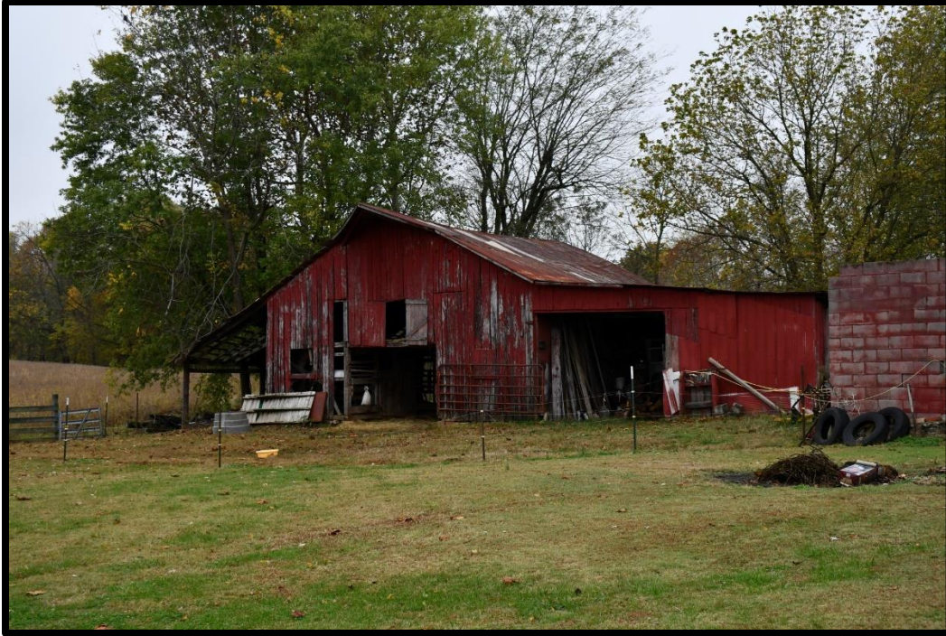
Plate 85. CA-18E and CA-18F, Barn and concrete block outbuilding, southeast elevation, looking northwest.
