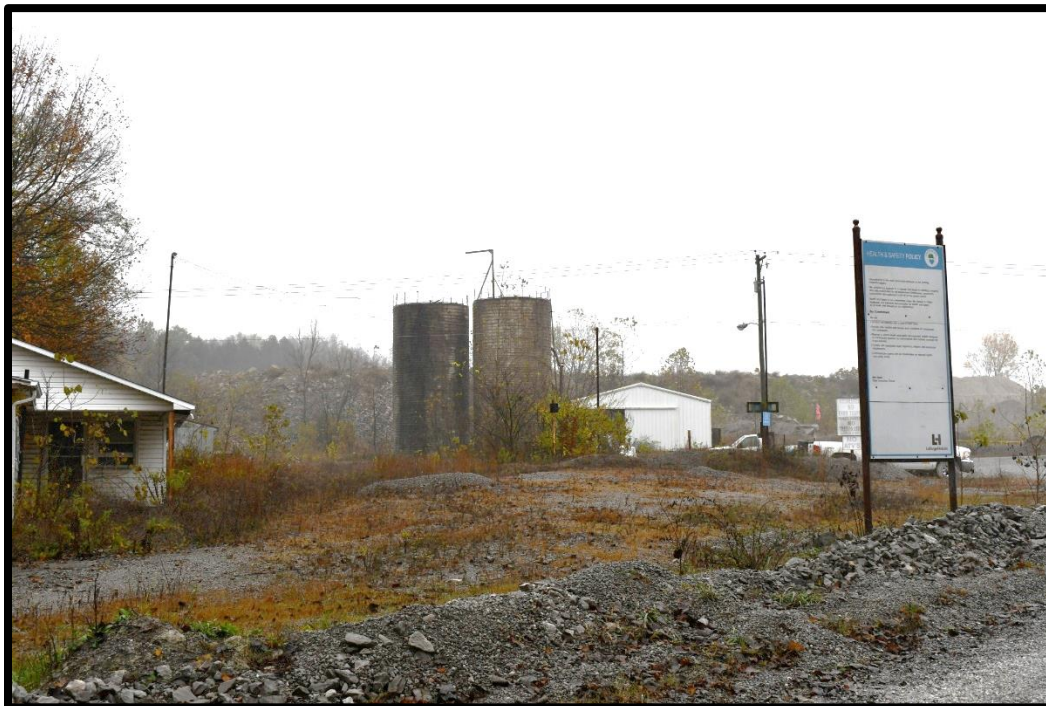
Plate 71. CA-347A to 347C, Fredonia Quarry barn and silos, southwest elevation, looking northeast.
