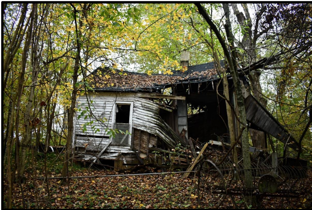
Plate 107. CA465, House, northeast elevation of north addition, looking southwest.
