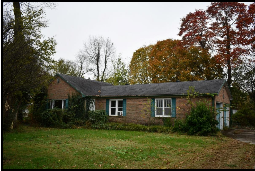
Plate 112. CA-443, House, northeast (front) and northwest elevations, looking southwest.
