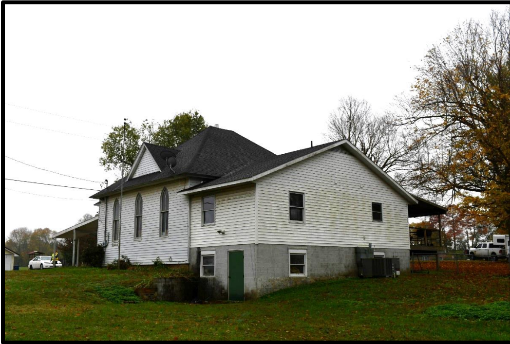
Plate 121. CA-16, Church, northeast and northwest elevations, looking south.
