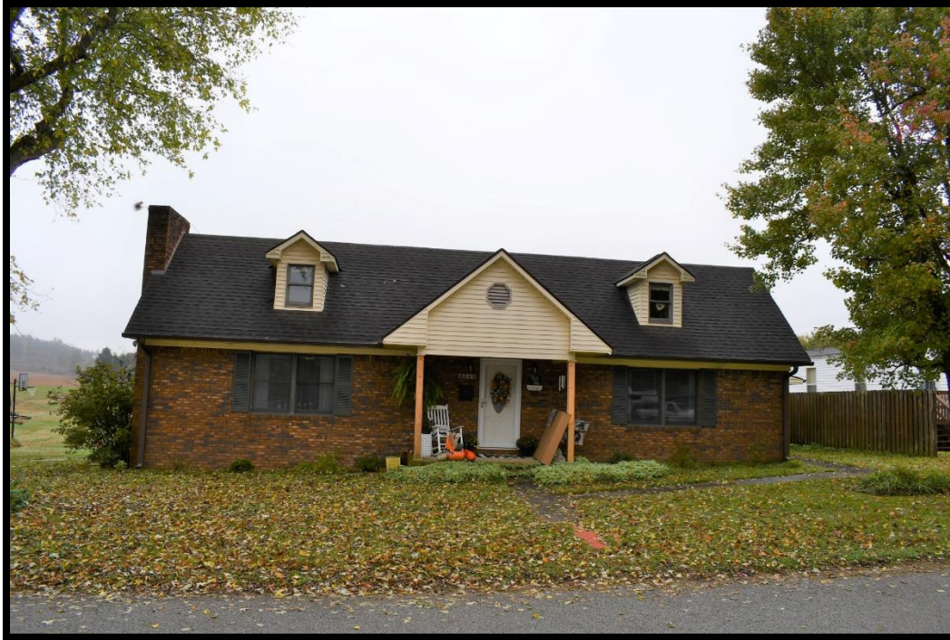
Plate 127. CA-447A, House, northwest elevation, looking southeast.
