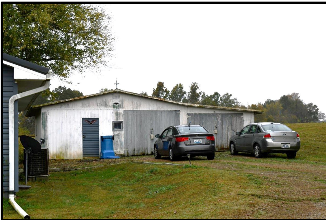
Plate 81. CA-435B, Garage, northwest (front) elevation, looking southeast.
