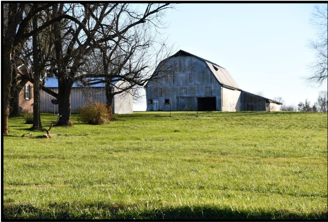
Plate 150. CA-450B Garage (left) and CA-450D, Stock Barn (right), north and west elevations, looking south.
