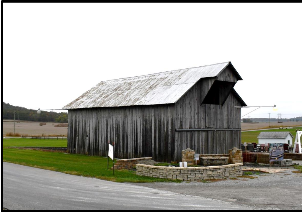
Plate 154. CA-453, Transverse frame barn, southwest (front) and northwest elevations, looking northeast.
