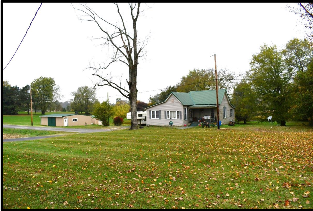
Plate 100. CA-19, the Major Brown House and Outbuildings, southeast (front) elevations, looking northwest.
