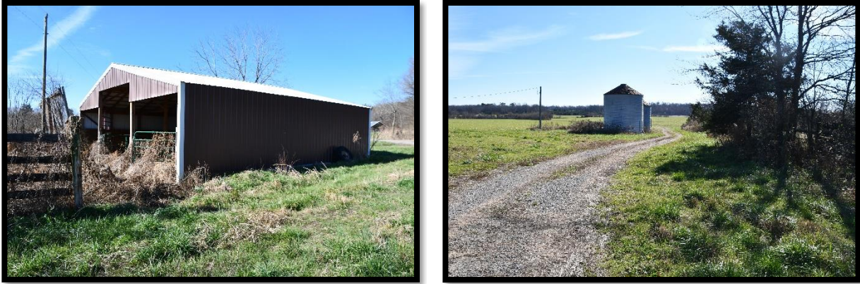
Plate 47. Left: CA-483E, Barn, looking SW. Right: CA-483F, Two silos, looking SE.
