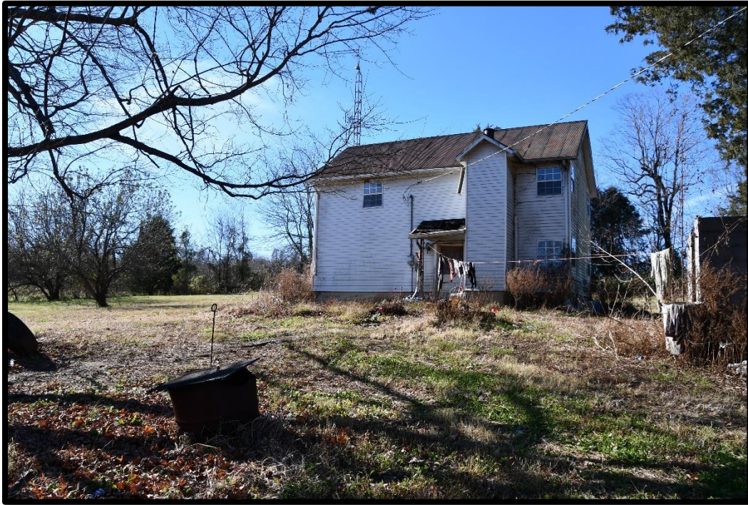
Plate 44. CA-483, House, looking SW.
