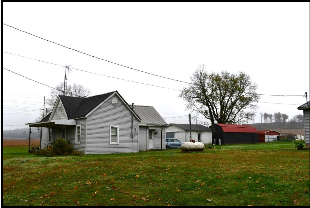
Plate 124. CA-446, House and outbuildings, northwest (front) and southwest elevations, looking east.
