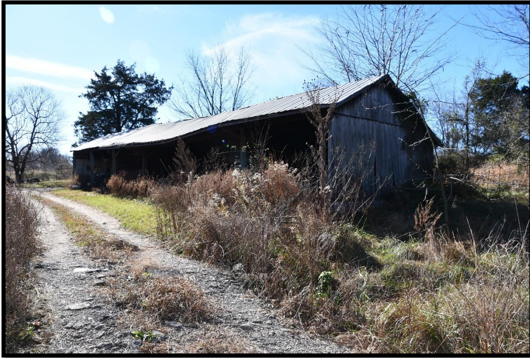
Plate 45. CA-483B, Machine shed, looking south.
