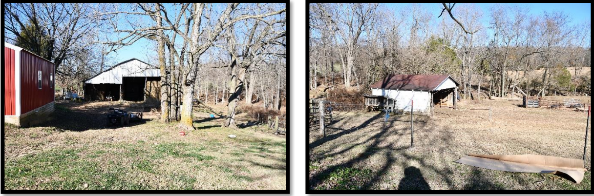
Plate 64. Left: CA-489E, Barn, looking north. Right: CA-489F, Barn, looking NE.
