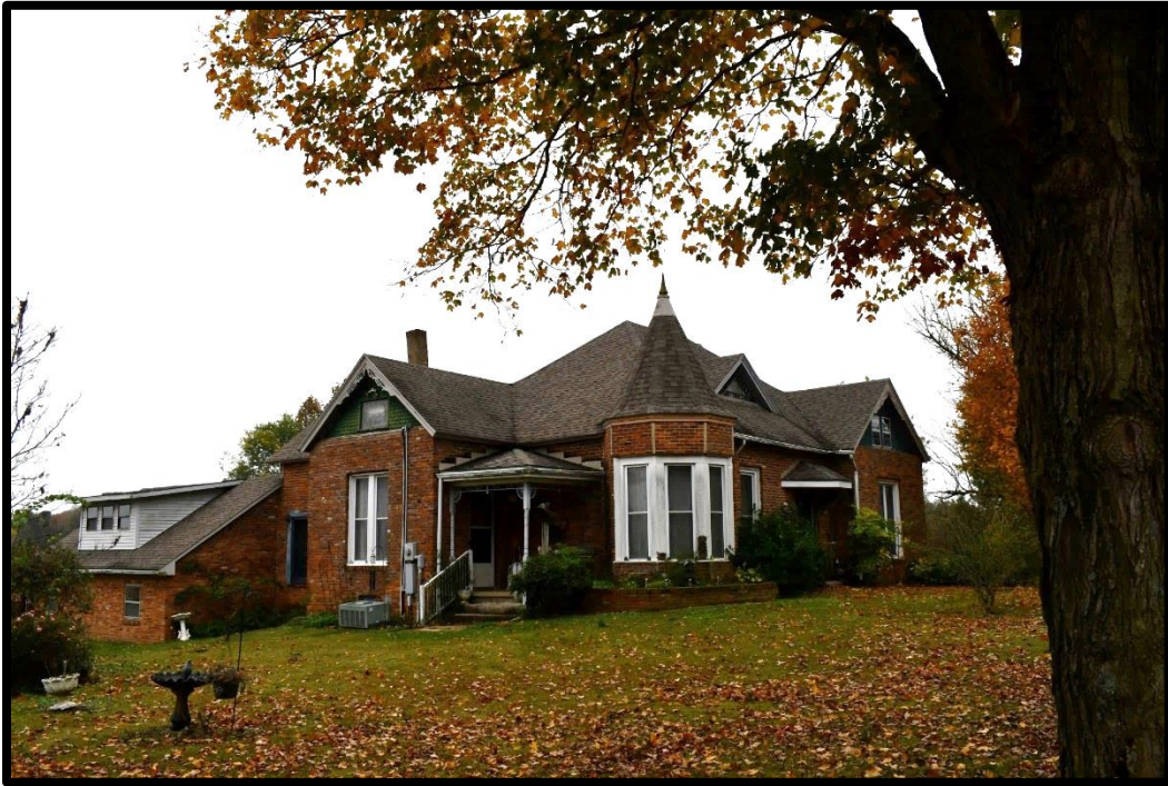
Plate 82. CA-18, House, southeast and northeast elevations, looking northwest.
