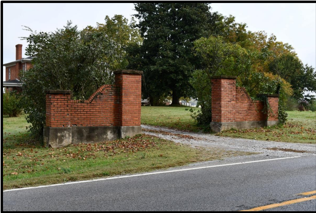
Plate 140. CA-449B, Driveway entry walls, southwest elevations, looking northeast.
