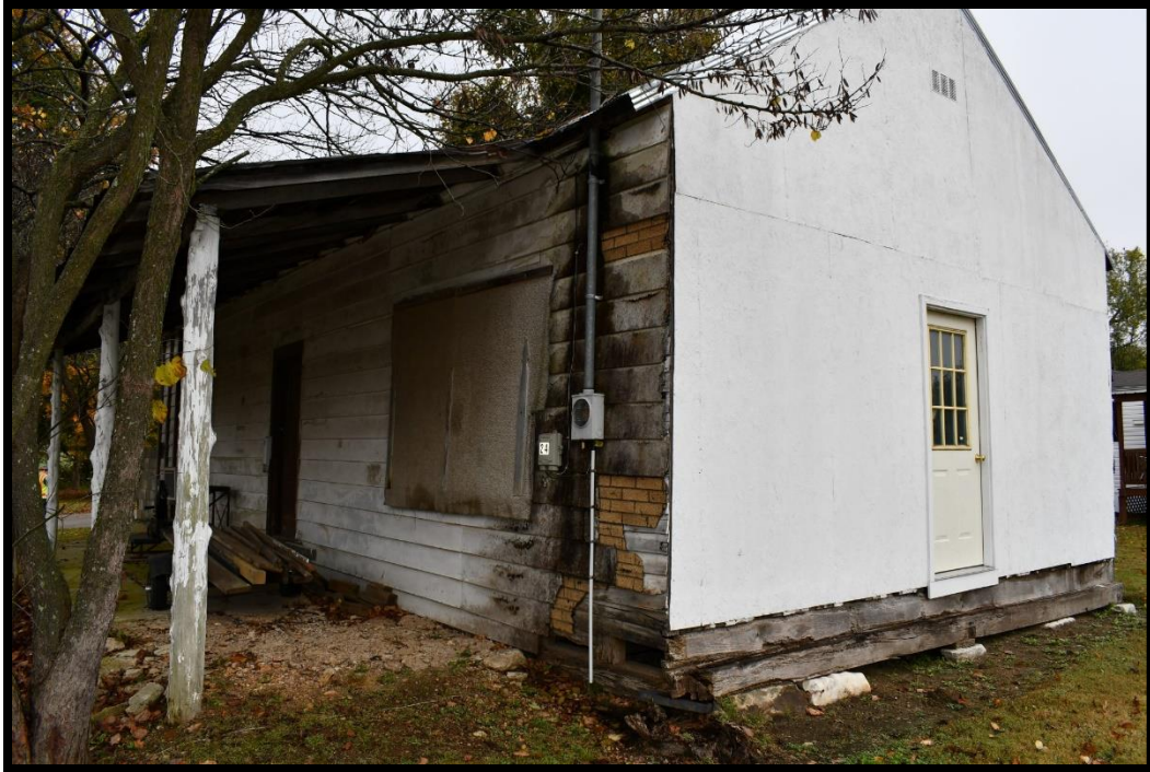
Plate 131. CA-20, Crider Store, southwest and southeast (rear) elevations, looking north.
