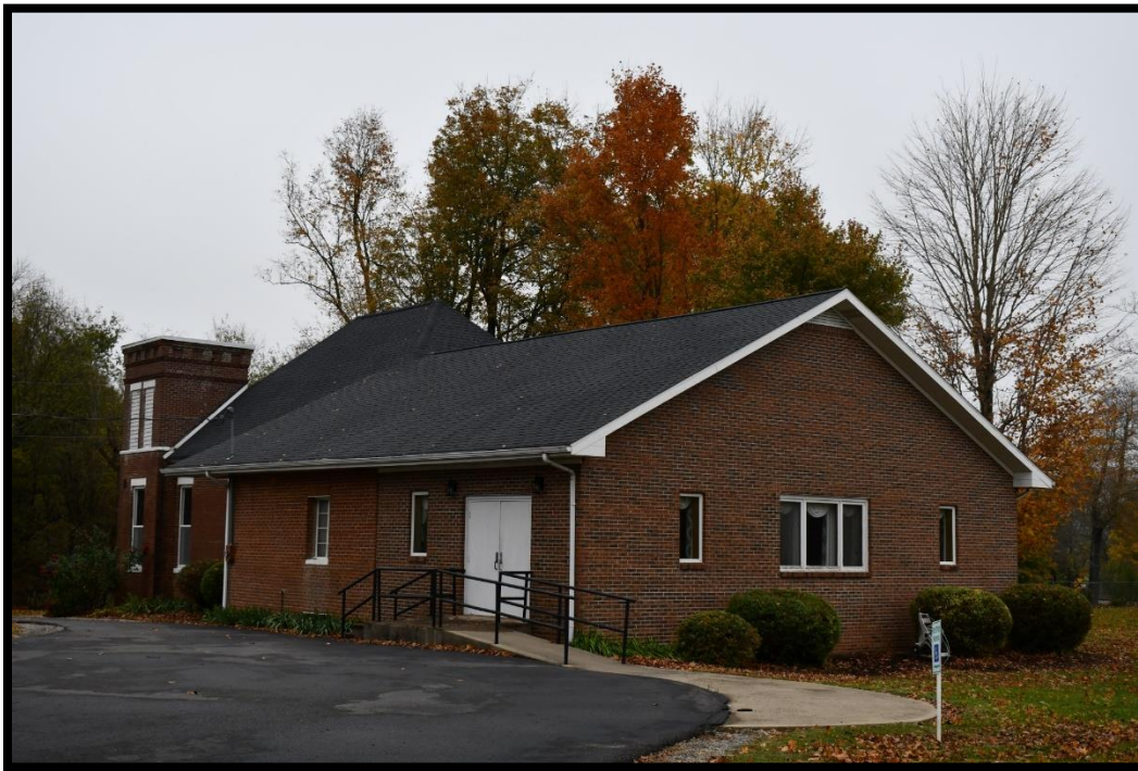
Plate 104. CA-17, Church, southeast and southwest elevations, looking north.
