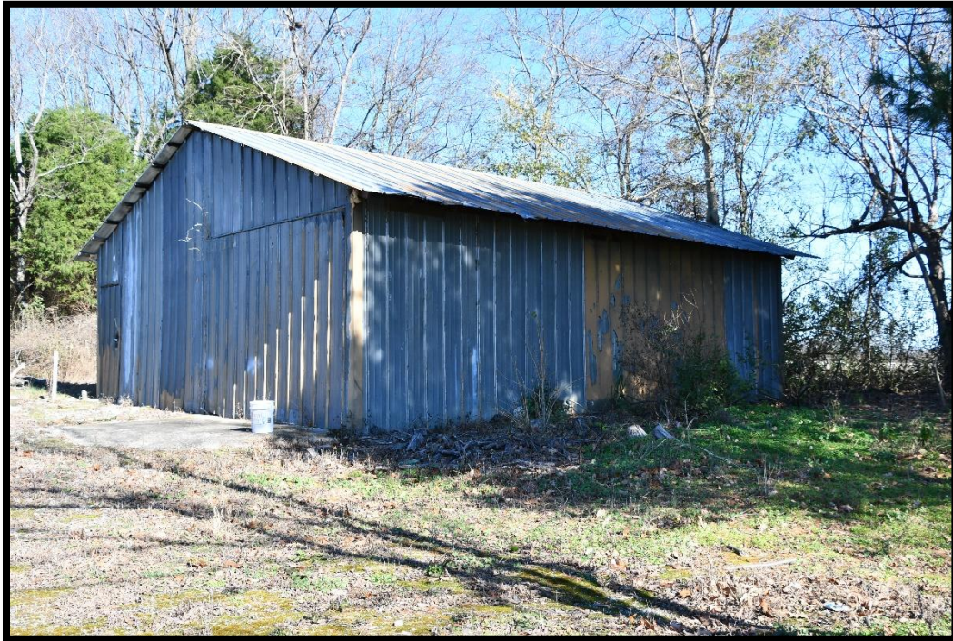
Plate 14. CA-473, Barn, looking NE.
