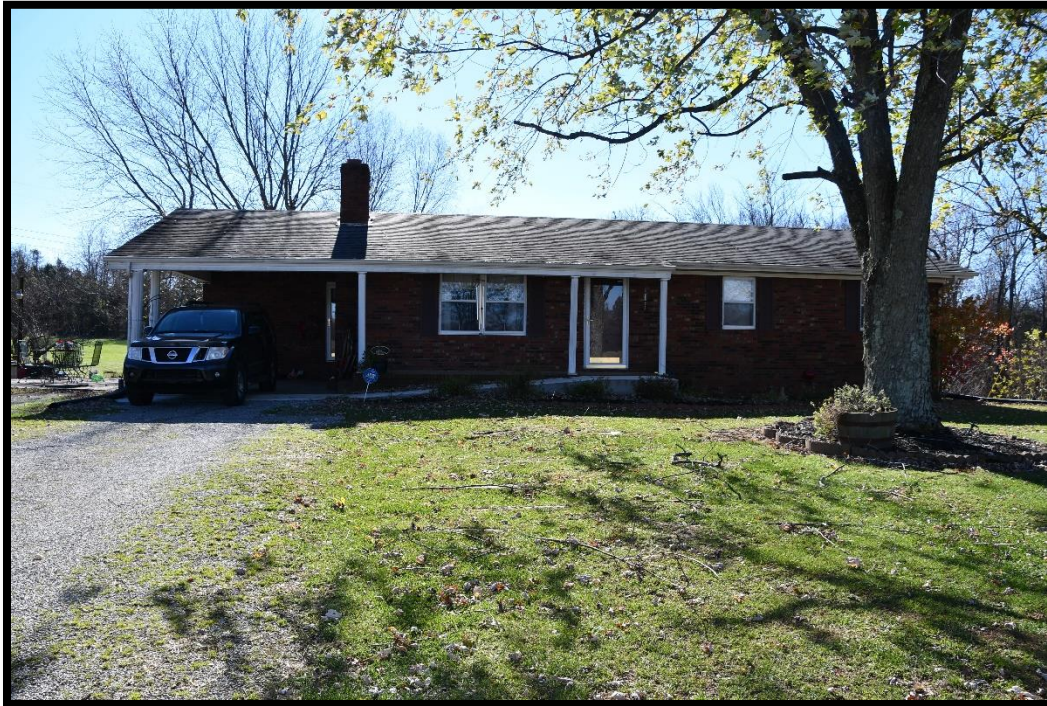
Plate 12. CA-472, House, looking south.
