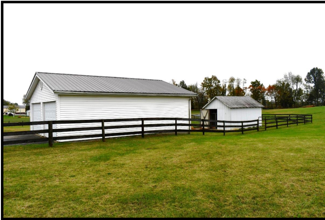
Plate 152. CA-452B and C, the modern garage (left) and the historic garage (right), northwest elevation, looking south.
