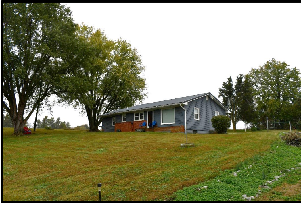
Plate 80. CA-435A, House, northeast (front) and northwest elevations, looking south.
