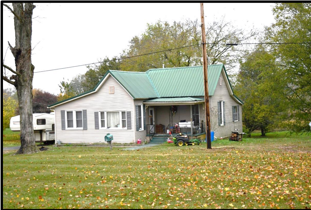
Plate 101. CA-19, House, southeast and northeast elevations, looking northwest.
