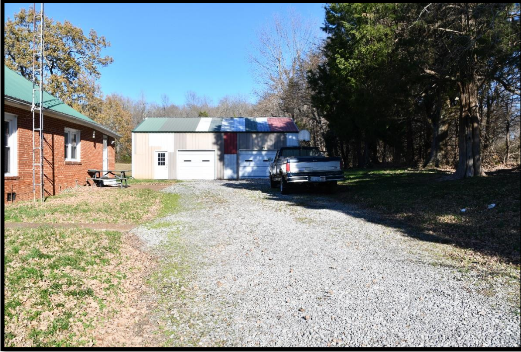
Plate 60. CA-488B, Garage, looking NE.
