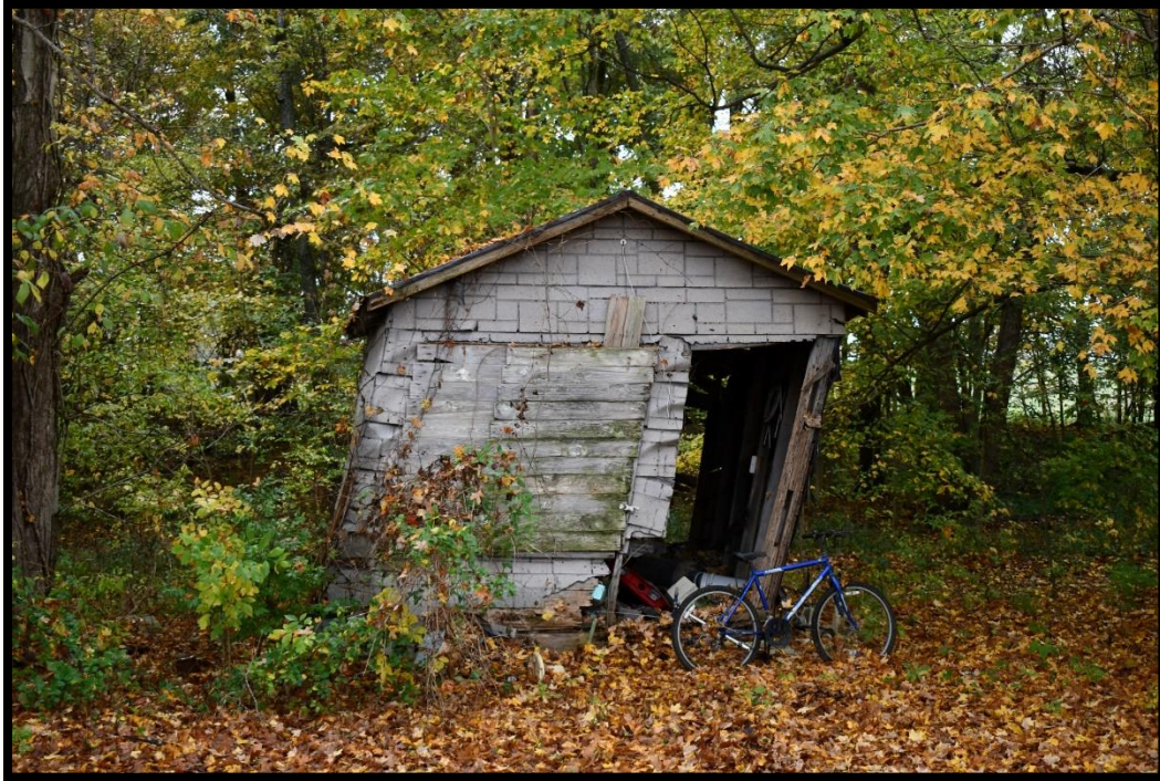
Plate 122. CA-445, Shed, southeast elevation, looking northwest.
