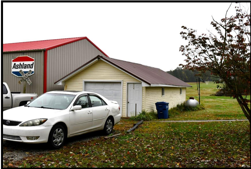
Plate 128. CA-447B, Garage, northwest and southwest elevations, looking east.
