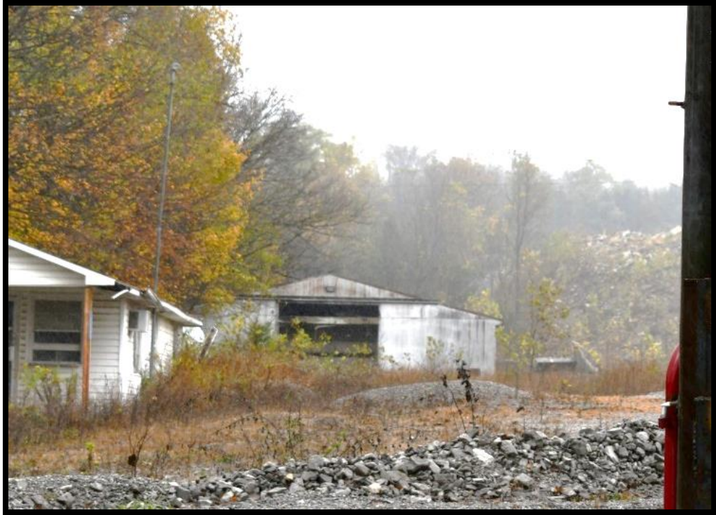
Plate 70. CA-347B, Fredonia Quarry barn, southwest elevation, looking northeast.
