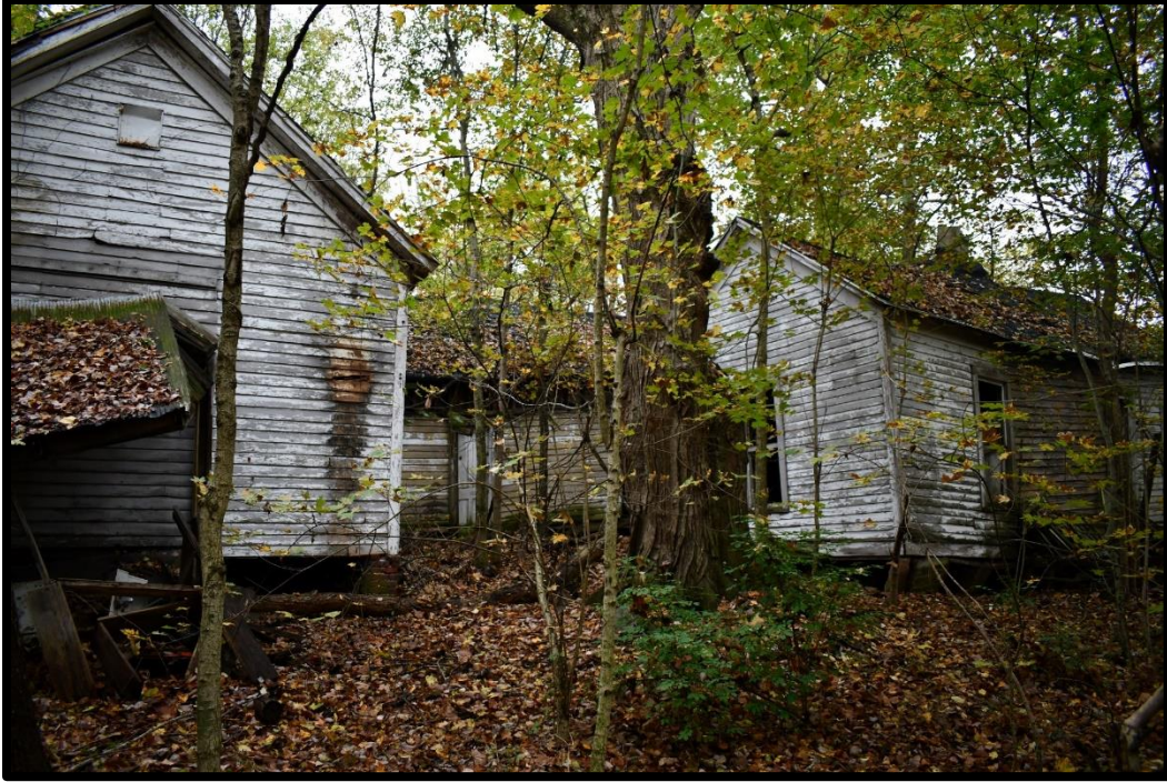
Plate 108. CA465, House, northwest elevation, looking south.
