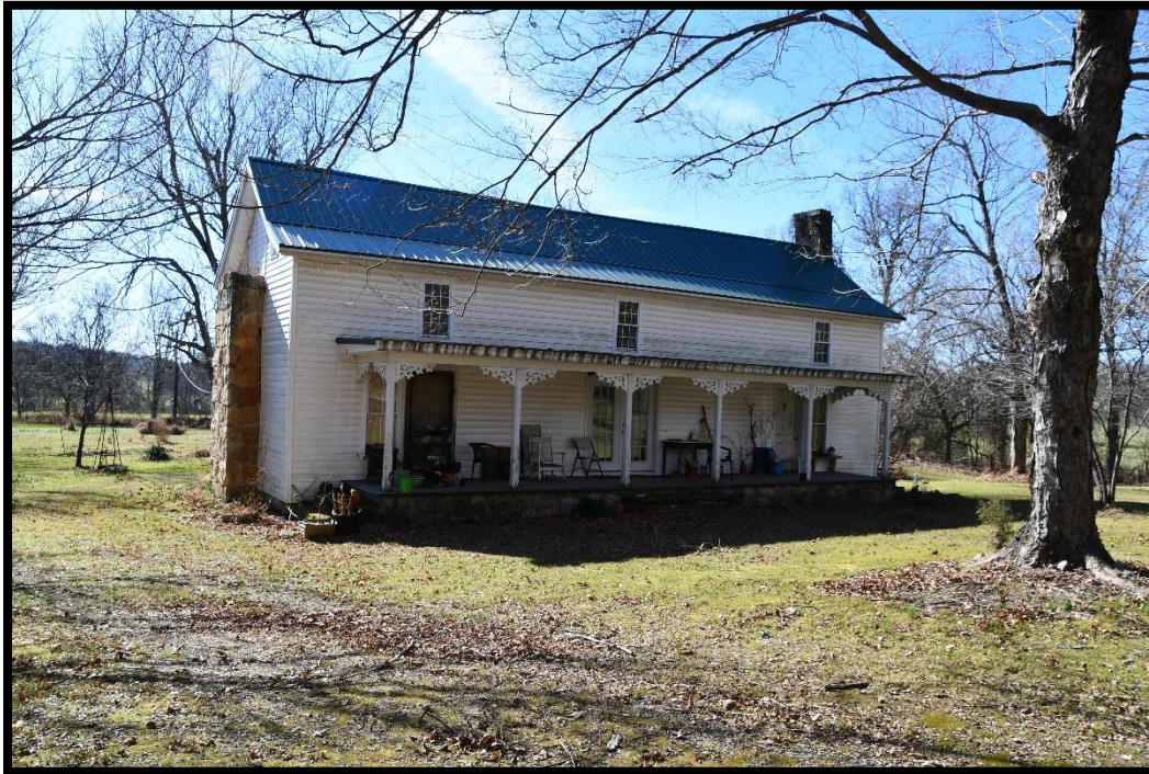
Plate 48. CA-484, House, looking SW.
