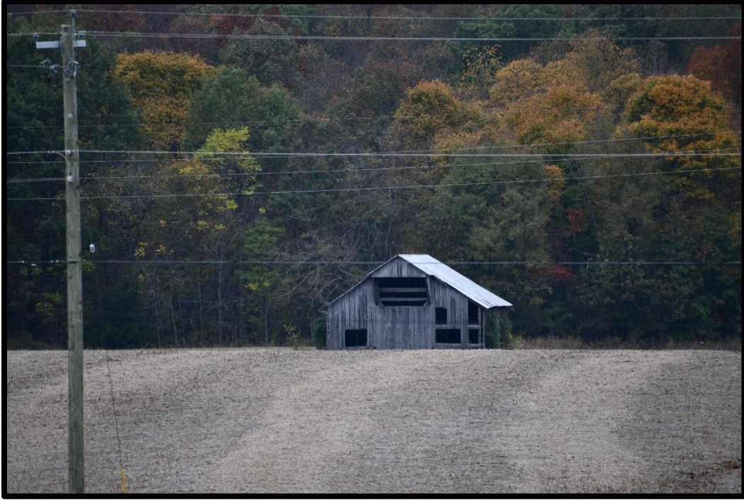
Plate 153. CA-451, Barn, southwest elevation, looking northeast.
