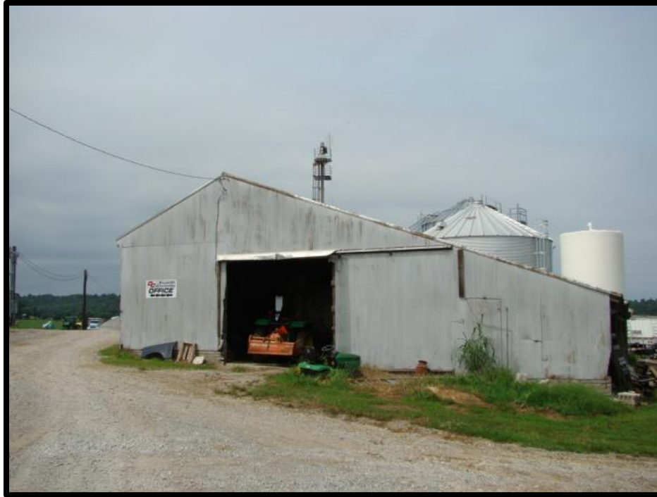
Plate 144. CA-449E, Barn/Workshop, southwest (front) elevation, looking north (Caldwell PVA).
