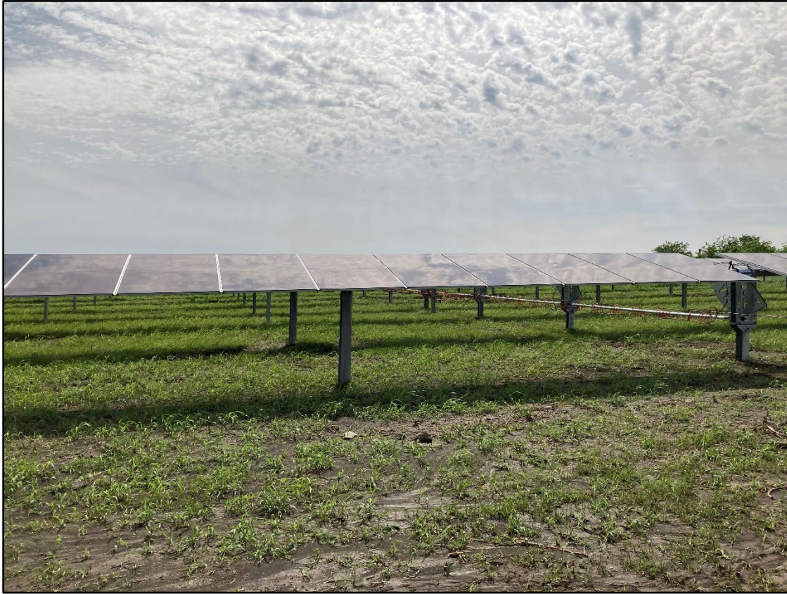
Figure 1 Tracking Rack System
