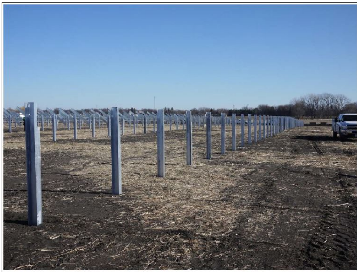
Figure 5 Standard Steel Pier Foundations
