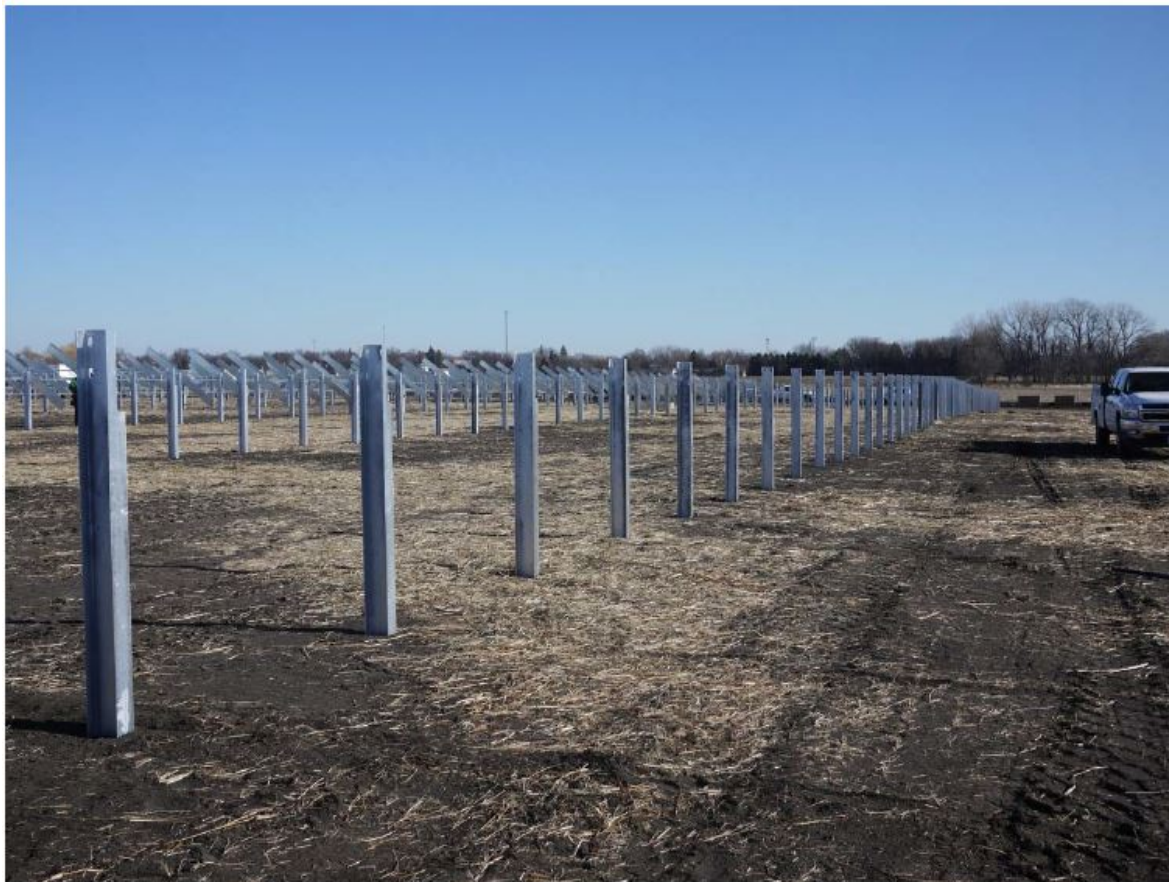
Figure 3 Standard Steel Pier Foundations
