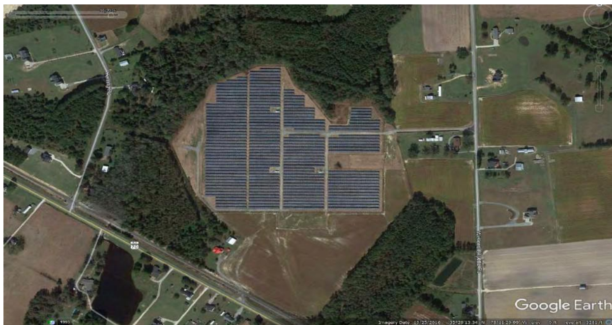
This 5 MW solar farm is located at 4839 US 70 Highway just east of Herring Road. This solar farm was completed on October 25, 2016.
