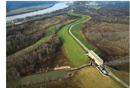
Flood Protection Pumps and Levees
