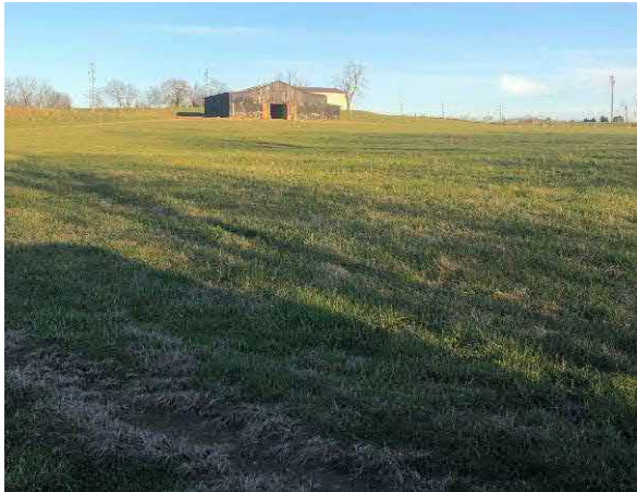
Photo #1 View of southwest portion of site northeast of Radio Station Road – barn and shed in DND area.
