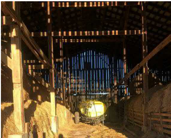
Photo #3 View of southwest portion of site – barn interior.
