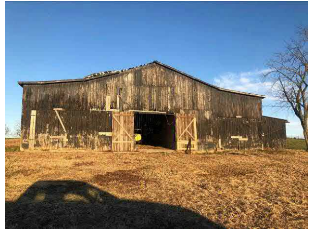
Photo #2 View of barn on southwest portion of site.
