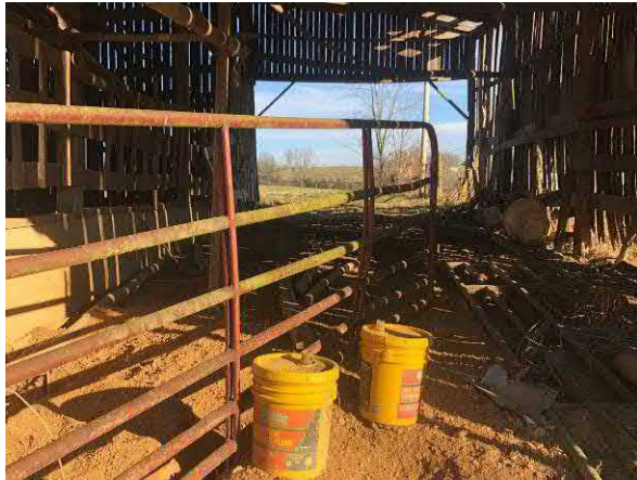
Photo #3 View of northwest portion of site – barn interior.
