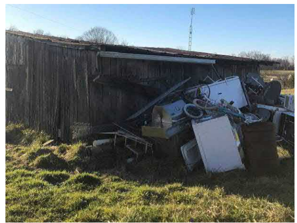
Photo #12 View of northwest portion of site – shed and debris.
