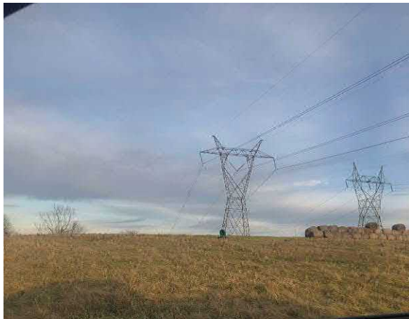
Photo #19 View of northwest portion of site.
