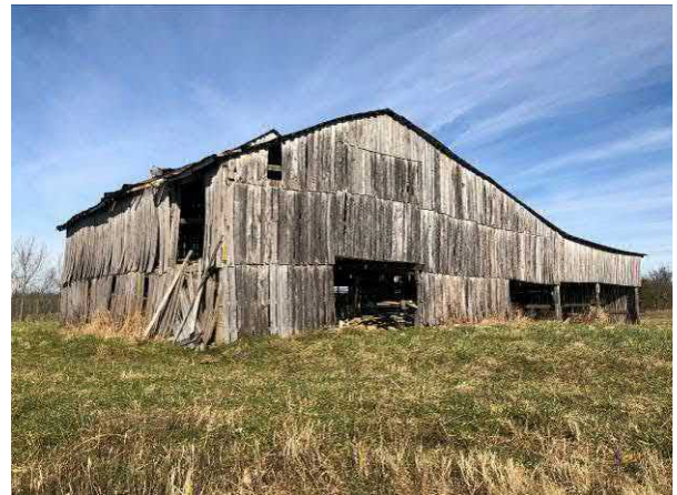
Photo #2 View of south-central portion of site – barn.
