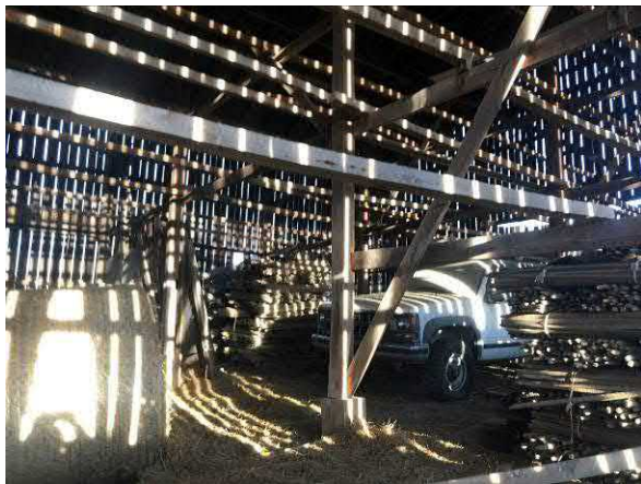
Photo #17 View of northwest portion of site – barn interior.
