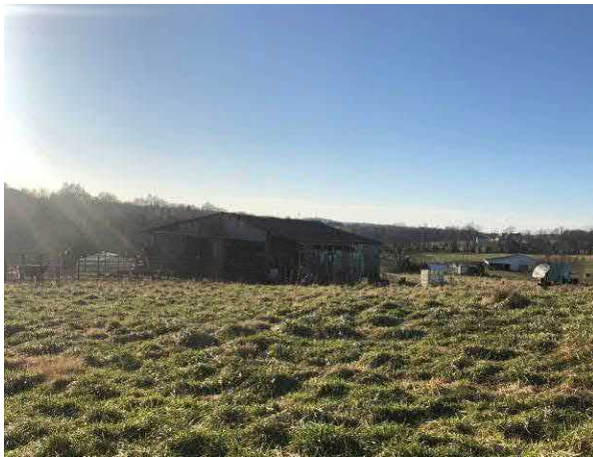
Photo #15 View of northwest portion of site – barn, tote, and debris.
