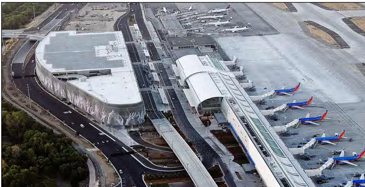
Figure 21: Solar on New Rental Car Parking Facility at Mineta San Jose Airport
