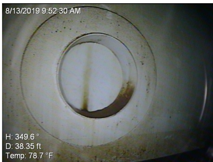
29) The sidewall hatch is in good condition.
