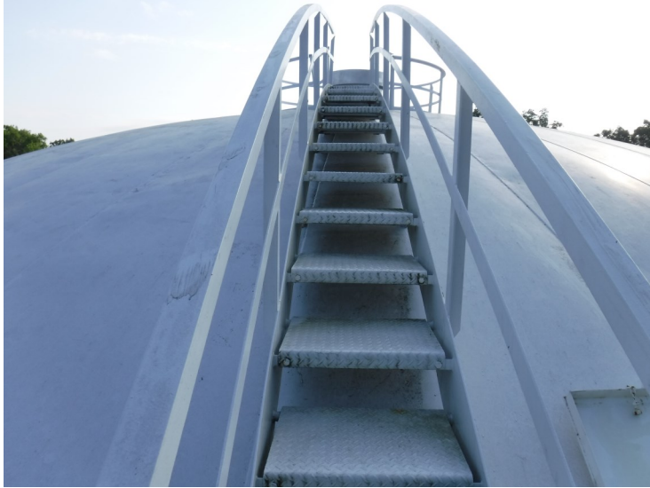
10) Handrail and stairs leading to the center of the roof.
