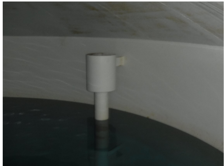
23) The overflow weir is in good condition.
