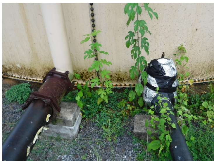
3) The drain line and overflow pipe are in good condition.
