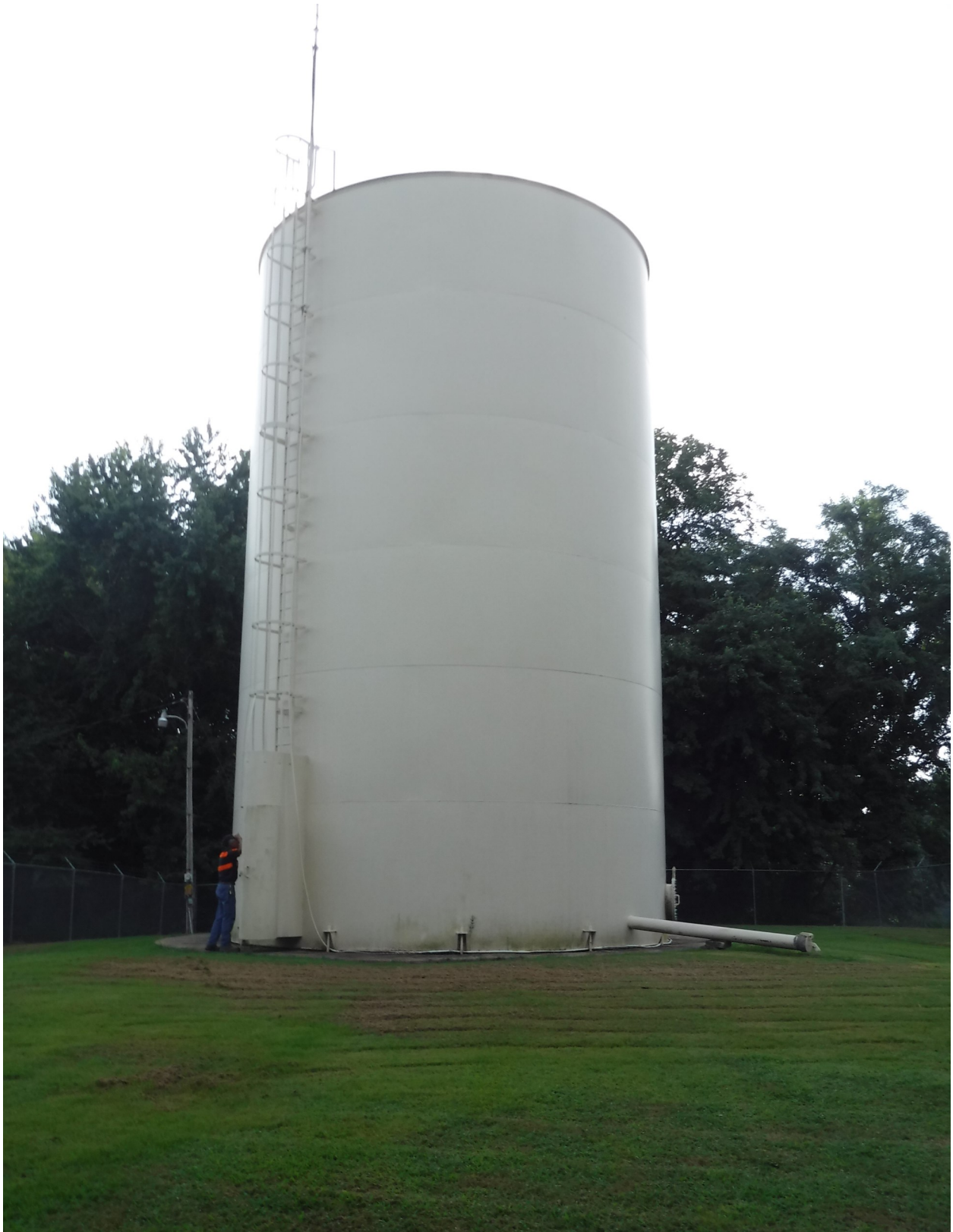
200,000 gallon standpipe located in Clinton, Kentucky and owned by Water Service Corporation of Kentucky.
