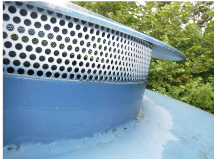
11) The flow through vent screen is in good condition.
