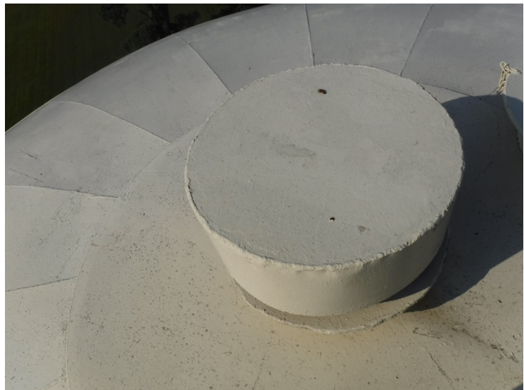
14) The flow-through roof vent is in good condition.
