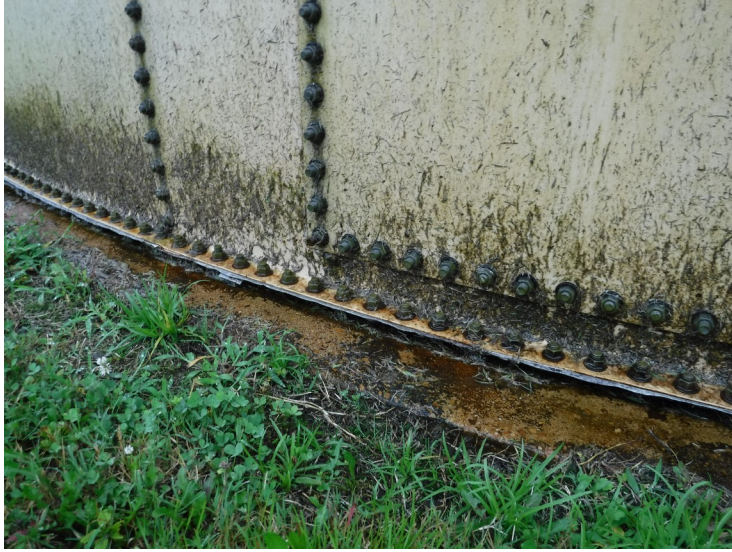
1) The exposed foundation is in good condition.
