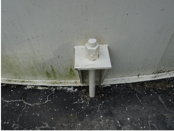
4) Typical anchor bolt is in good condition.
