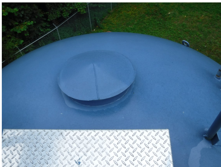
12) The roof coating is in good condition.
