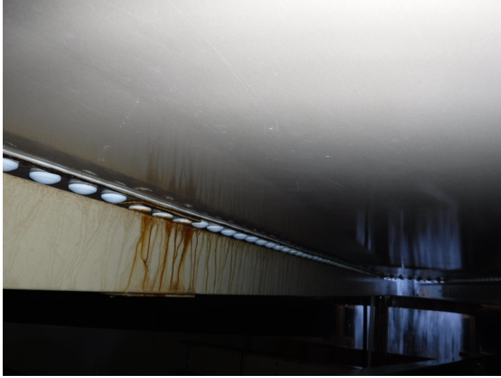
16) The roof lining is in good condition overall.
