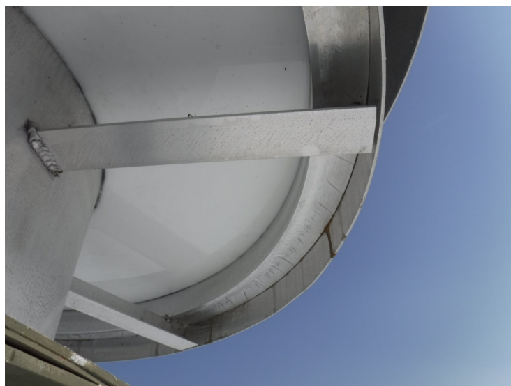
12) The vent pressure plate is aligned.
