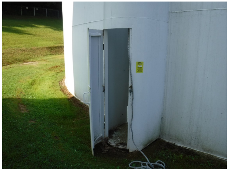
8) The vandal guard is in good condition.
