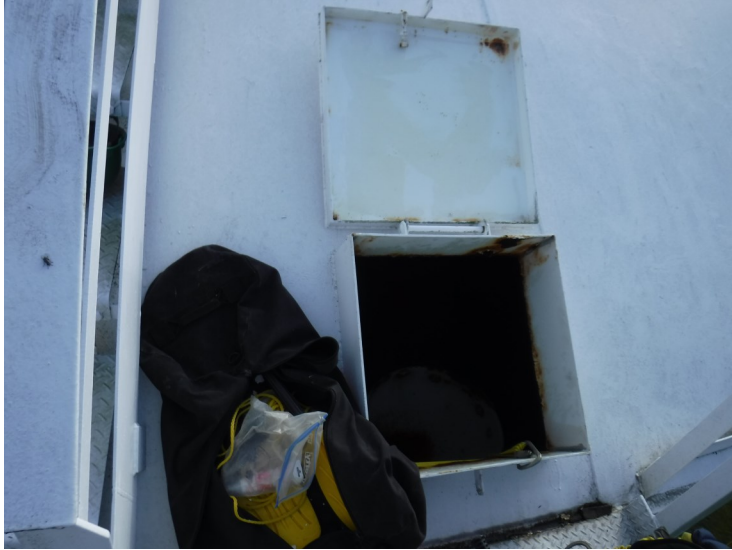
16) The wet interior hatch is in good condition.
