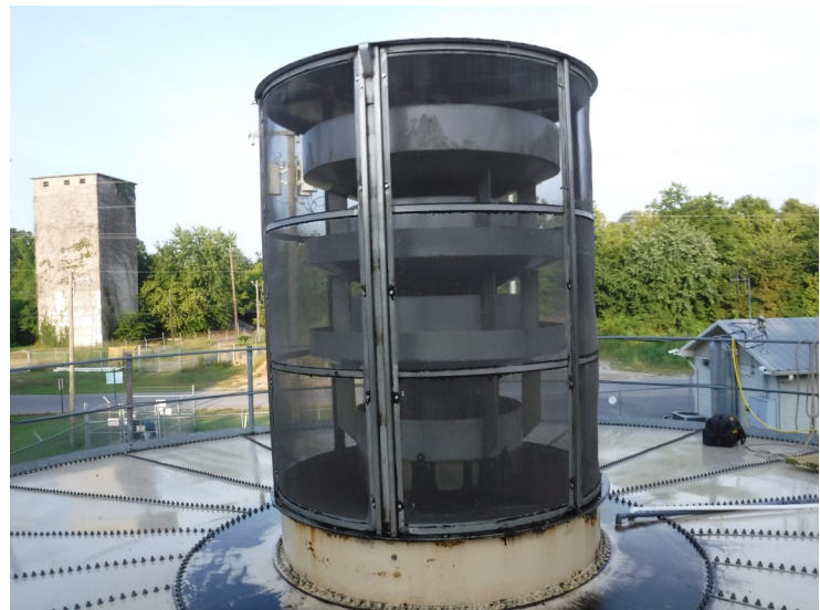
11) The aerator vent is in good condition.
