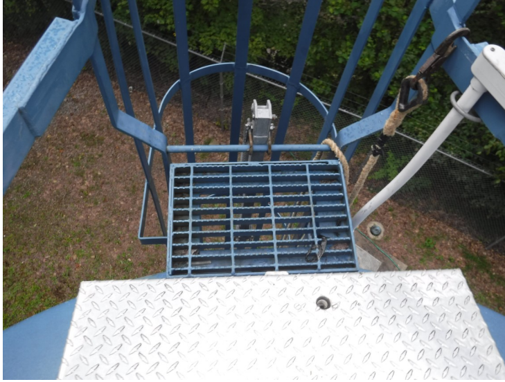
10) The ladder step-off platform is in good condition.
