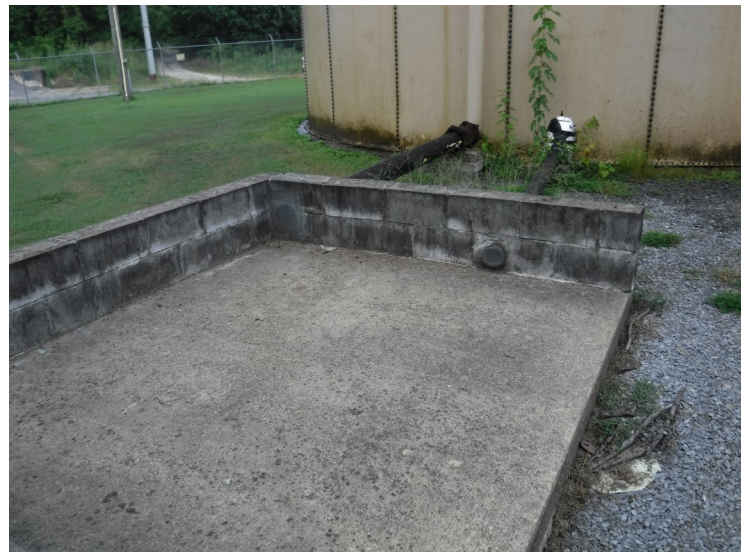
5) The overflow splash pad is in good condition.
