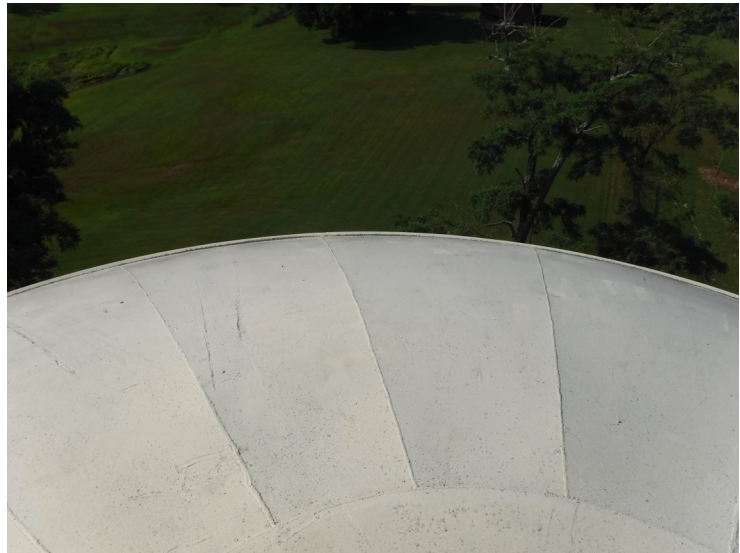
17) The roof coating is in good condition overall.
