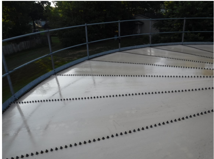
14) The roof lining is in good condition overall.
