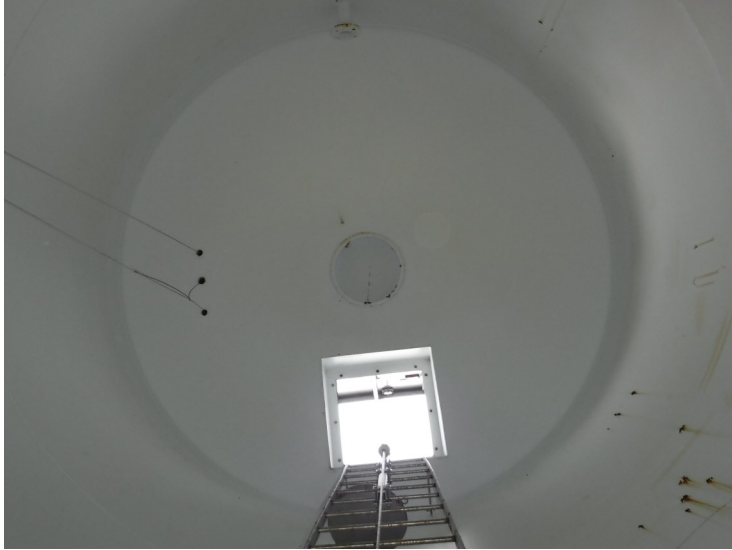
16) The wet interior roof coating is in good condition overall.
