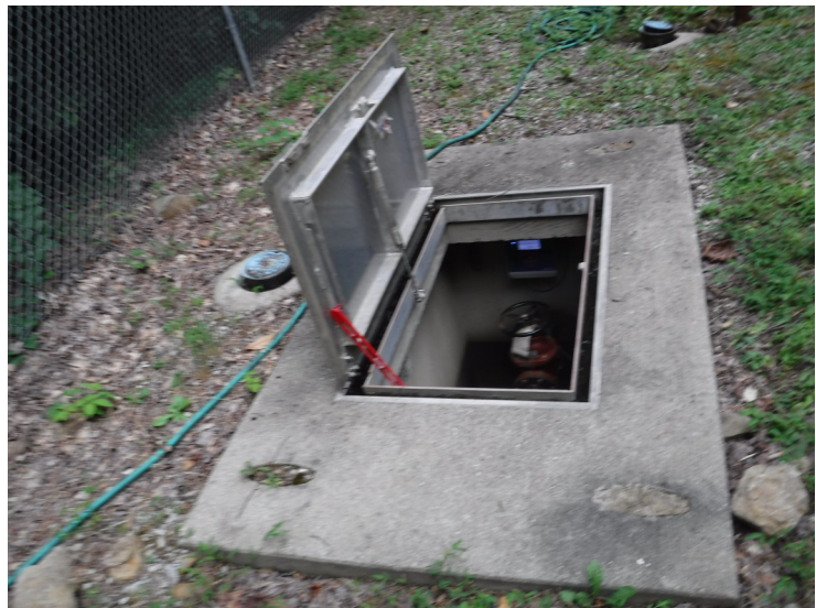
26) The metal cover for the pit piping is in good condition.
