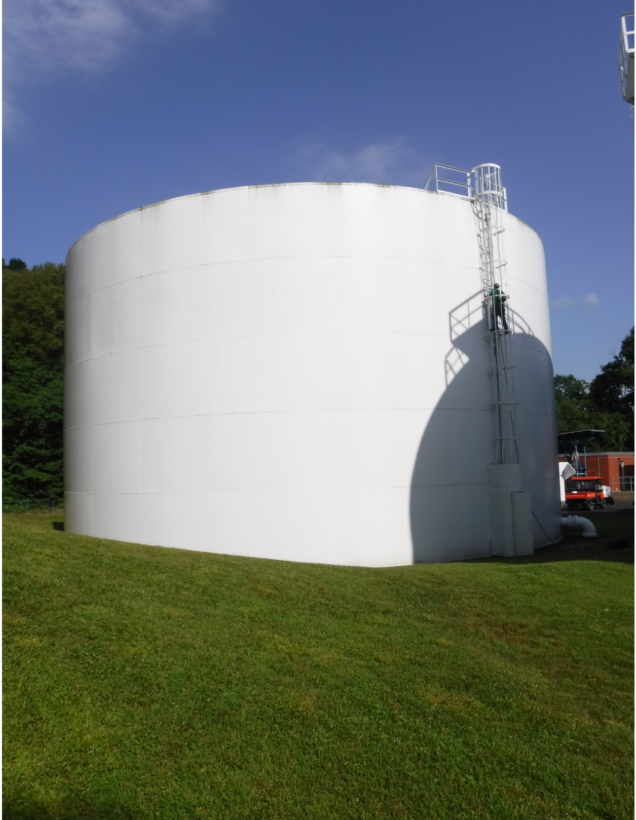
1,250,000 gallon ground storage tank #2 owned by Water Service Corporation of Kentucky in Middlesboro, Kentucky.
