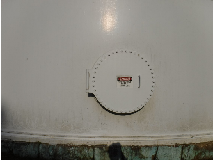
4) The sidewall manway is in good condition.
