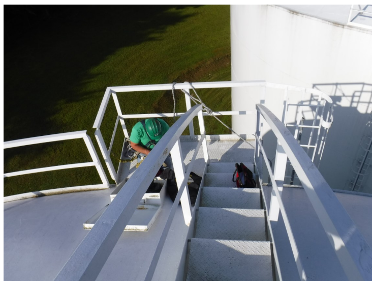
9) Step-off platform at the top of the sidewall.
