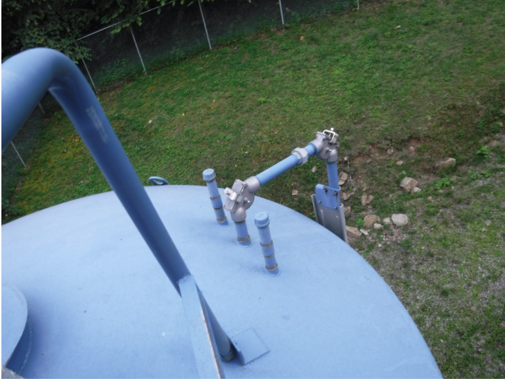
13) The roof penetrations for the level indicator are in good condition.
