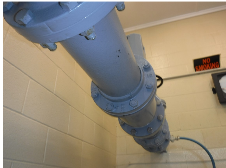
29) The coating on the piping is in good condition.
