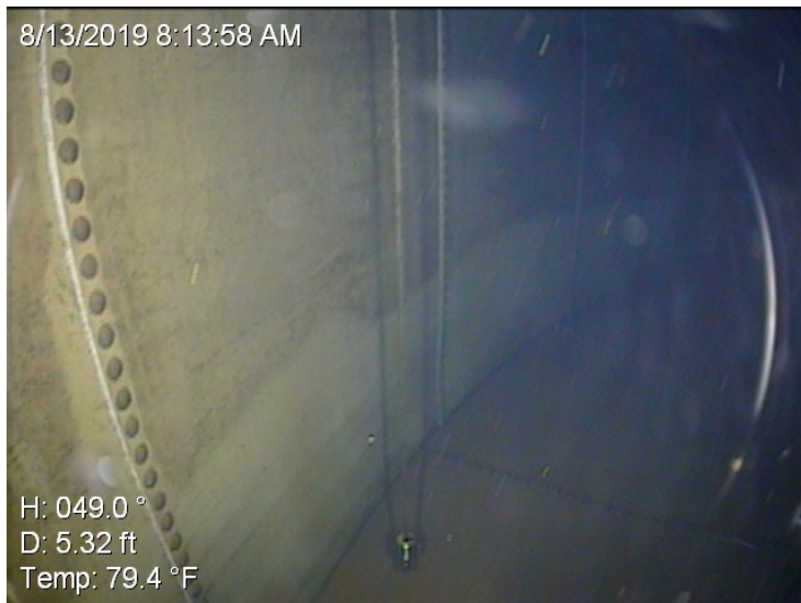
19) The sidewall lining is in good condition overall.
