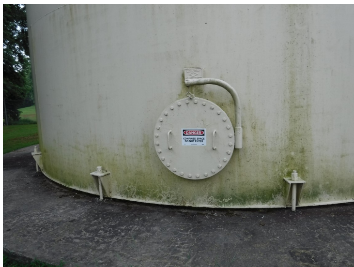
9) Typical sidewall manway is in good condition.
