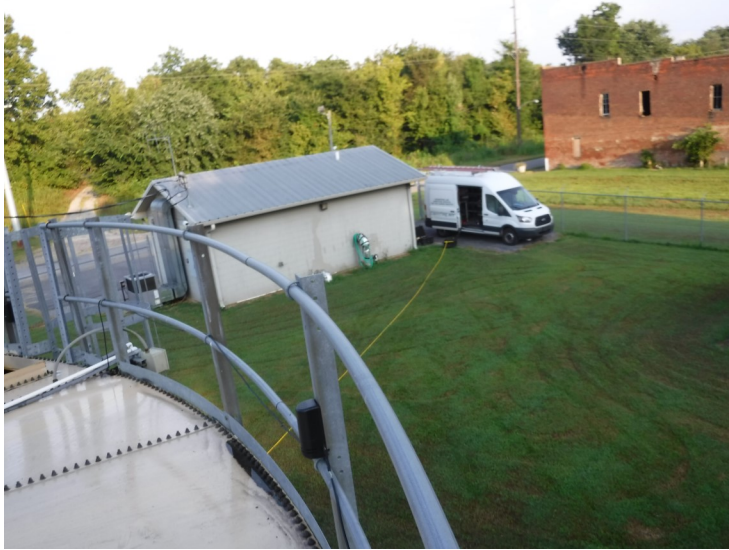
10) The roof handrail is in good condition.
