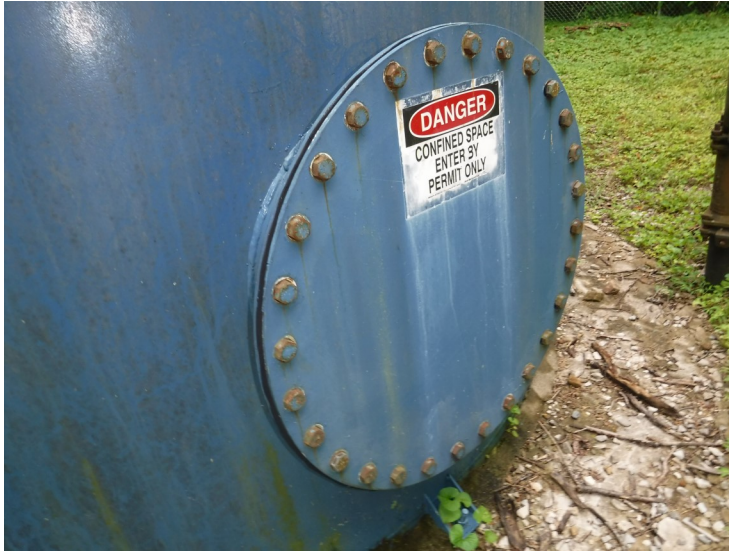
4) The sidewall manway is in good condition.
