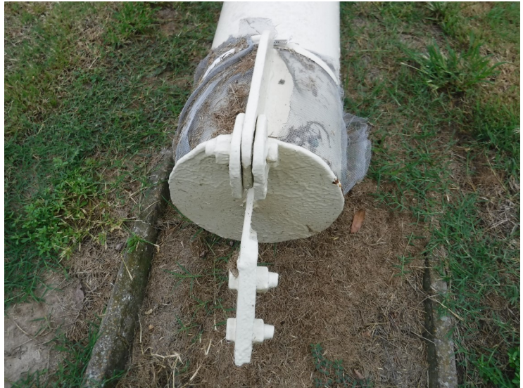
5) The overflow flap gate is in good condition.
