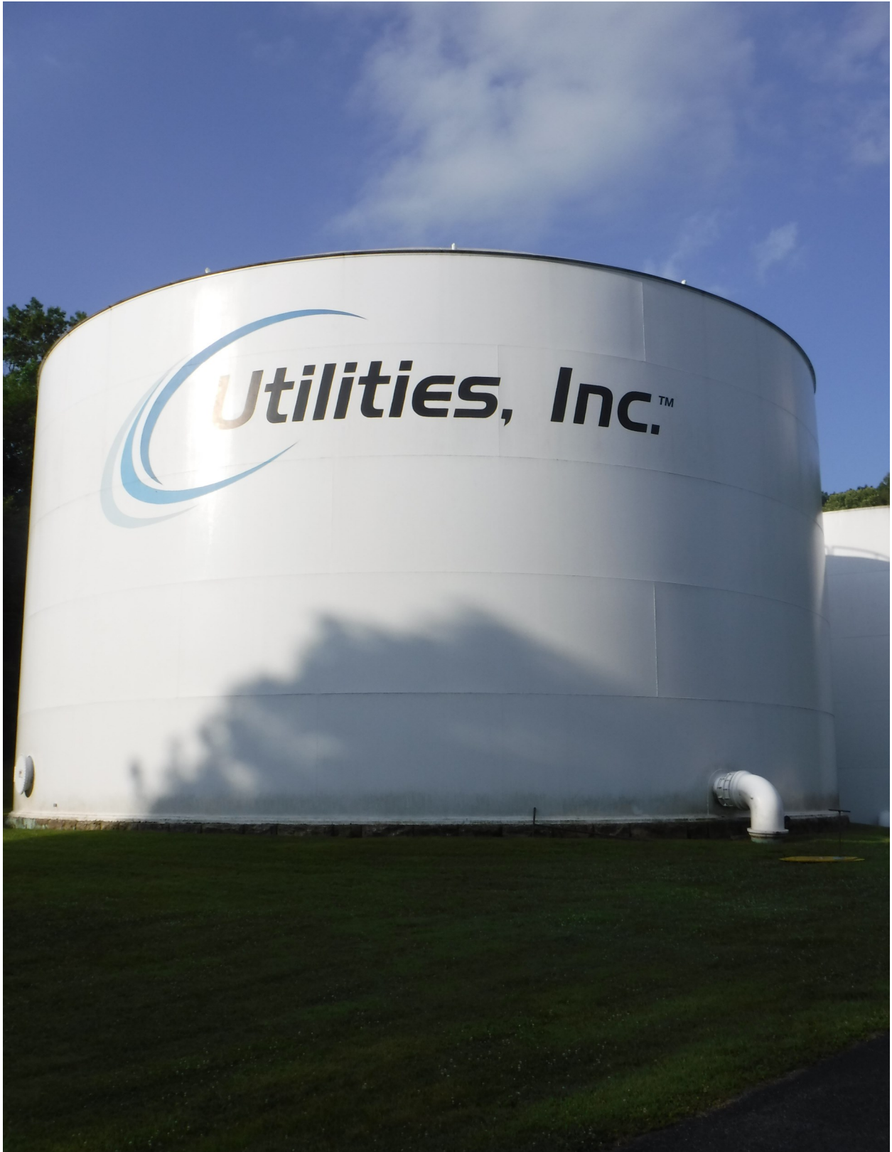
1,250,000 gallon ground storage tank #1 owned by Water Service Corporation of Kentucky located in Middlesboro, Kentucky.
