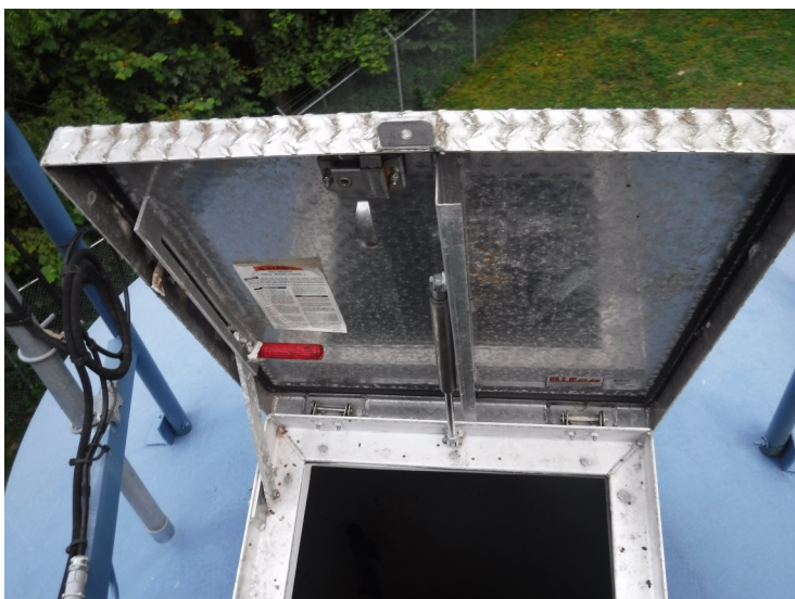
15) The hatch cover operated properly during the inspection.
