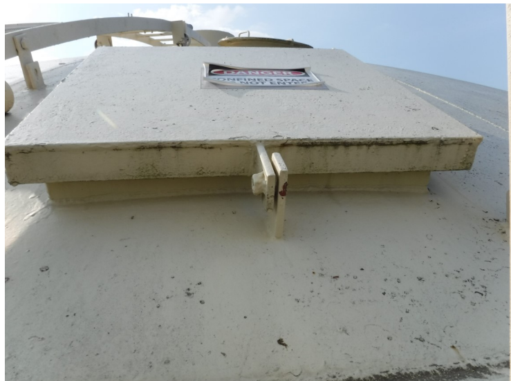
20) The wet interior roof hatch is in good condition.
