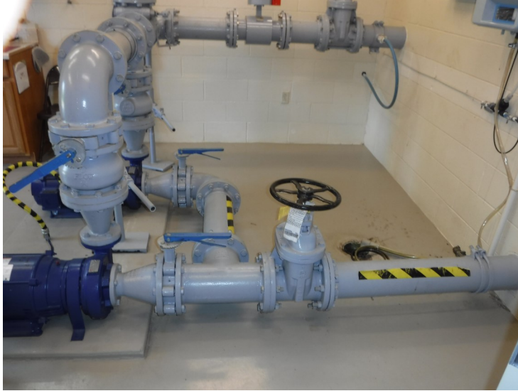
28) There is a pumphouse adjacent to the tank with piping.
