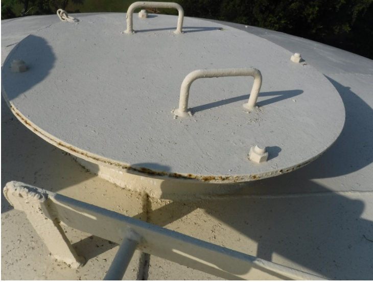
16) The bolted ventilation hatch is in good condition.
