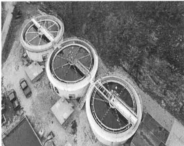
Drone View Water Plant Clarifiers
