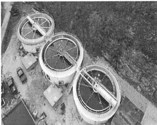
Drone View Water Plant Clarifiers
