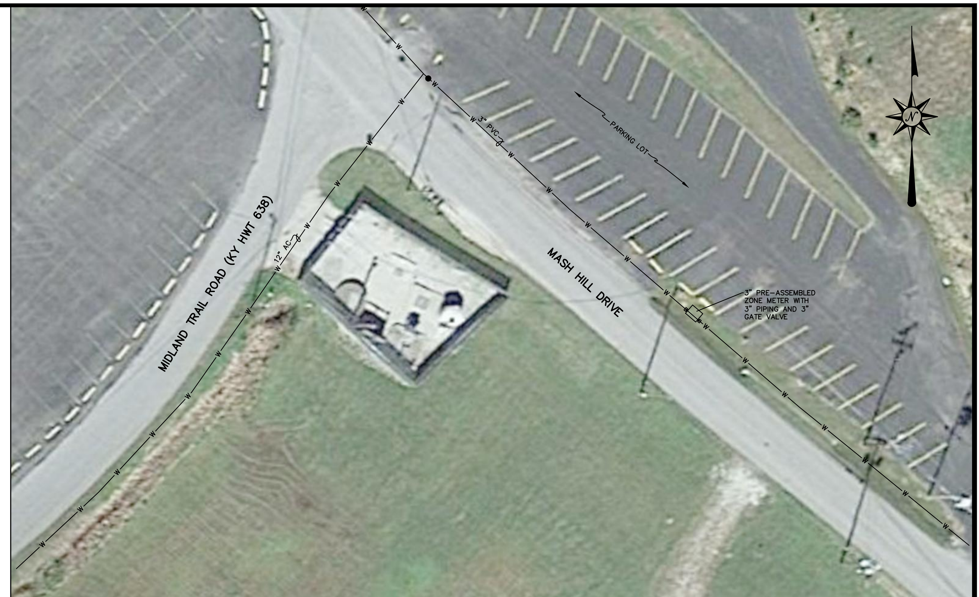
MIDLAND TRAIL ROAD (KY HWY 638) AT MASH HILL DRIVE
