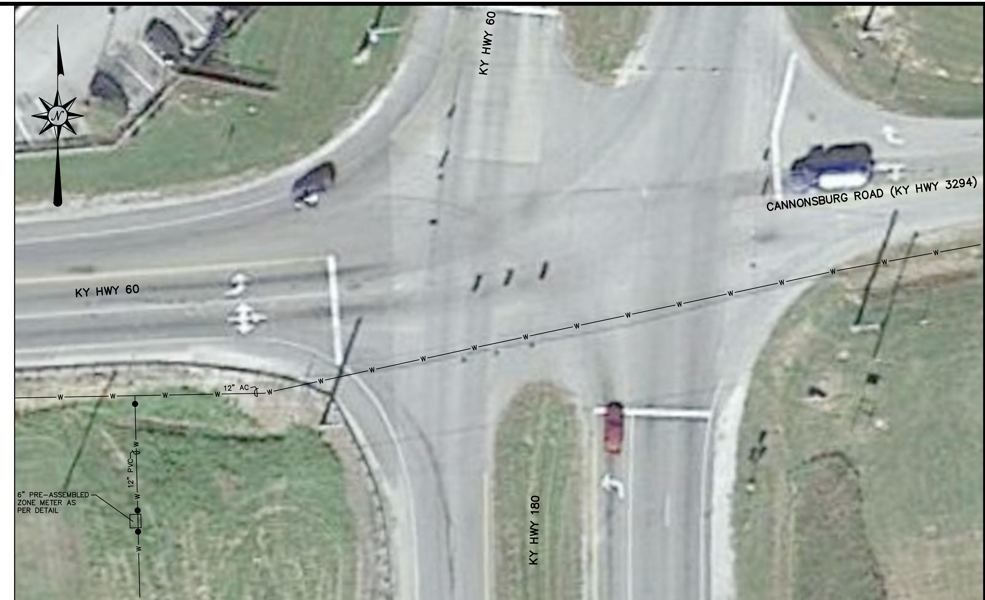
KY HWY 60 AT KY HWY 180 AT CANNONSBURG ROAD (KY HWY 3294)
