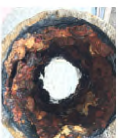
6" unlined cast iron pipe
