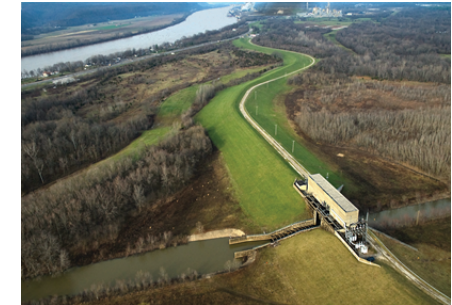
Flood Protection Pumps and Levees
