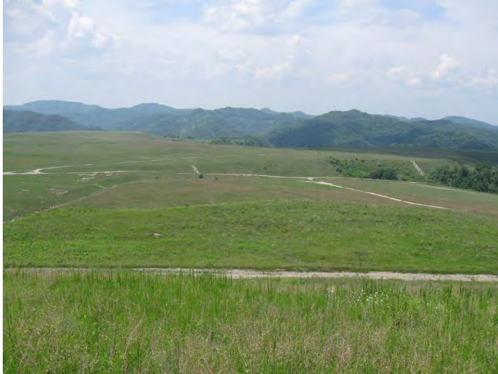
Photo No. 2 Center view of sector #2 looking towards Long Branch (upper reach)
