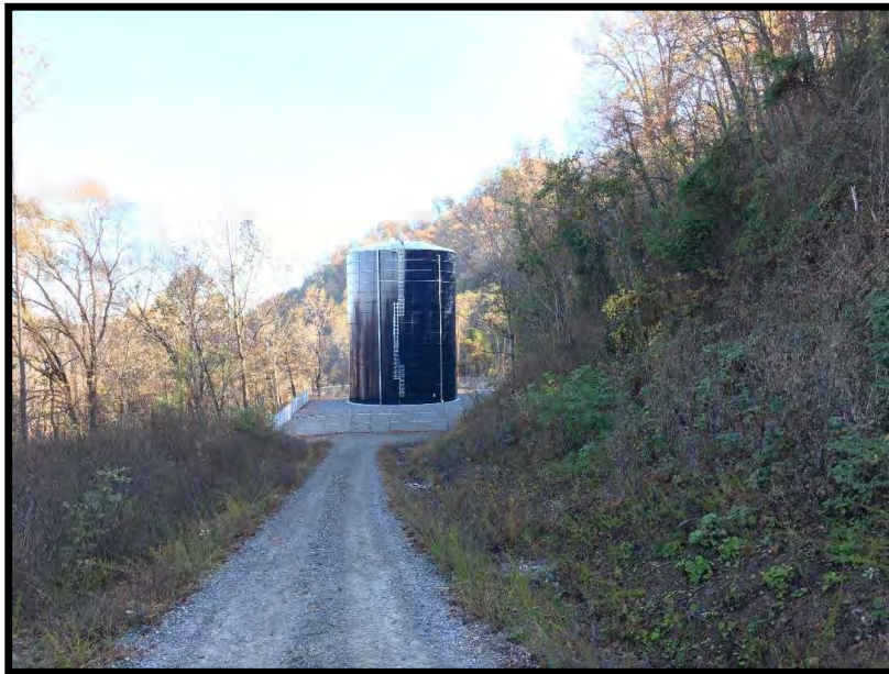
Photo #8 View of water tank located on southern portion of property.
