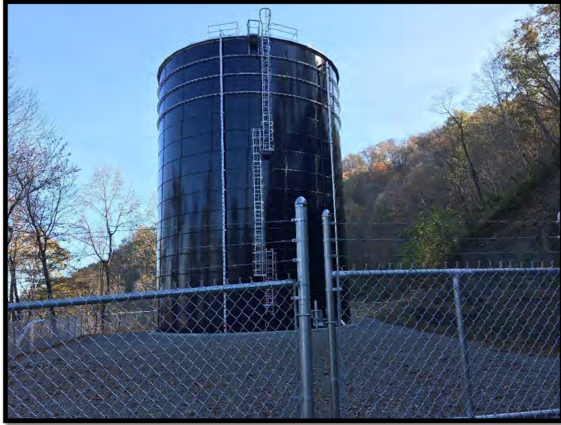
Photo #9 View of water tank.
