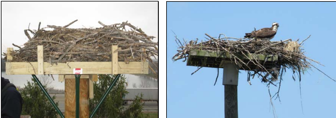
Figure 9.2 – Platforms on a Dummy Pole for Osprey Nests
