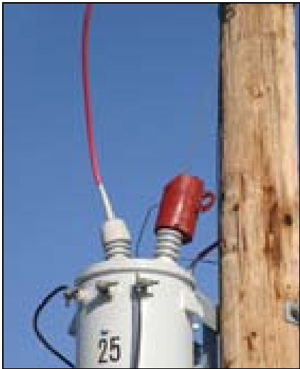
Figure 11.8 Bushing and Jumper Covers
