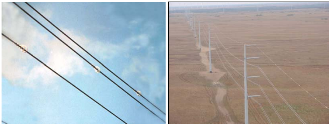
Figure 11.3 Bird/Swan Flight Diverters, installed
