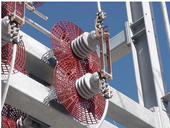
Figure 11.13 Barriers between phase and ground
