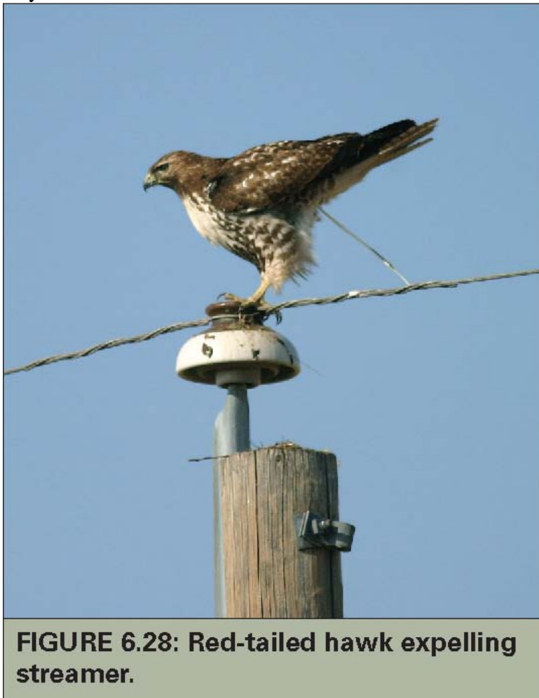
Figure 7.3 Streamer (contamination build-up)
