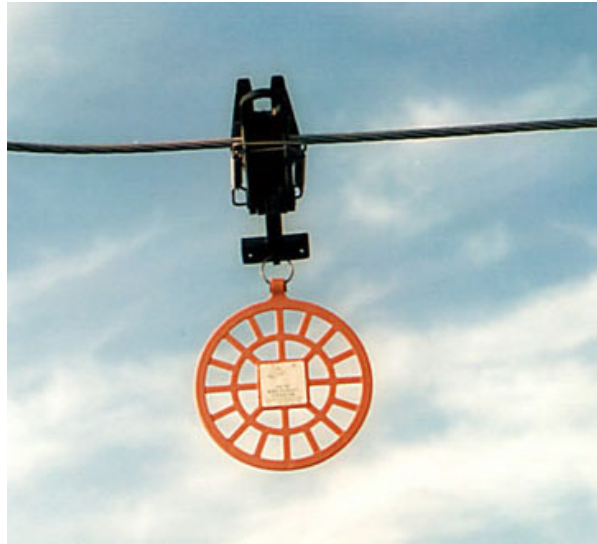
Figure 11.5 Waffle-design Flapper
