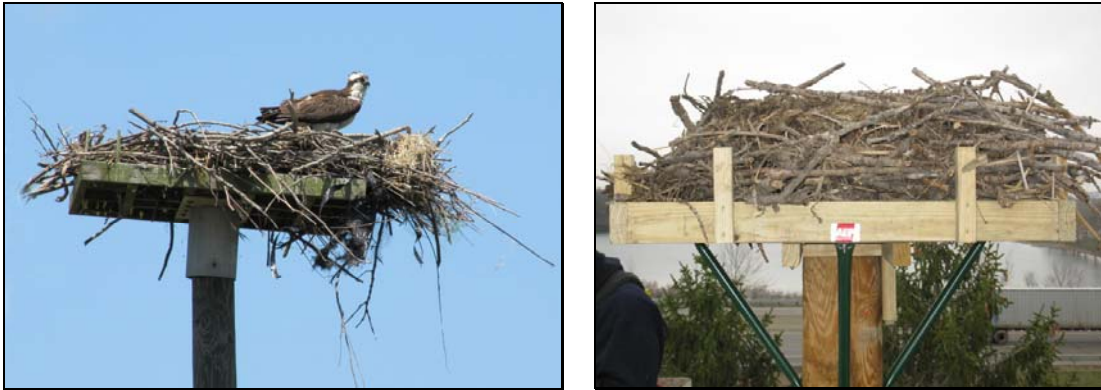
Figure 11.17 Nest platforms on dummy poles.
