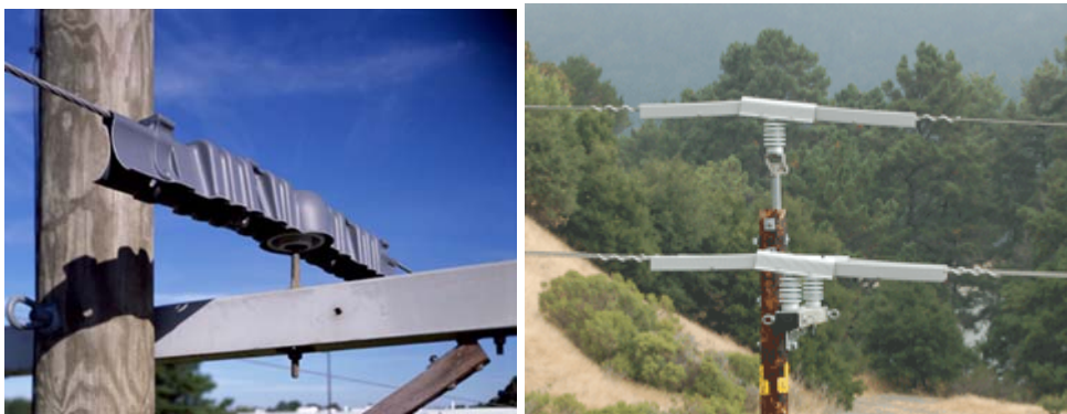
Figure 11.11 Insulator and Conductor Covers (Tyco/Eco)
