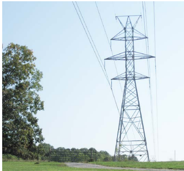
Figure 2. Proposed Typical Structure (Steel Lattice Tower)
