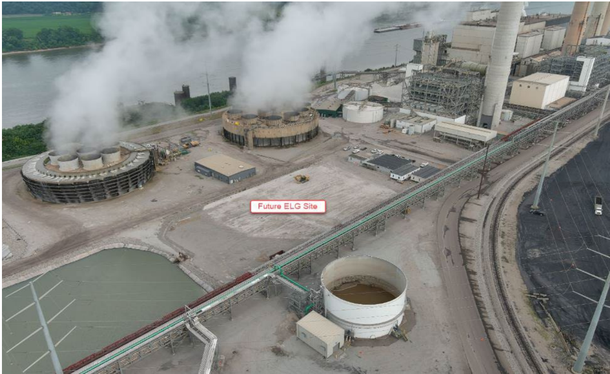
Mill Creek – ELG Water Treatment Future Location – July 2022
