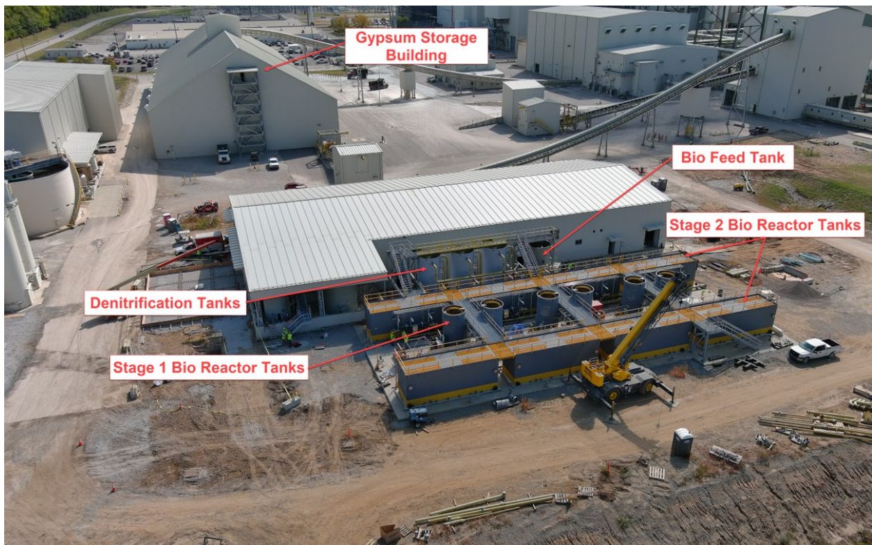
Trimble County – ELG Water Treatment Location – October 2022
