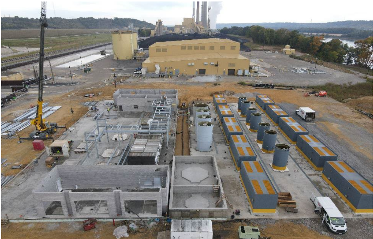
Ghent – ELG Water Treatment Future Location – October 2022
