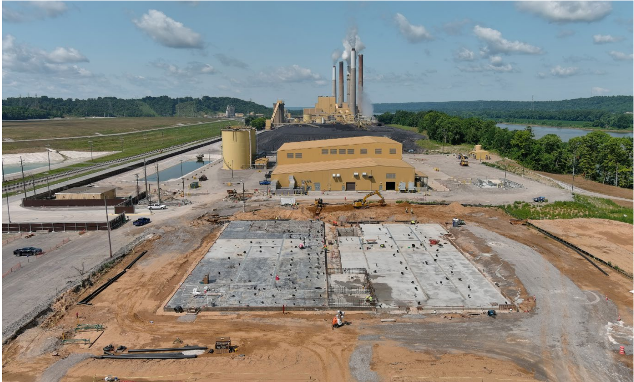
Ghent – ELG Water Treatment Future Location – July 2022
