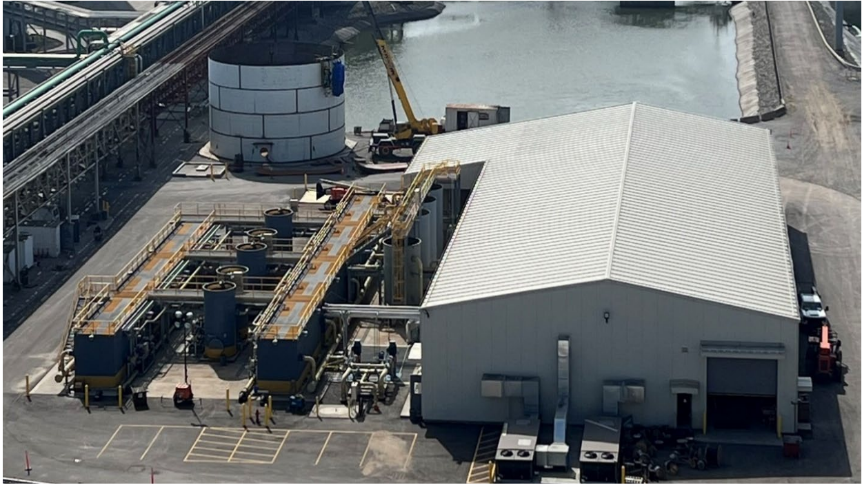
Mill Creek – ELG Water Treatment – June 2023
