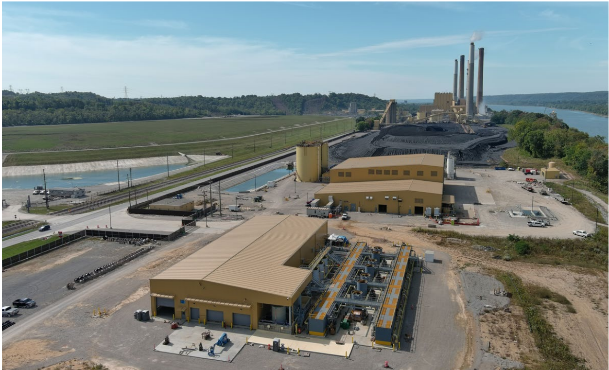
Ghent – ELG Water Treatment – October 2023
