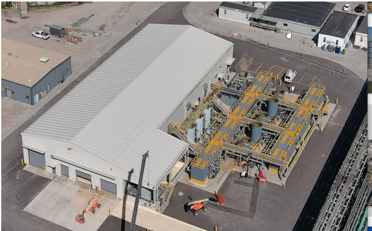
Mill Creek – ELG Water Treatment – October 2023
