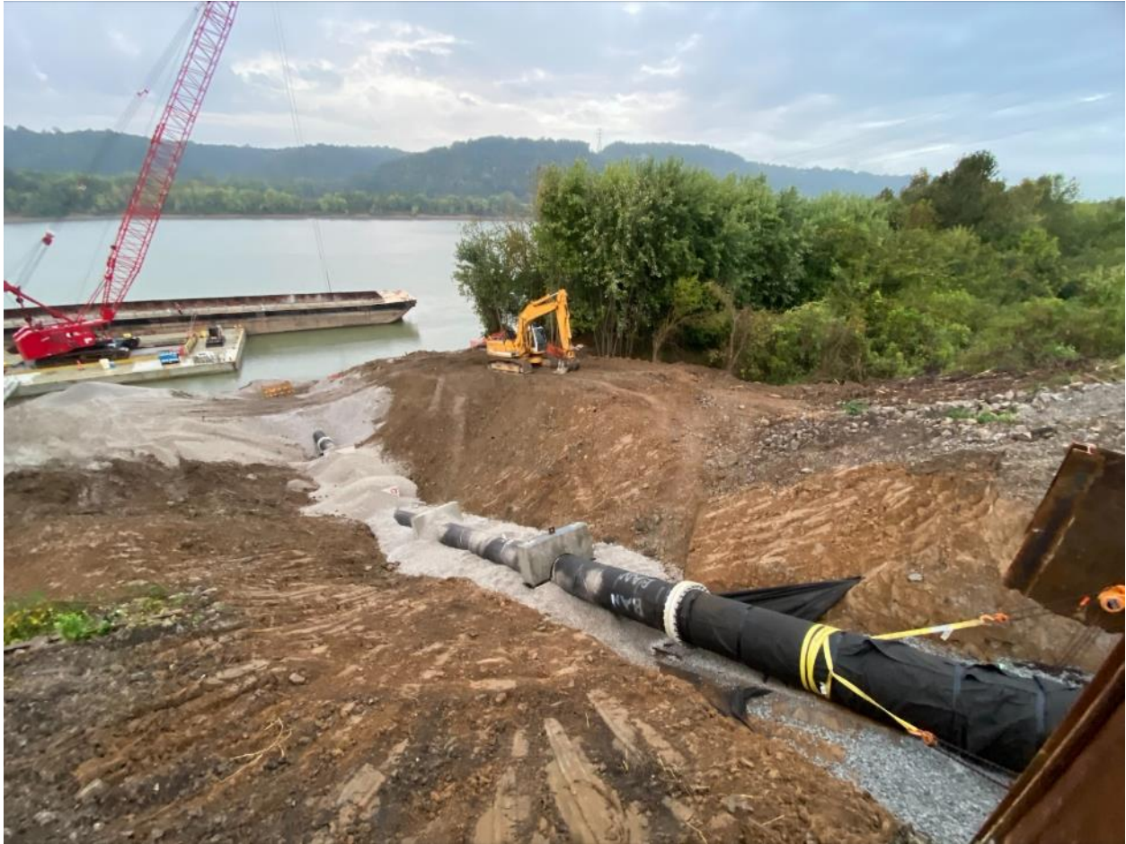
Mill Creek – North Diffuser – October 2021
