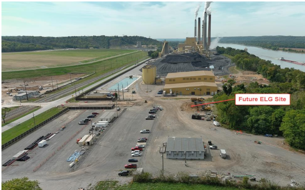
Ghent – ELG Water Treatment Future Location – September 2021
