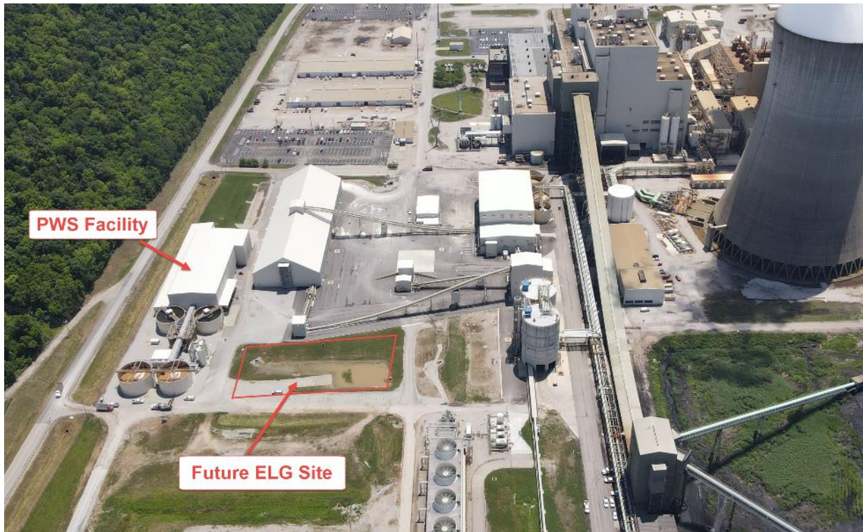
Trimble County – ELG Water Treatment Future Location – July 2021
