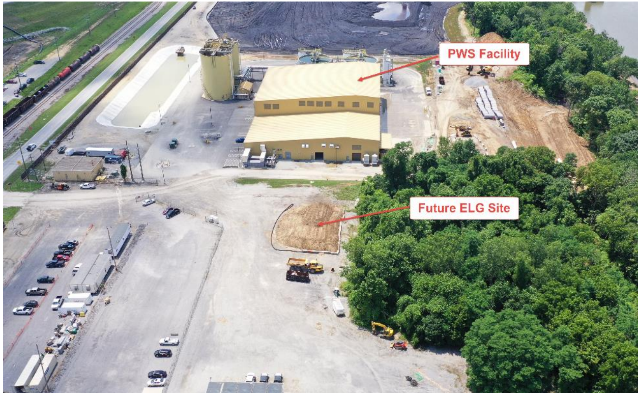
Ghent – ELG Water Treatment Future Location – July 2021
