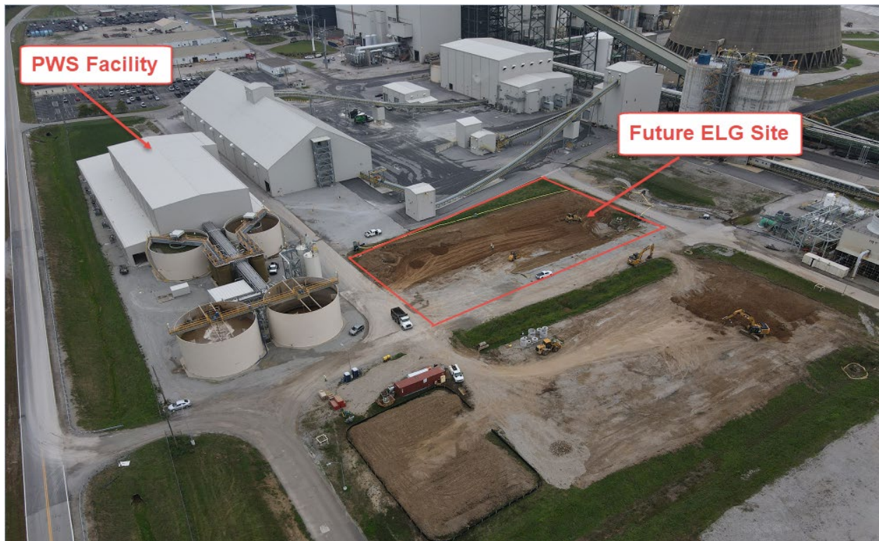
Trimble County – ELG Water Treatment Future Location – October 2021
