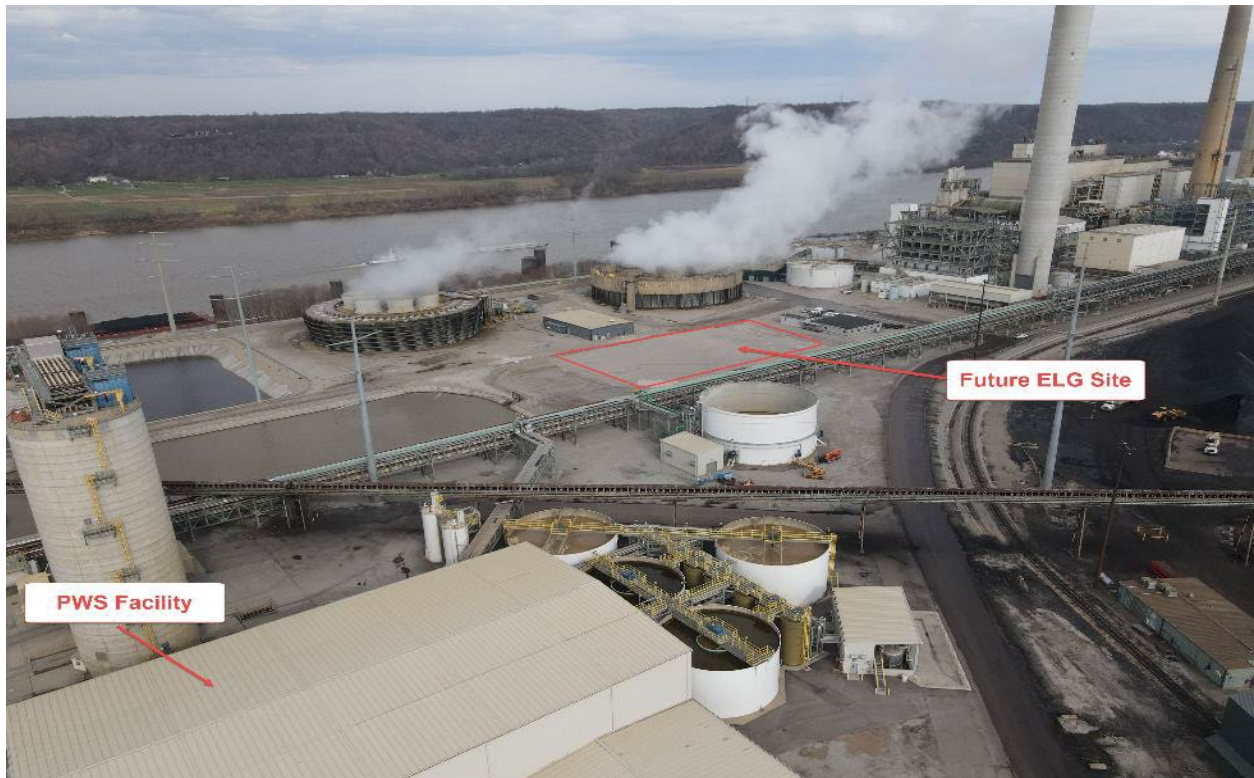
Mill Creek – ELG Water Treatment Future Location – March 2022
