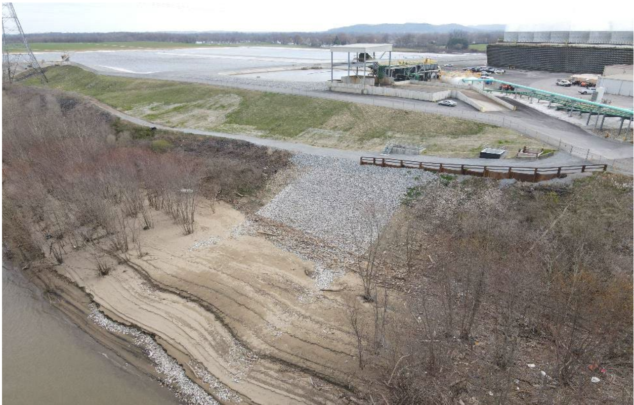
Mill Creek – North Diffuser – March 2022
