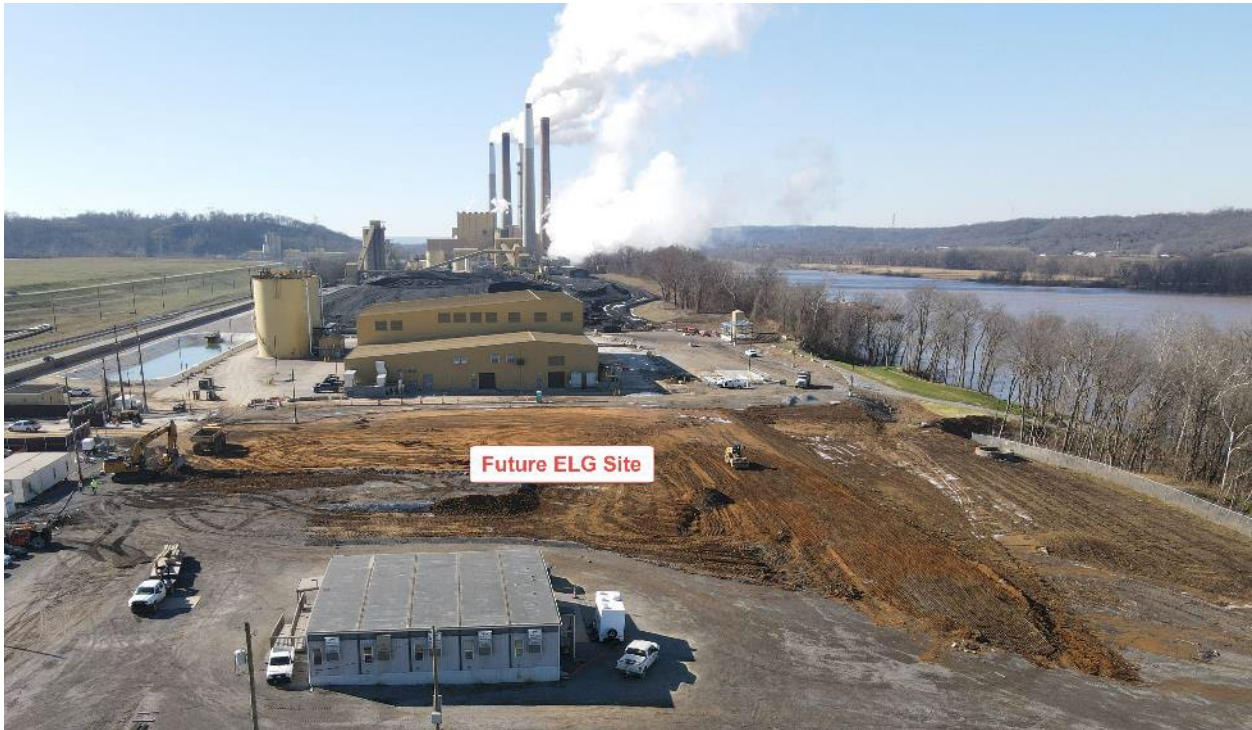
Ghent – ELG Water Treatment Future Location – January 2022
