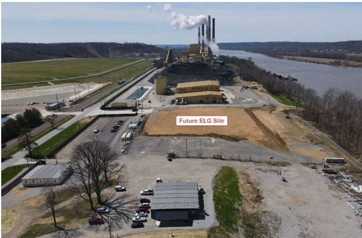
Ghent – ELG Water Treatment Future Location – March 2022
