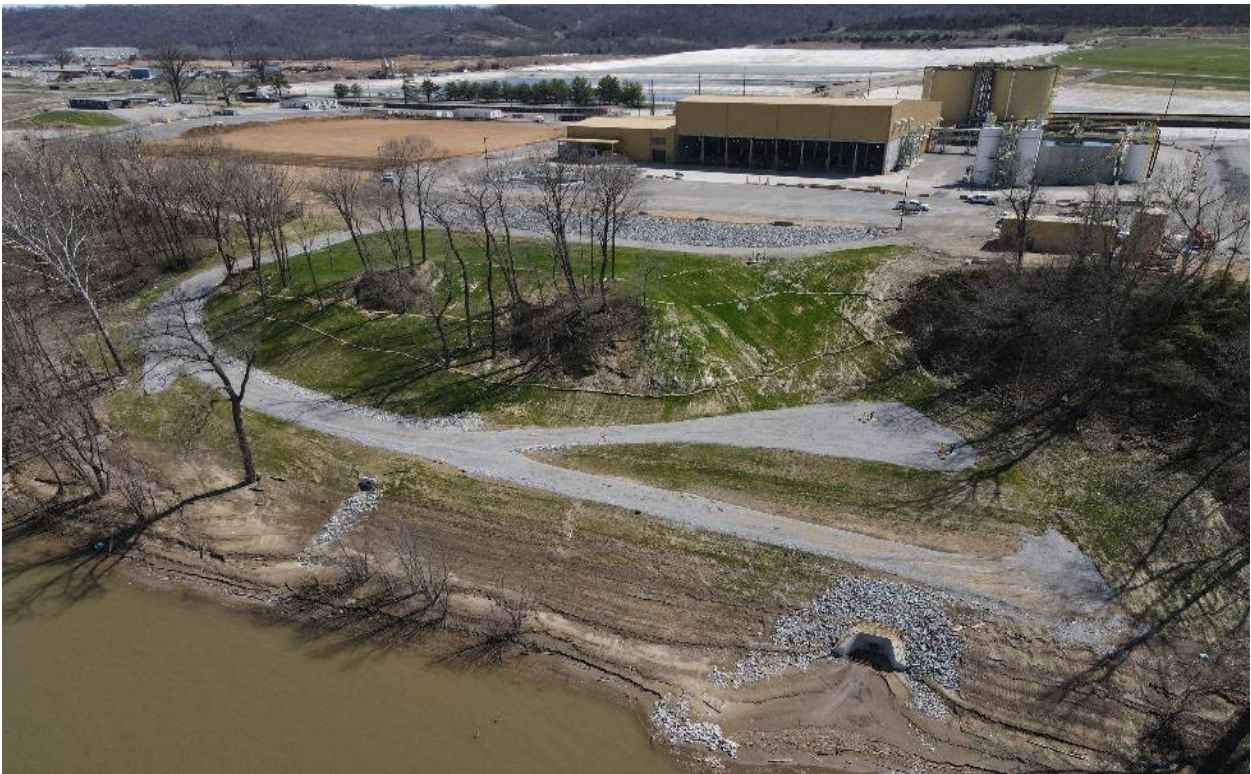
Ghent Outfall 001 Diffuser – Land Overview Looking Southeast – March 2022
