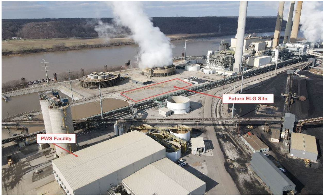
Mill Creek – ELG Water Treatment Future Location – January 2022
