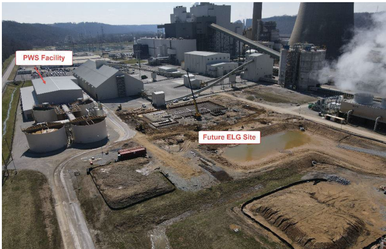
Trimble County – ELG Water Treatment Future Location – March 2022
