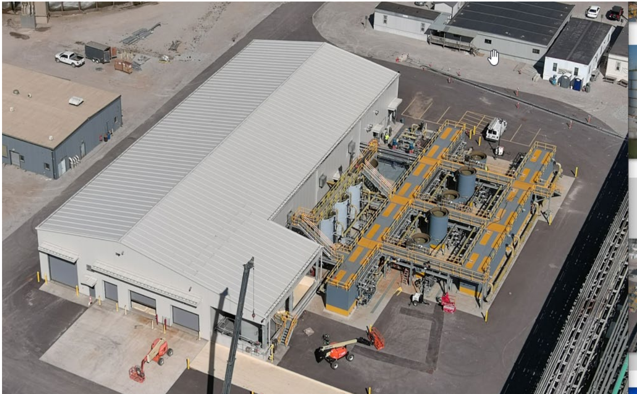
Mill Creek – ELG Water Treatment – October 2023
