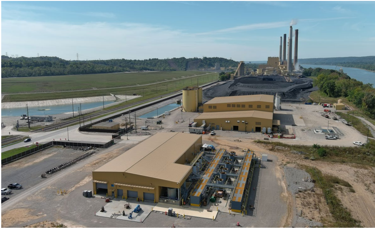
Ghent – ELG Water Treatment – October 2023
