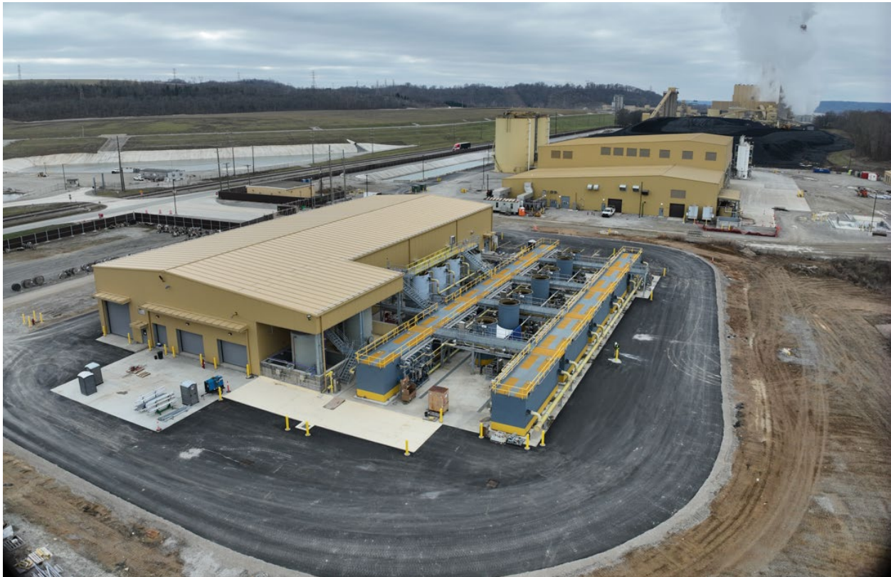
Ghent – ELG Water Treatment – December 2023
