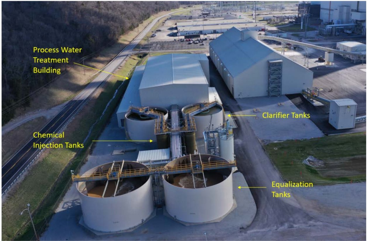
5 Trimble County Process Water Treatment System – External View
