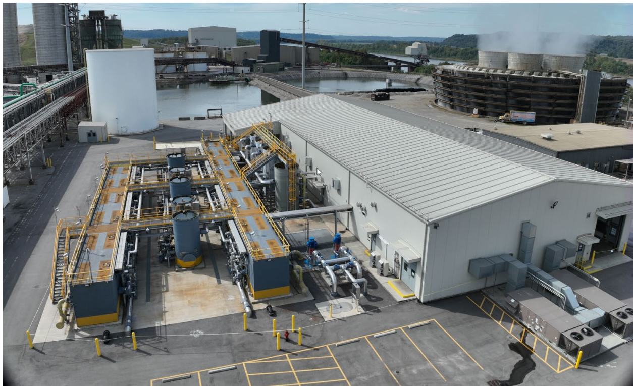
Mill Creek – ELG Water Treatment – September 2024
