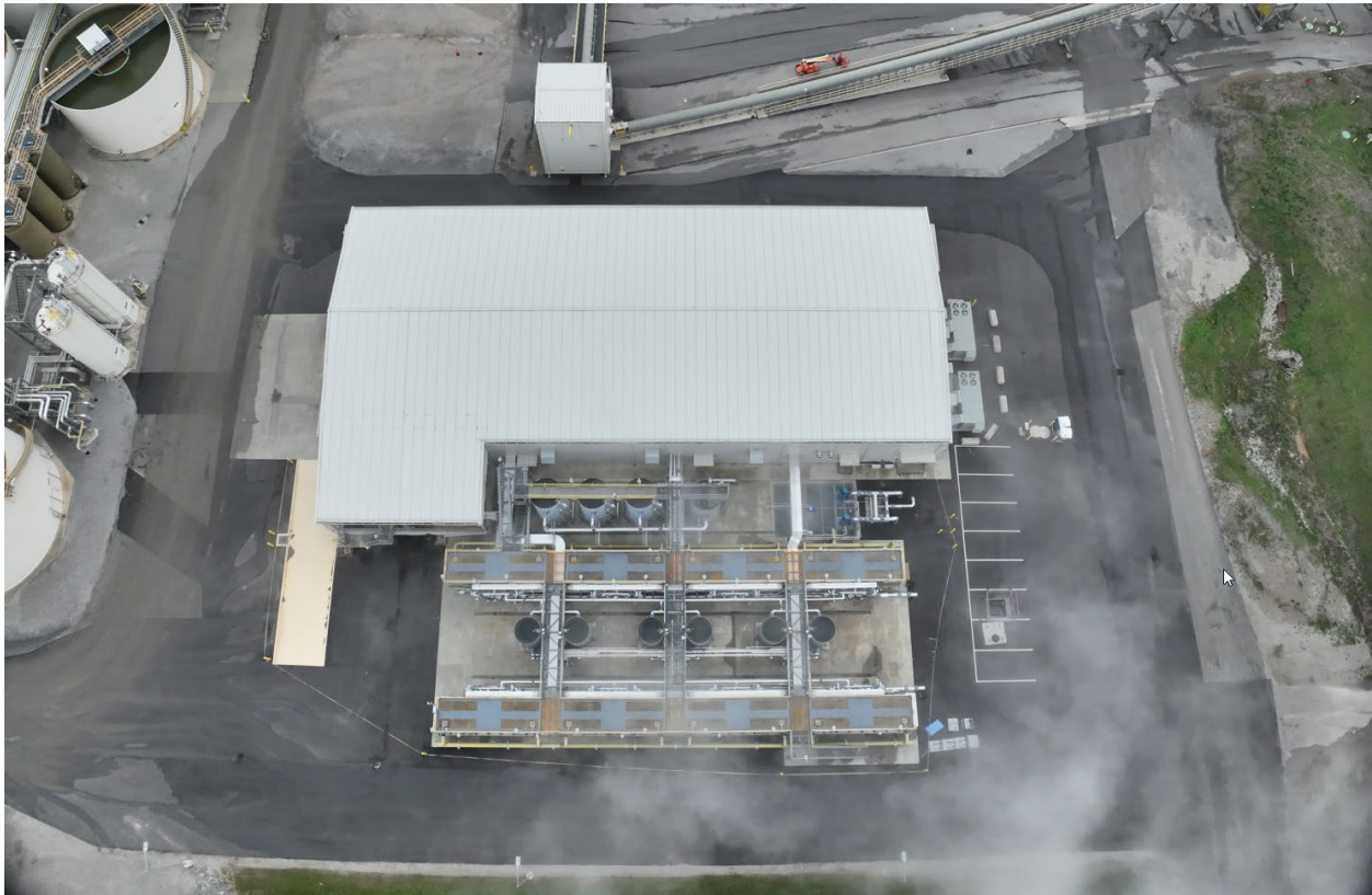
Trimble County – ELG Water Treatment Location – March 2024 – July 2024 No Changes
