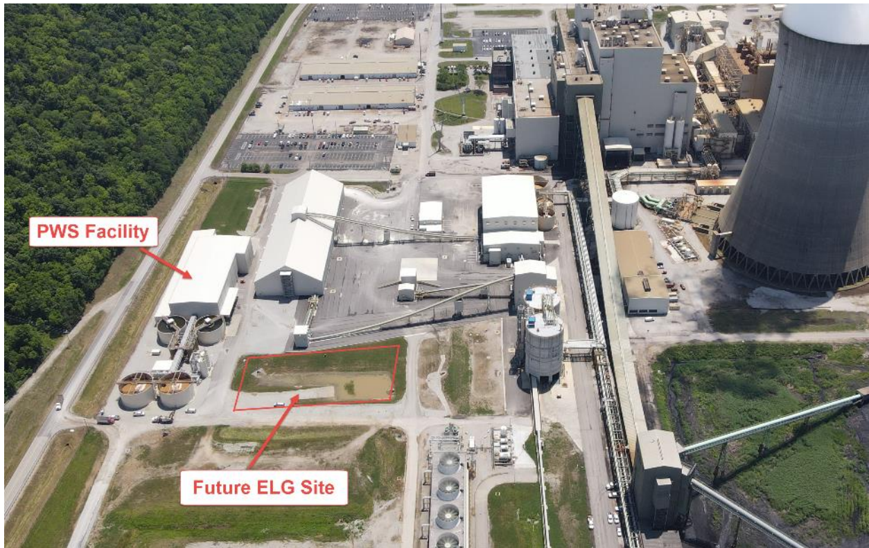
Trimble County – ELG Water Treatment Future Location – July 2021
