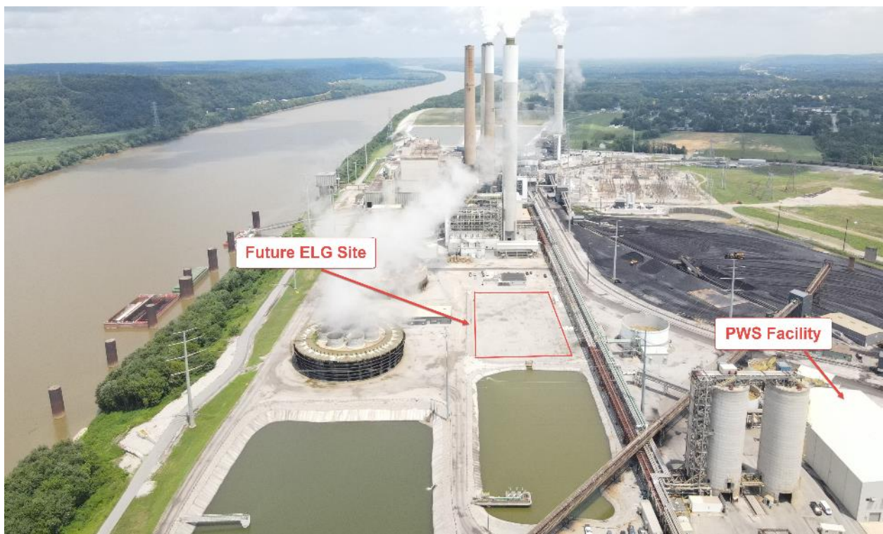
Mill Creek – ELG Water Treatment Future Location – July 2021
