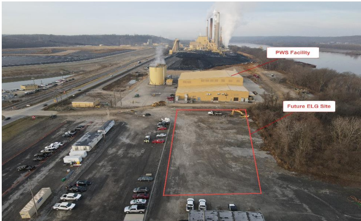
Ghent – ELG Water Treatment Future Location – March 2021
