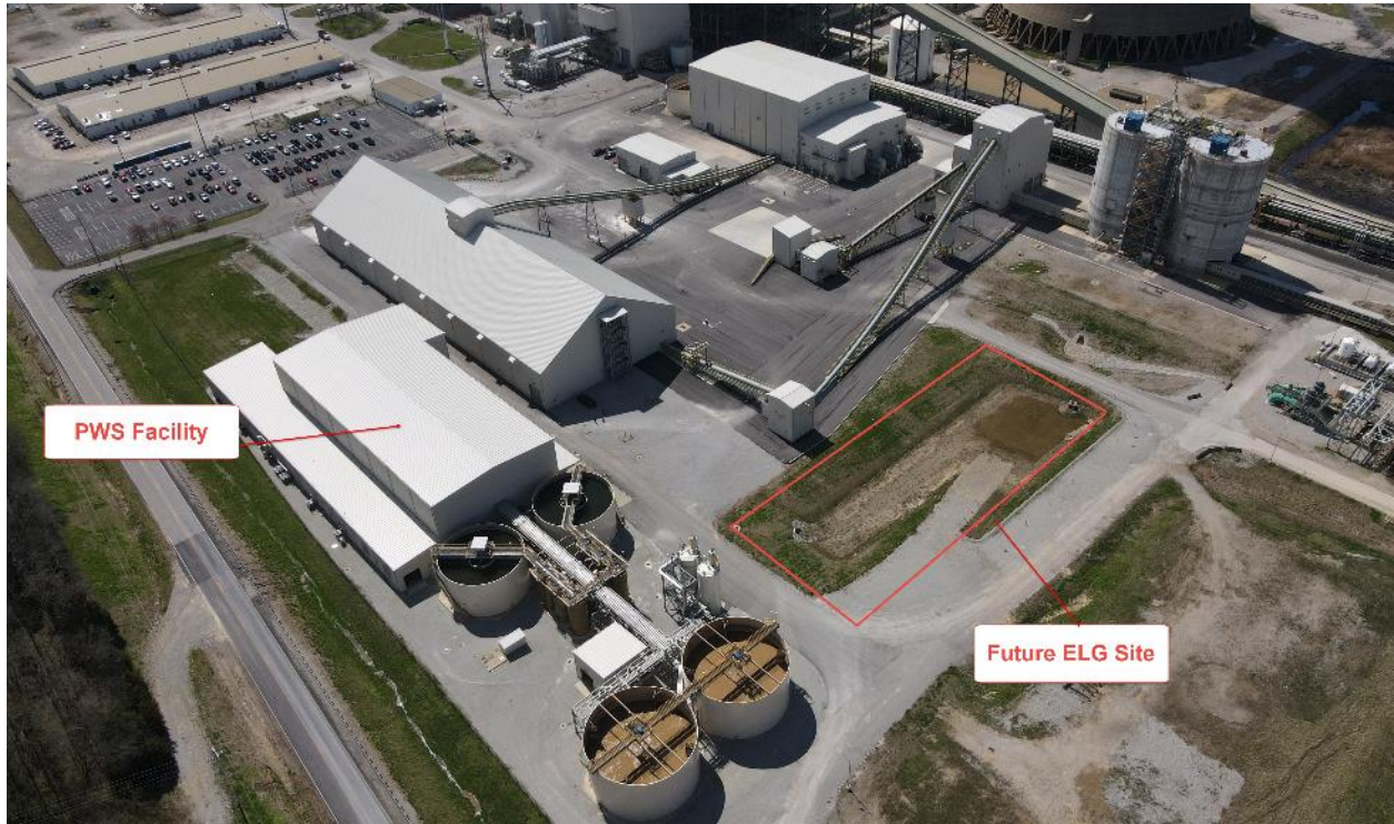
Trimble County – ELG Water Treatment Future Location – March 2021
