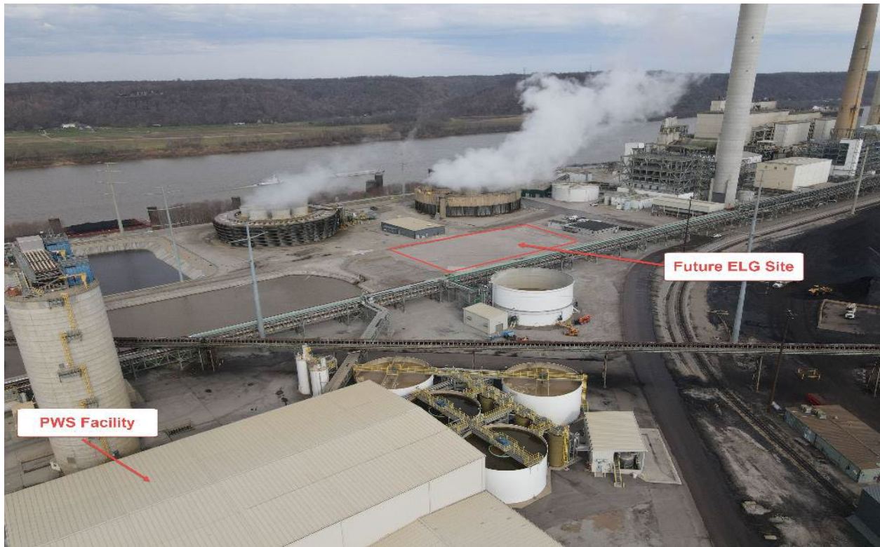
Mill Creek – ELG Water Treatment Future Location – March 2022
