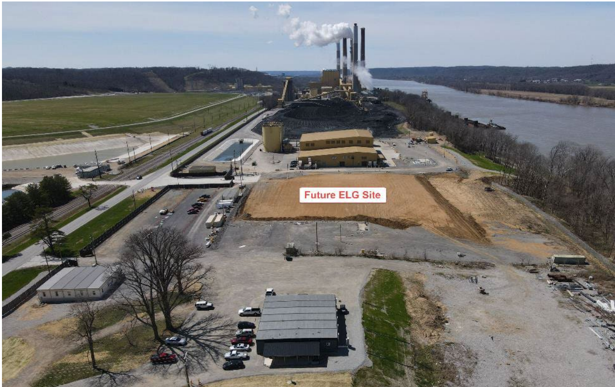
Ghent – ELG Water Treatment Future Location – March 2022
