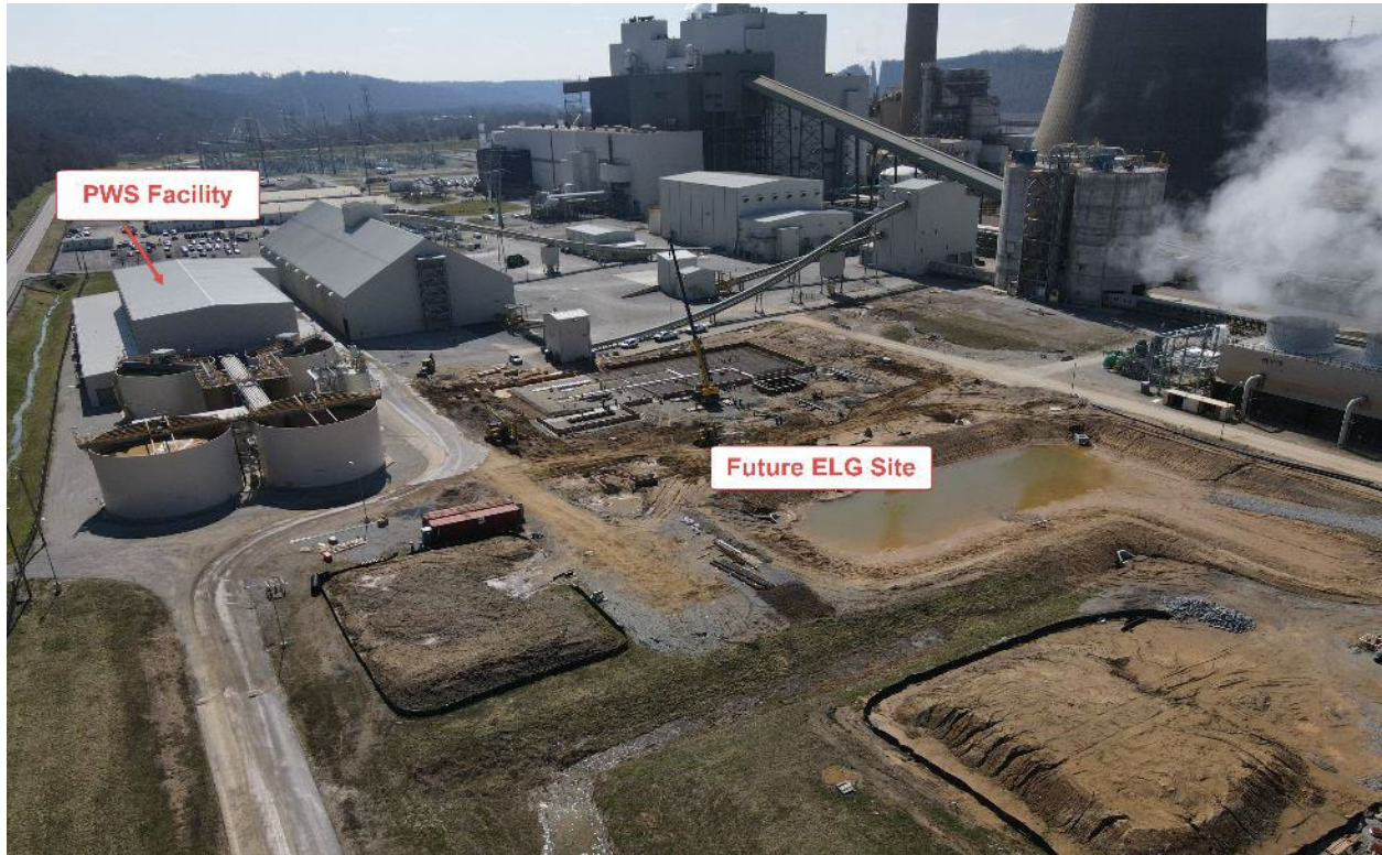
Trimble County – ELG Water Treatment Future Location – March 2022
