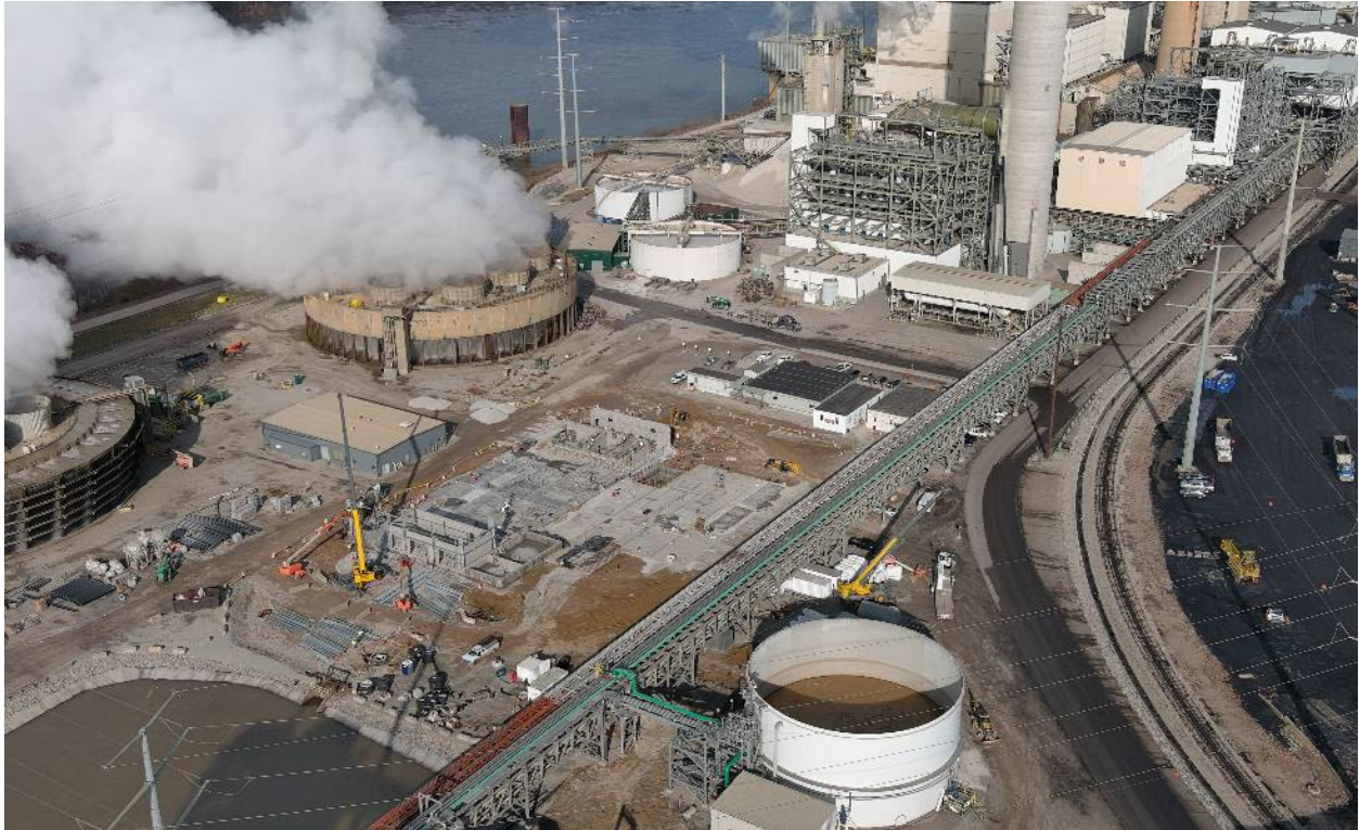
Mill Creek – ELG Water Treatment – December 2022
