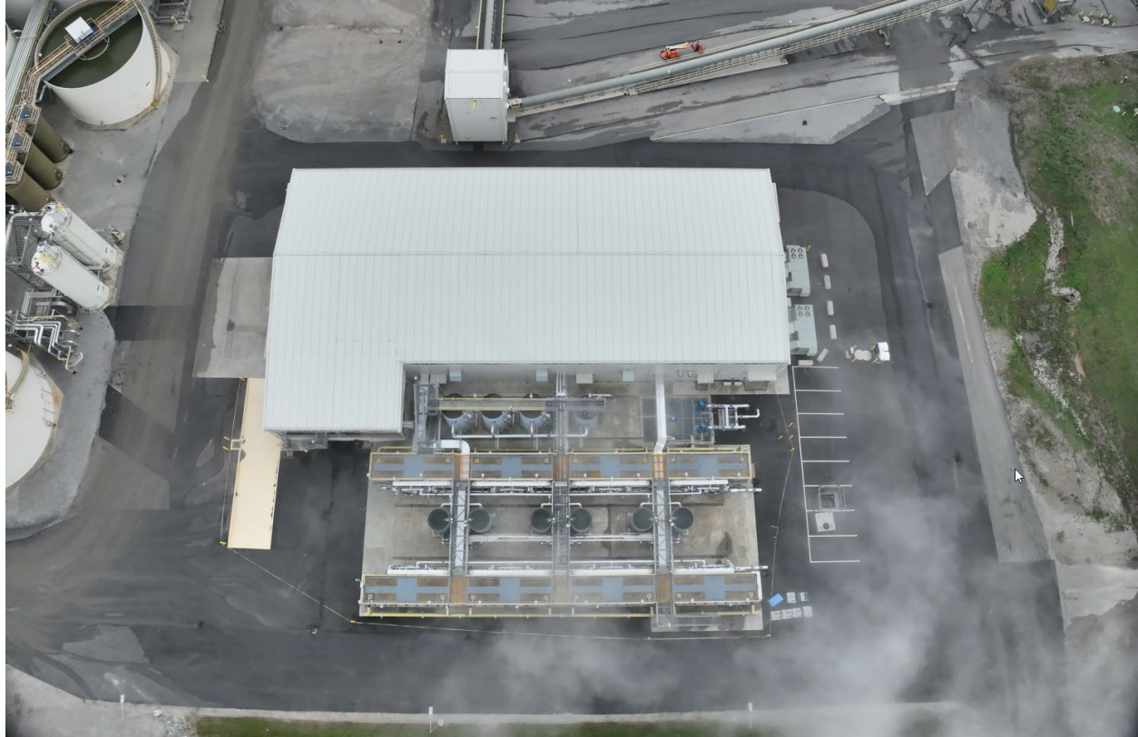
Trimble County – ELG Water Treatment Location – March 2024
