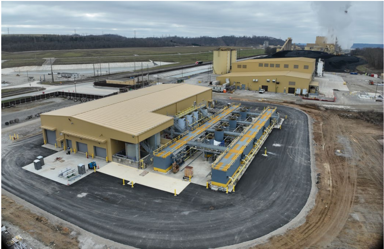
Ghent – ELG Water Treatment – December 2023
