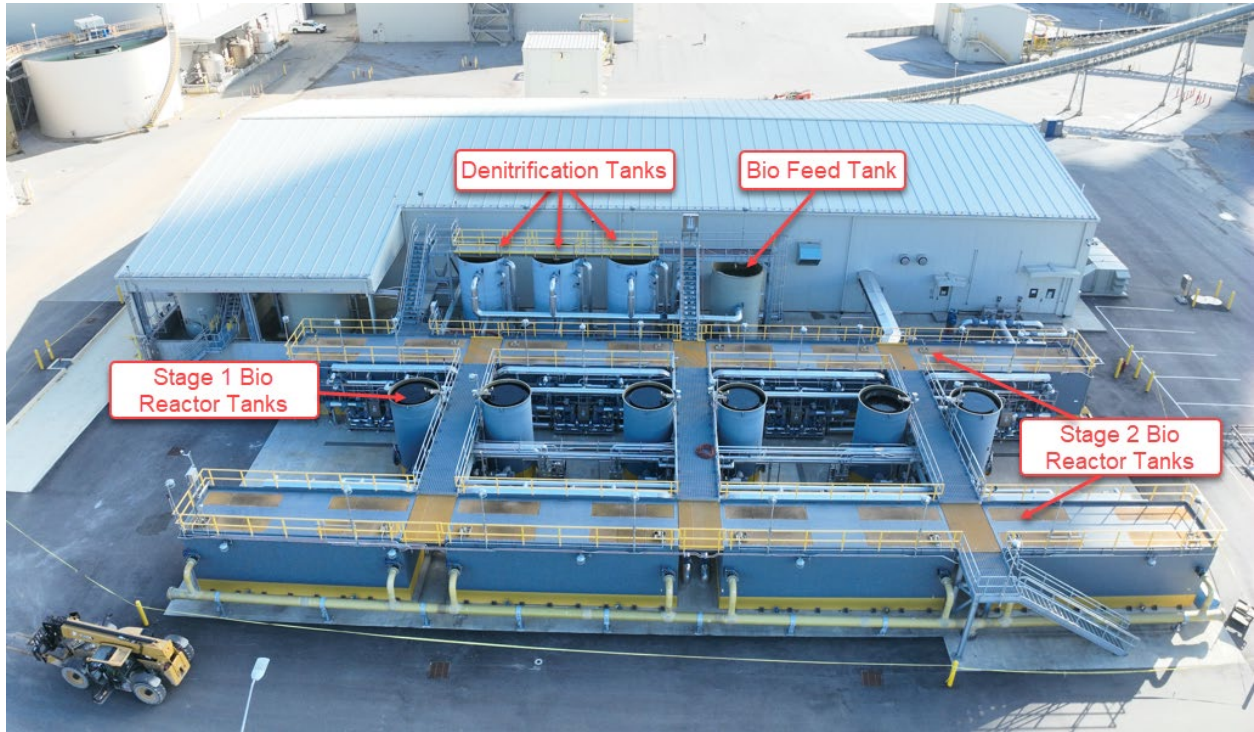
Trimble County – ELG Water Treatment Location – December 2023
