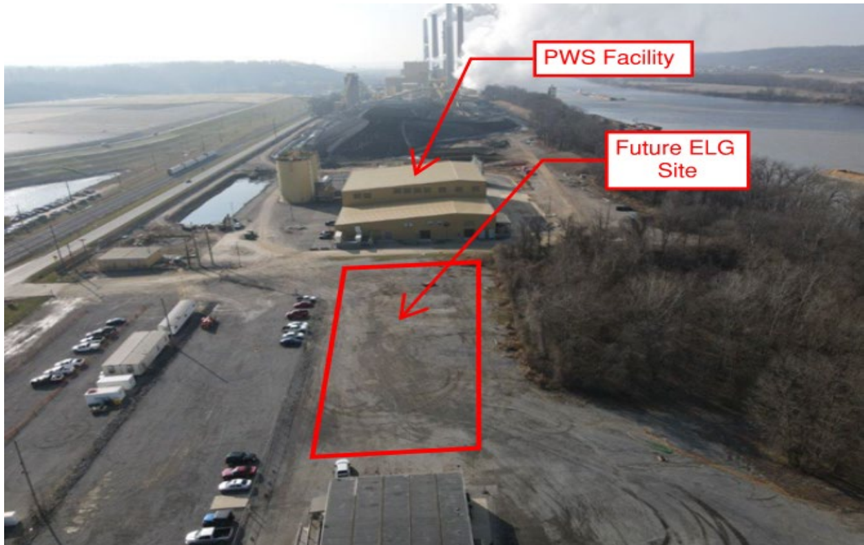
Ghent – ELG Water Treatment Future Location – December 2020
