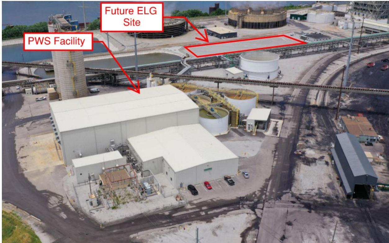
Mill Creek – ELG Water Treatment Future Location – December 2020
