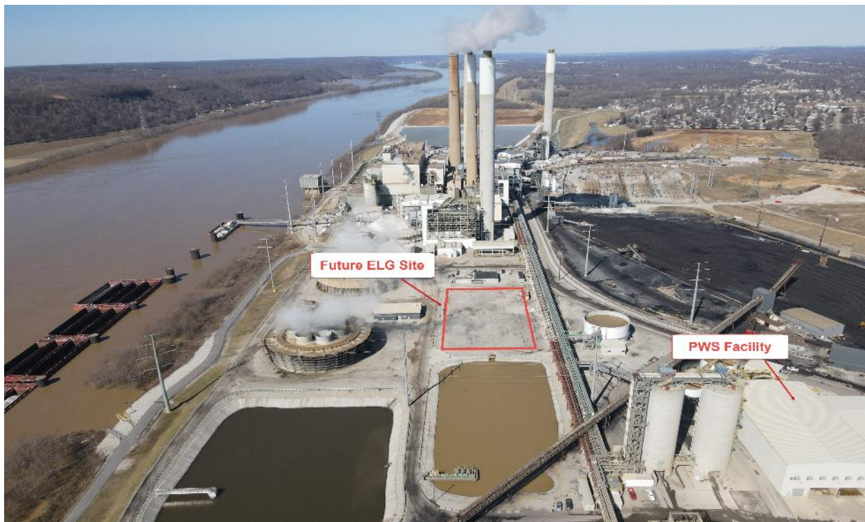
Mill Creek – ELG Water Treatment Future Location – March 2021
