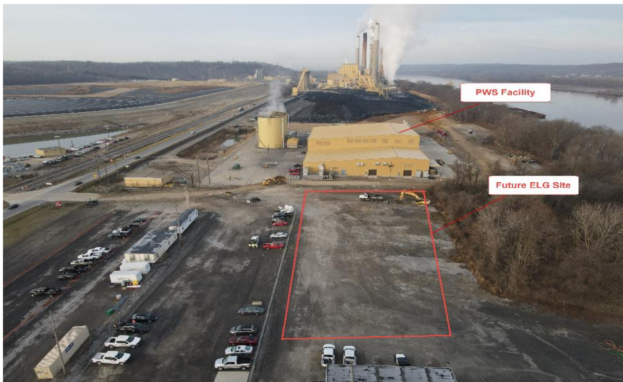
Ghent – ELG Water Treatment Future Location – March 2021
