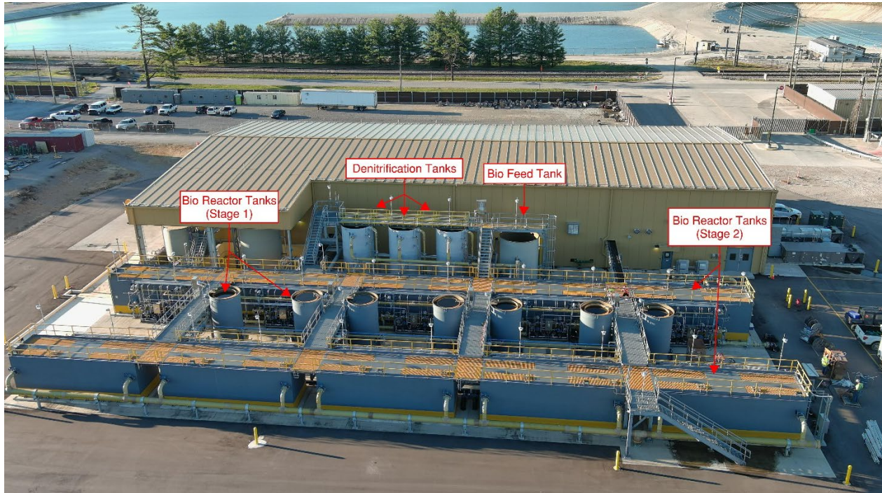
Ghent – ELG Water Treatment – No Changes
