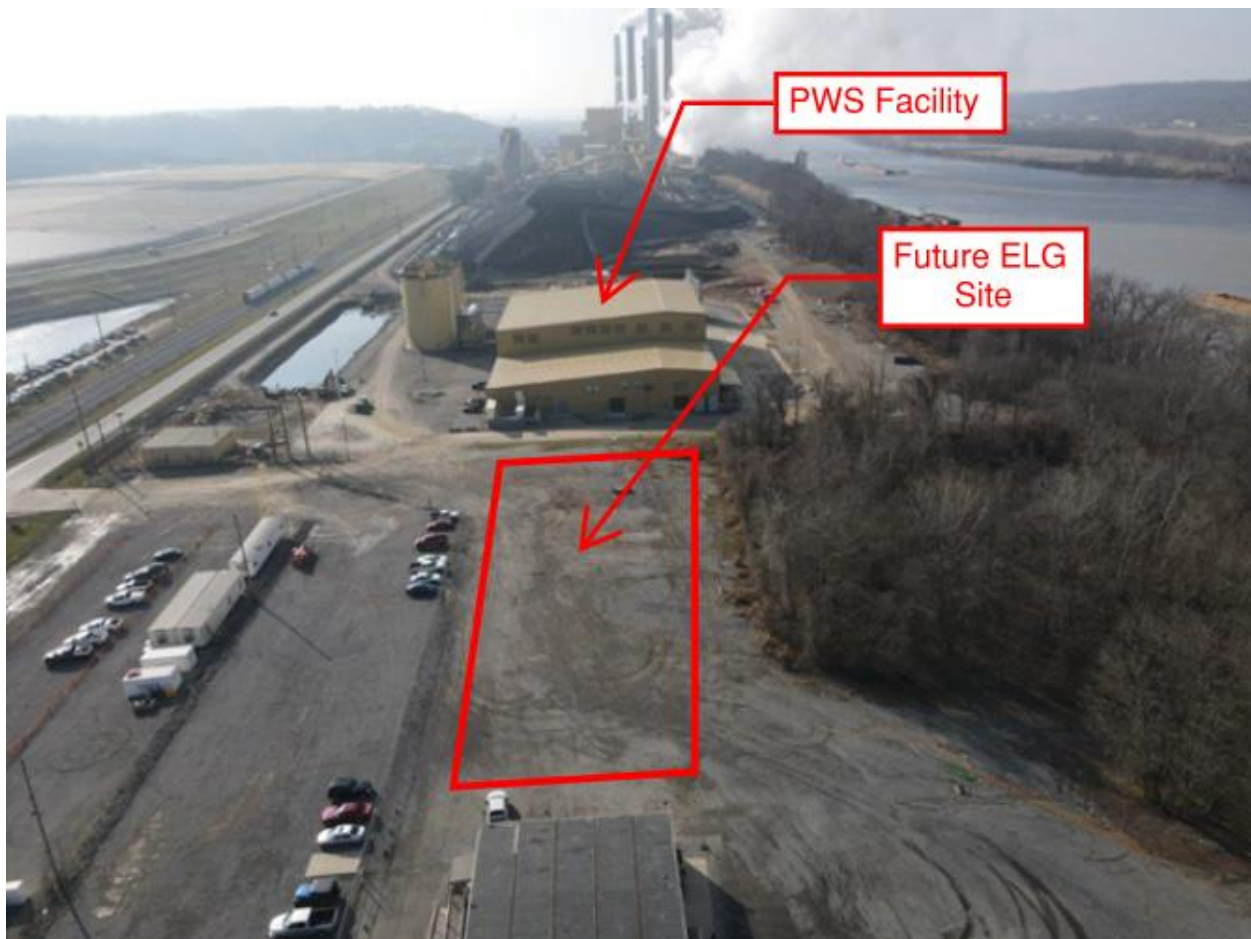
Ghent – ELG Water Treatment Future Location – December 2020
