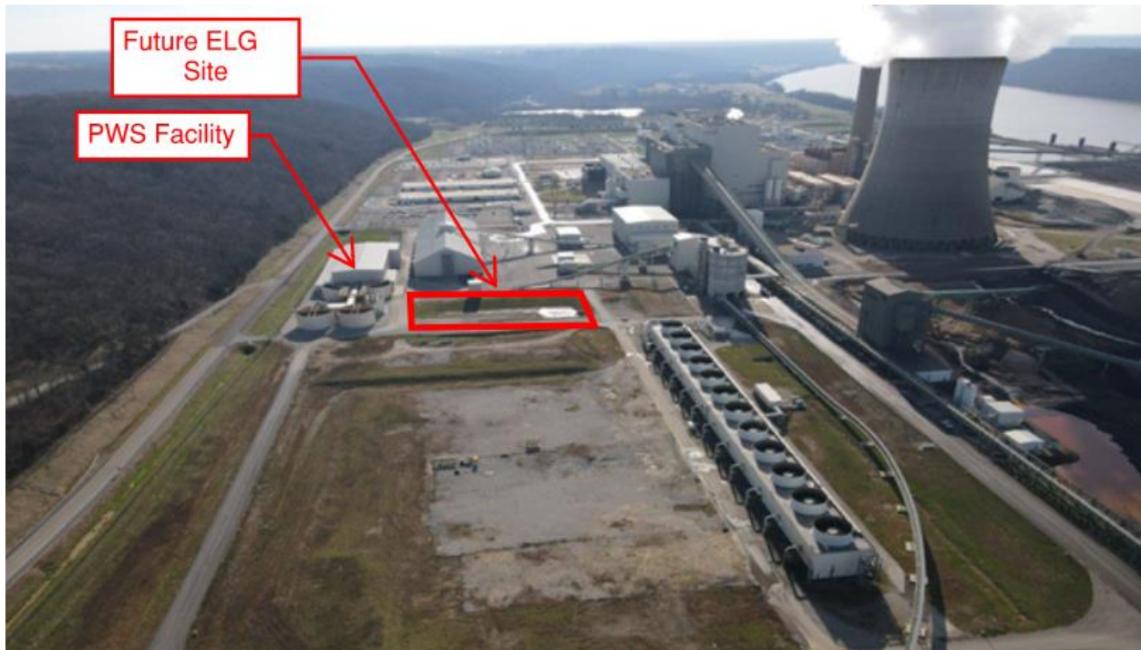
Trimble County – ELG Water Treatment Future Location – December 2020
