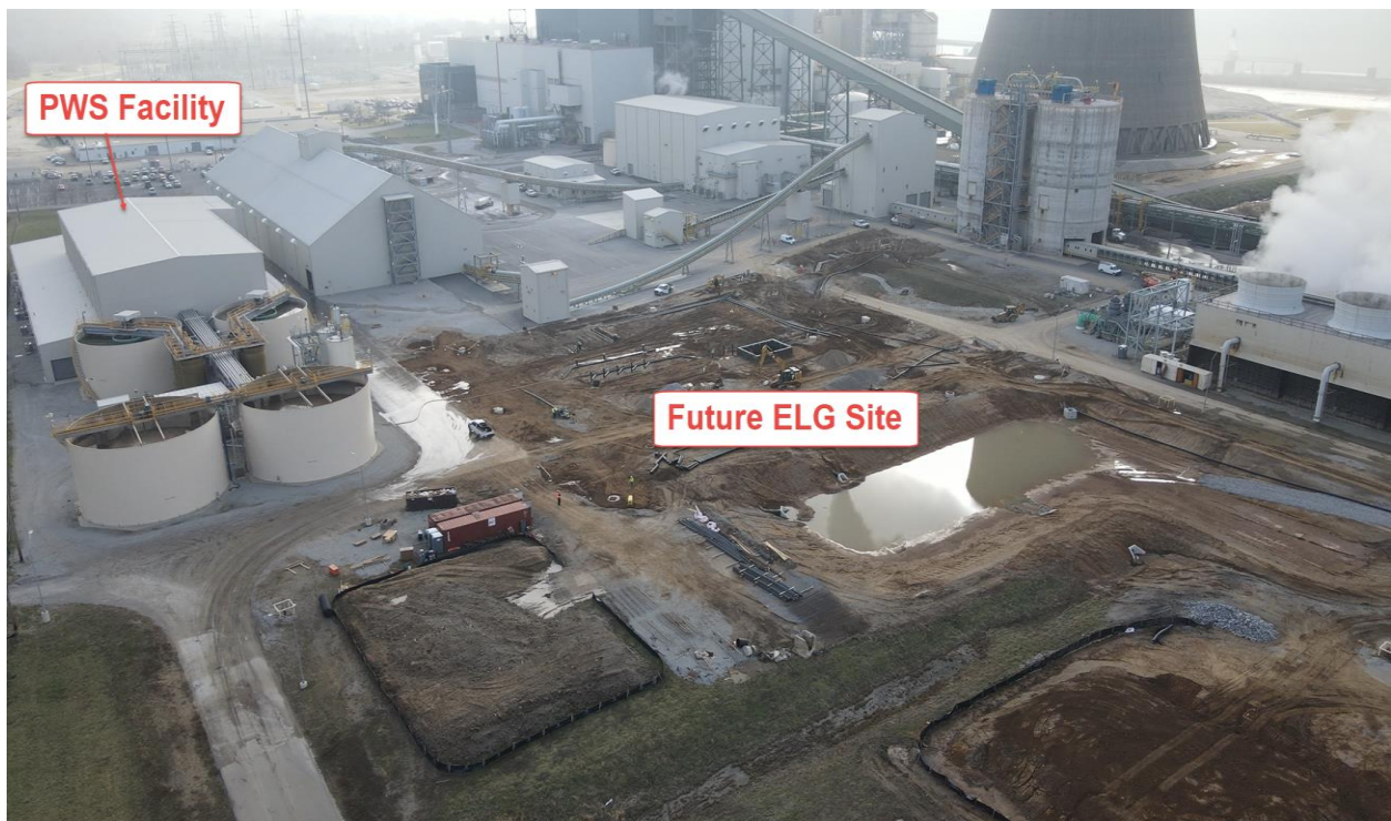
Trimble County – ELG Water Treatment Future Location – January 2022
