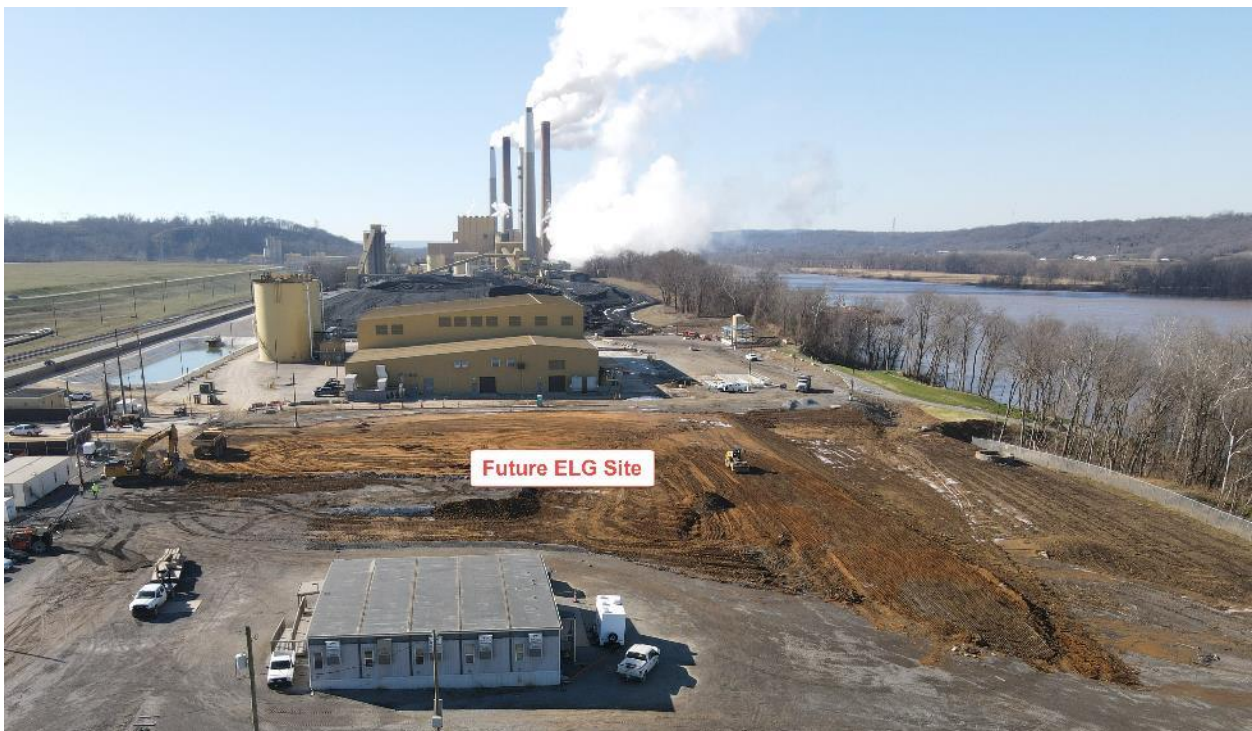
Ghent – ELG Water Treatment Future Location – January 2022
