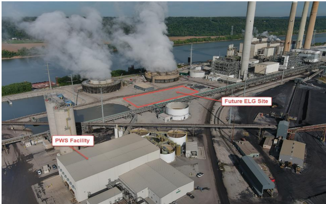
Mill Creek – ELG Water Treatment Future Location – October 2021
