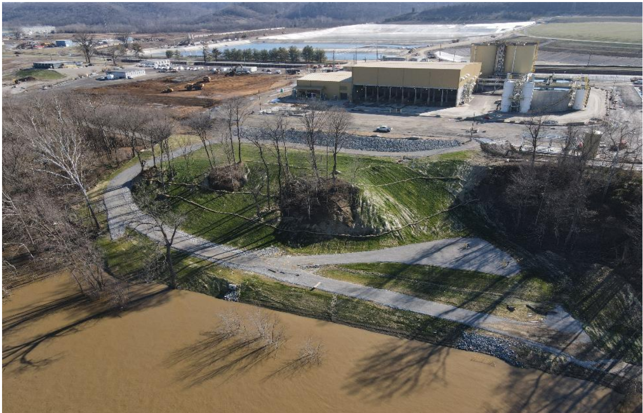
Ghent Outfall 001 Diffuser – Land Overview Looking Southeast – January 2022
