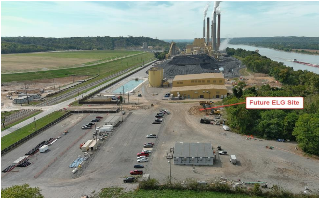
Ghent – ELG Water Treatment Future Location – September 2021
