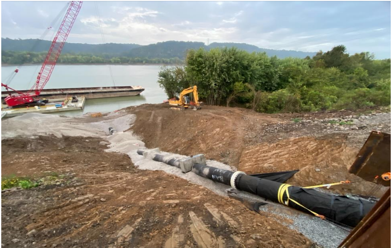
Mill Creek – North Diffuser – October 2021
