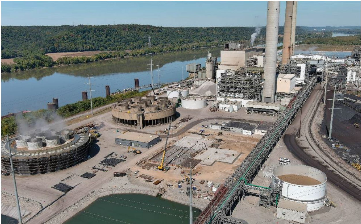
Mill Creek – ELG Water Treatment – October 2022
