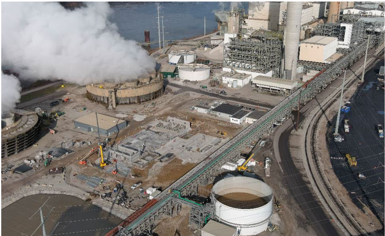
Mill Creek – ELG Water Treatment – December 2022
