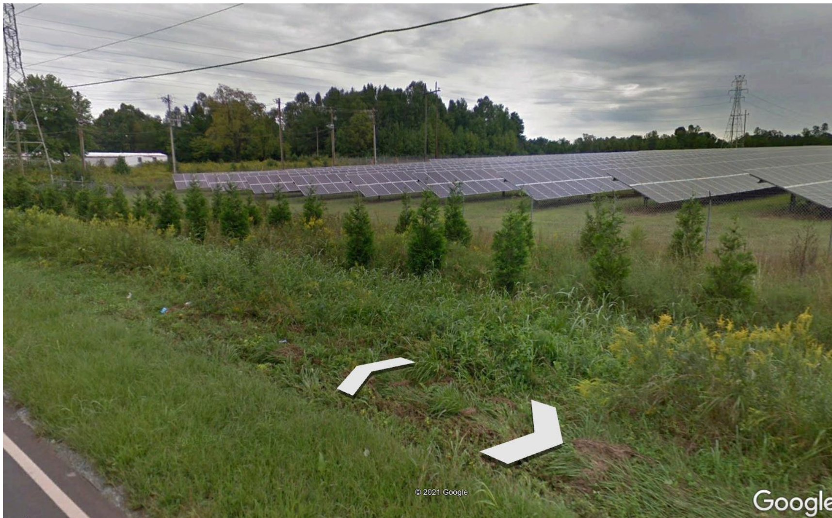
Image 4: Solar farm in Orange County, outside of Mebane, NC. Buffer shown is an alternating row of evergreen trees approximately 6-7ft tall. Image from Google Streetview.
