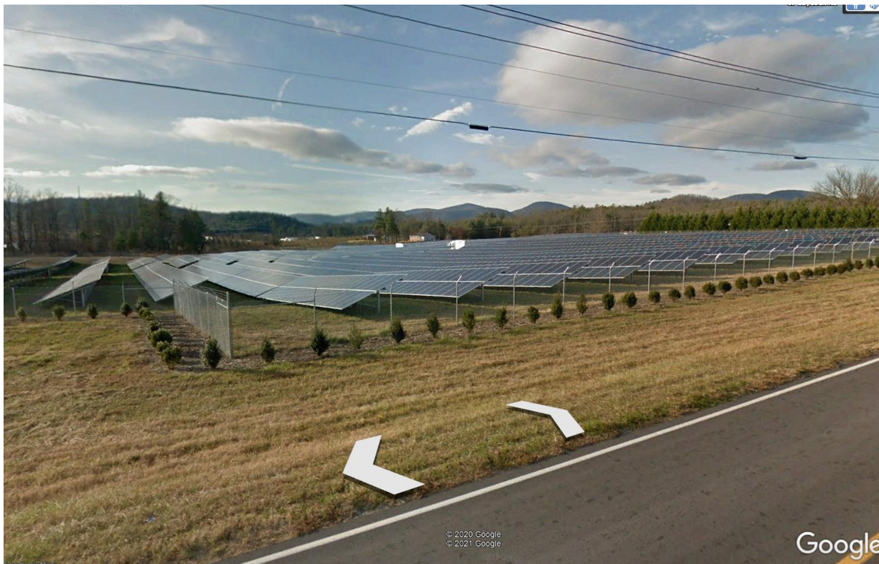
Image 1: A solar farm in Western NC. Buffer shown in a single row of 3-4ft tall evergreen trees. Image from Google Streetview.
