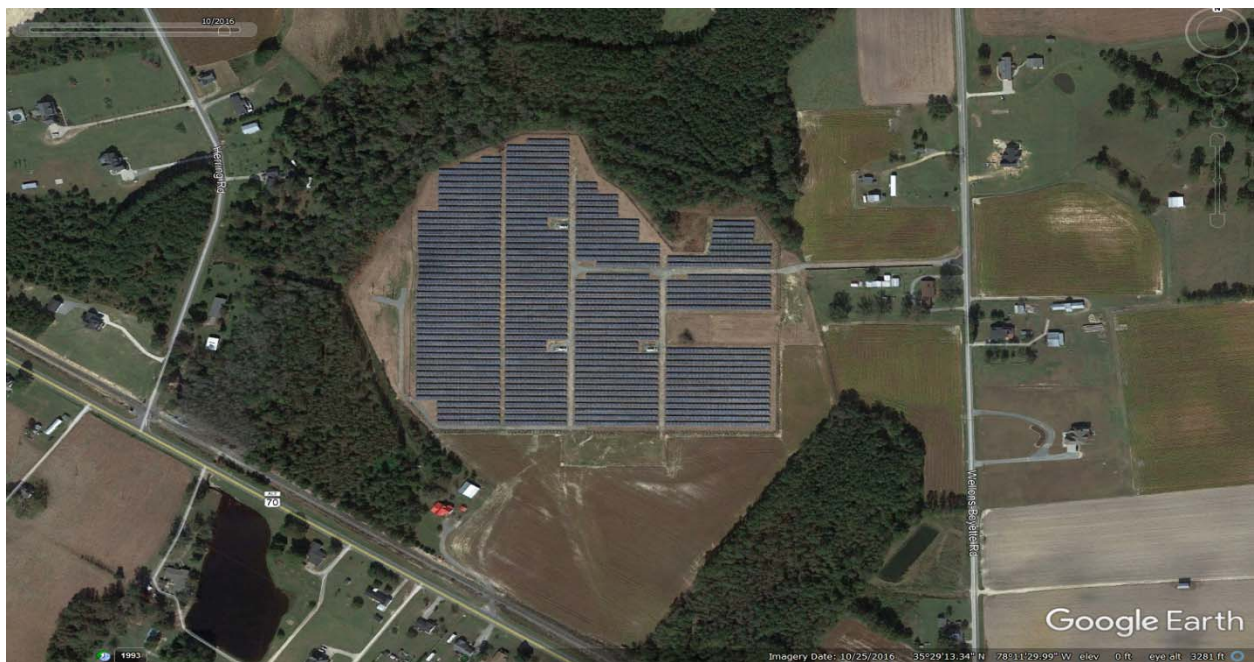
This solar farm is located at 4839 US 70 Highway just east of Herring Road. This solar farm was completed on October 25, 2016.
