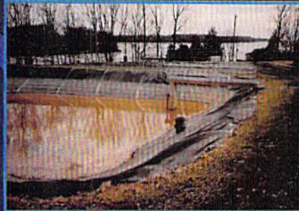
Residual Solids Storage
