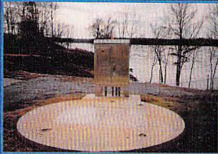
Residual Solids Pumping Station
