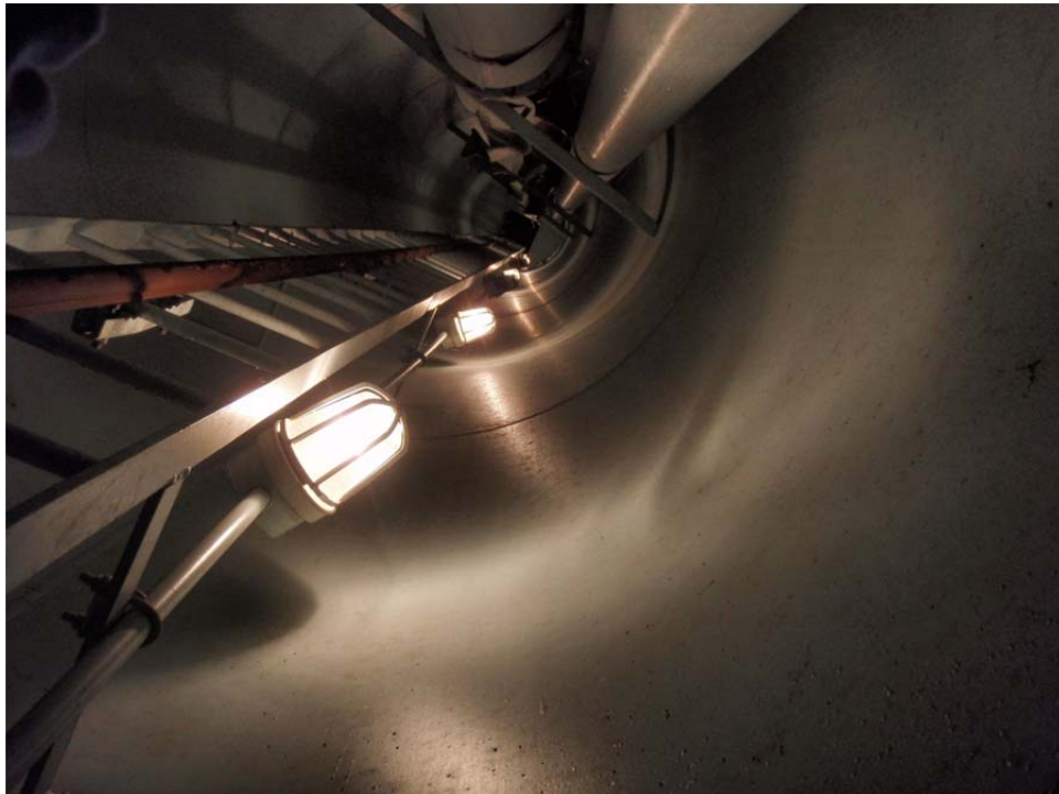
Photograph 8 – Rusted Safe-T-Climb Rail System on Interior Dry Riser (looking up)
