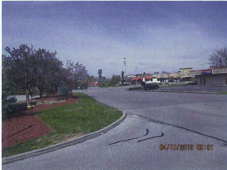
Photo Location 16. View of proposed route just north of Florence Mall and southwest of Woodspoint Station (Proposed). Photograph taken facing west.
