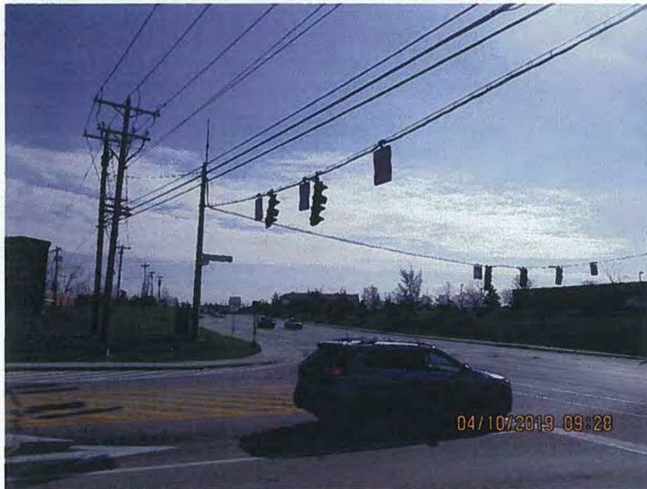
Photo Location 5. View of proposed route crossing at the intersection of Houston Road and Ted Bushelman Boulevard. Photograph taken facing northeast.
