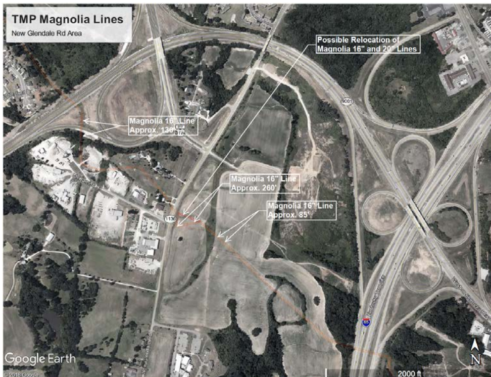
Photo 4: The photo depicts a crossing on the Magnolia 16-inch Line to be replaced under Old Mill Rd.
