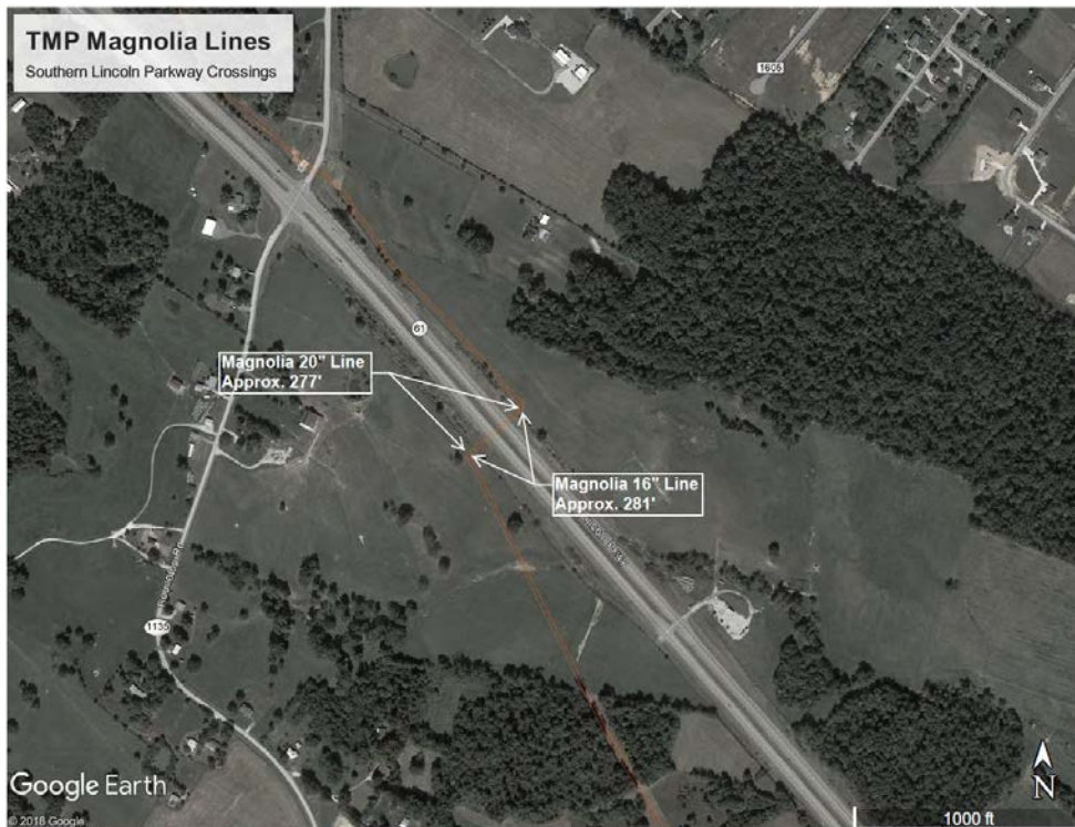
Photo 2: The photo depicts crossings on both Magnolia Lines to be replaced under Lincoln Pkwy, north of Harvest Dr
