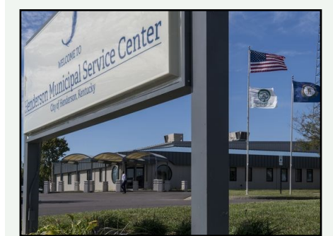
The new Municipal Service Center housing the Public Works Department, Henderson Municipal Gas utility and Special Projects Office has been in the works for many years.
