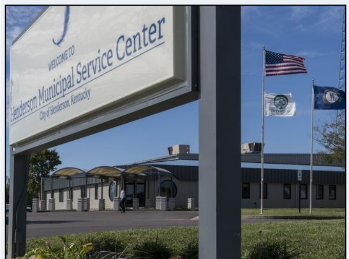
The Municipal Service Center housing the Public Works Department, Henderson Municipal Gas utility and Special Projects Office was in the works for many years and finally opened in 2017. A new gutter system and wash bay are the next planned improvements.
