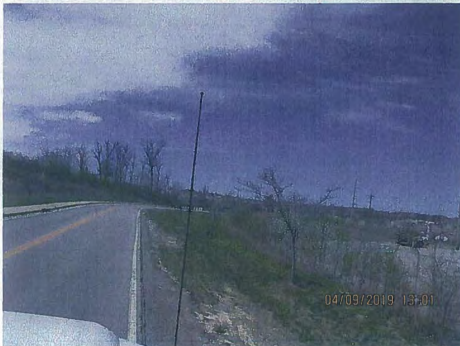
Photo Location 2. View of Oakbrook Drive north of Oakbrook Station. Photograph taken facing west.
