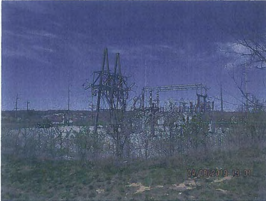
Photo Location 2. View of Oakbrook Station. Photograph taken facing northwest.
